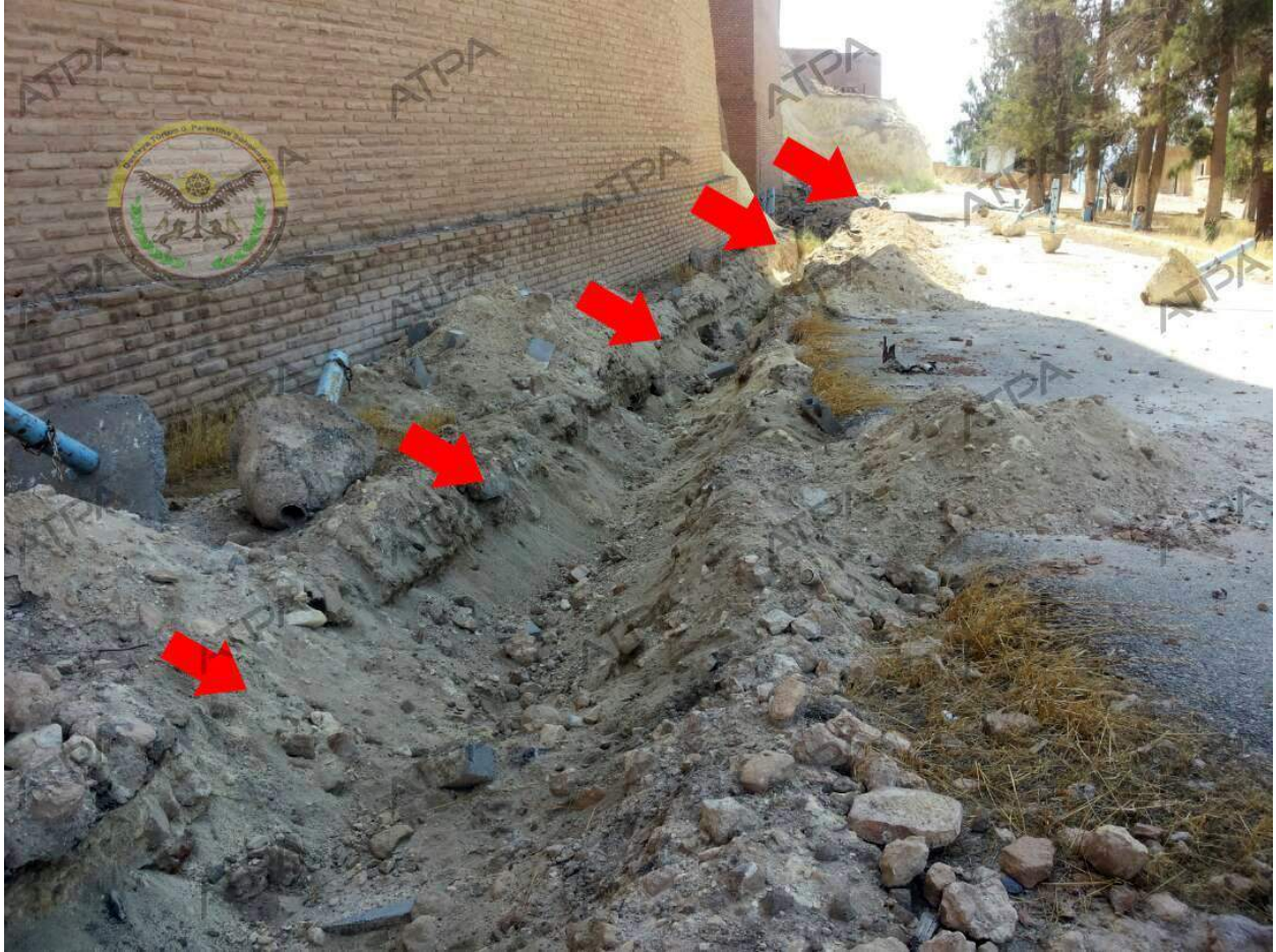
The trench where the cables were located (ATPA; September 23, 2017)
