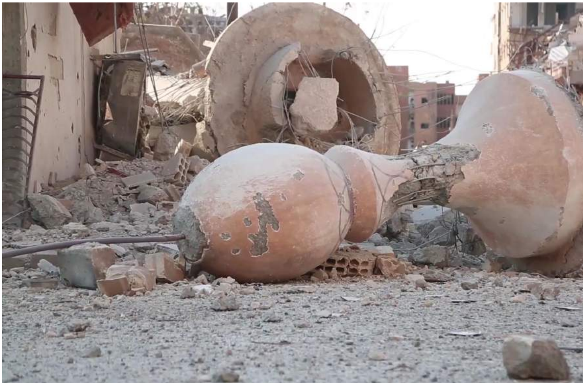
The remains of the top of the minaret (RBSS; September 18, 2017)
