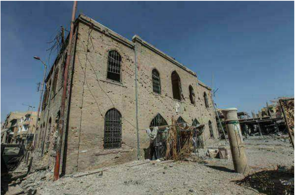
Damage to the southern facade (RBSS; September 15, 2017)
