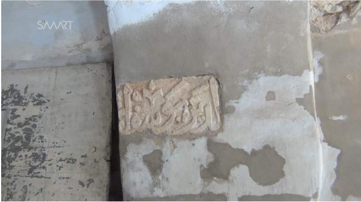
Video still of repairs to a wall (SMART News Agency; September 28, 2017)
