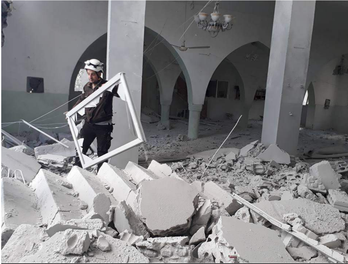
Damage to the interior of al-Kabir mosque (SNHR; September 26, 2017)
