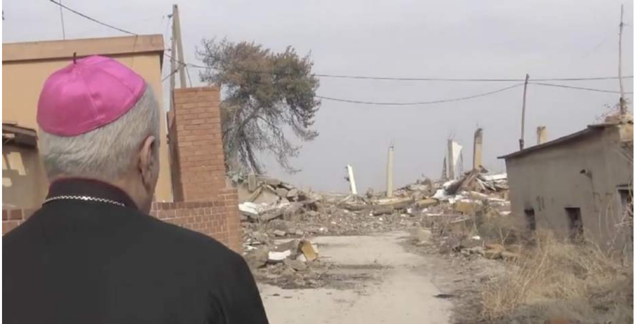
Video still of the rubble of the church (France 24; September 22, 2017)
