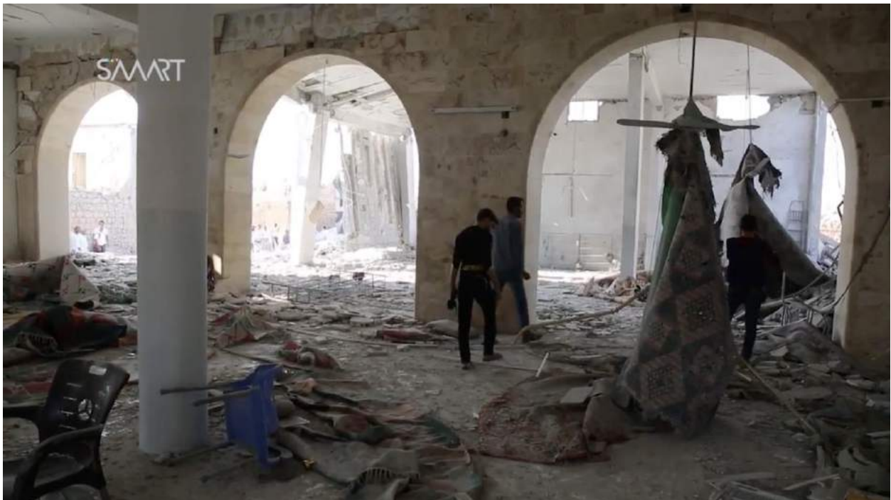
Video still of damage to the mosque's interior (SNHR; September 22, 2017)
