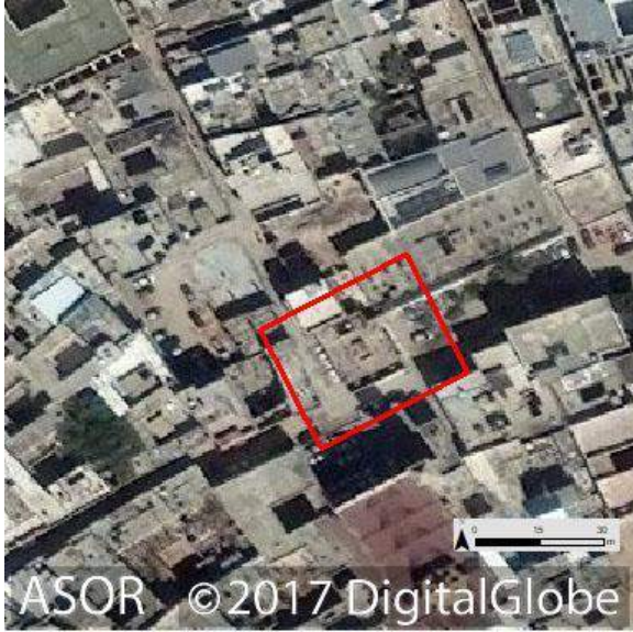
Historic building R-8 in the old city of Tripoli, shown within the red rectangle, prior to its destruction (DigitalGlobe NextView License; March 18, 2016)
