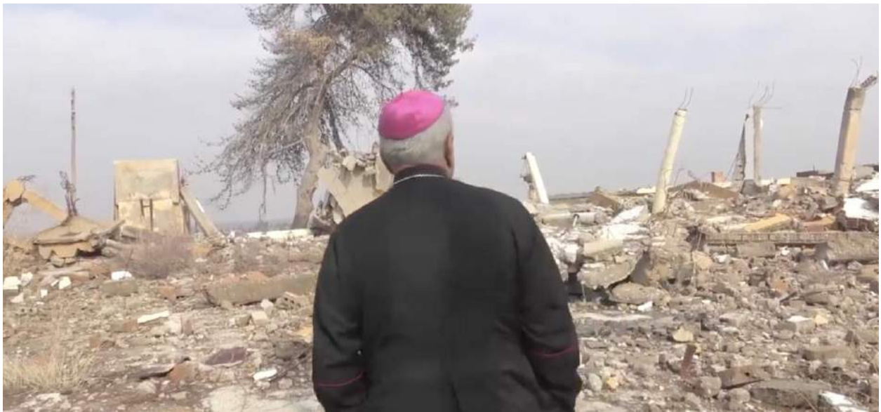
Video still of the rubble of the church (France 24; September 22, 2017)
