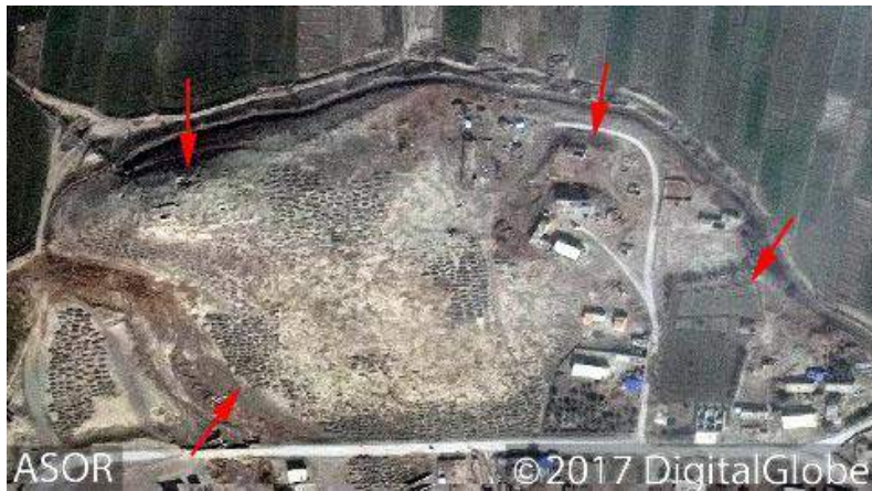
Tell Qsubi with multiple forms of damage indicated by red arrows (DigitalGlobe NextView License; February 17, 2017)
