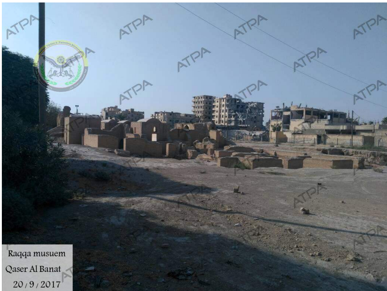
Qasr al-Banat, seen from the southeast (ATPA; September 23, 2017)
