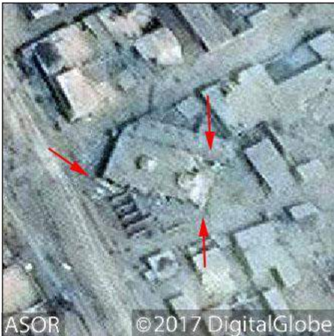
Damage to the mosque from explosives as indicated by the red arrows (DigitalGlobe NextView License; September 16, 2017)
