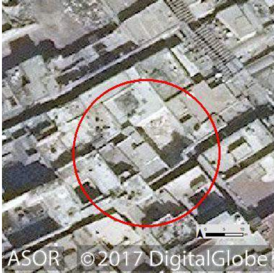
Historic building R-2 prior to destruction shown within the red circle (DigitalGlobe NextView License; October 19, 2016)
