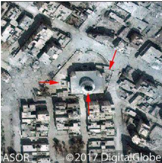
Severe damage to the dome of the mosque as a result of an airstrike indicated by red arrow. Additionally damage also indicated by red arrows (DigitalGlobe NextView License; September 24, 2017)
