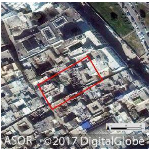
Construction of a new building in the place of R-11, shown within the red rectangle (DigitalGlobe NextView License; December 3, 2015)
