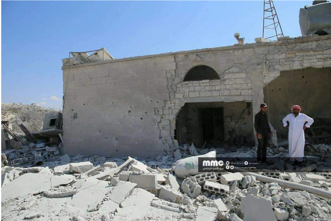
Damage to al-Janoubi Mosque (SNHR; September 28, 2017)
