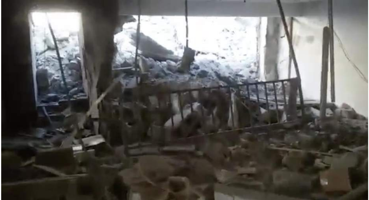
Video still of damage to the mosque (SNHR; September 29, 2017)
