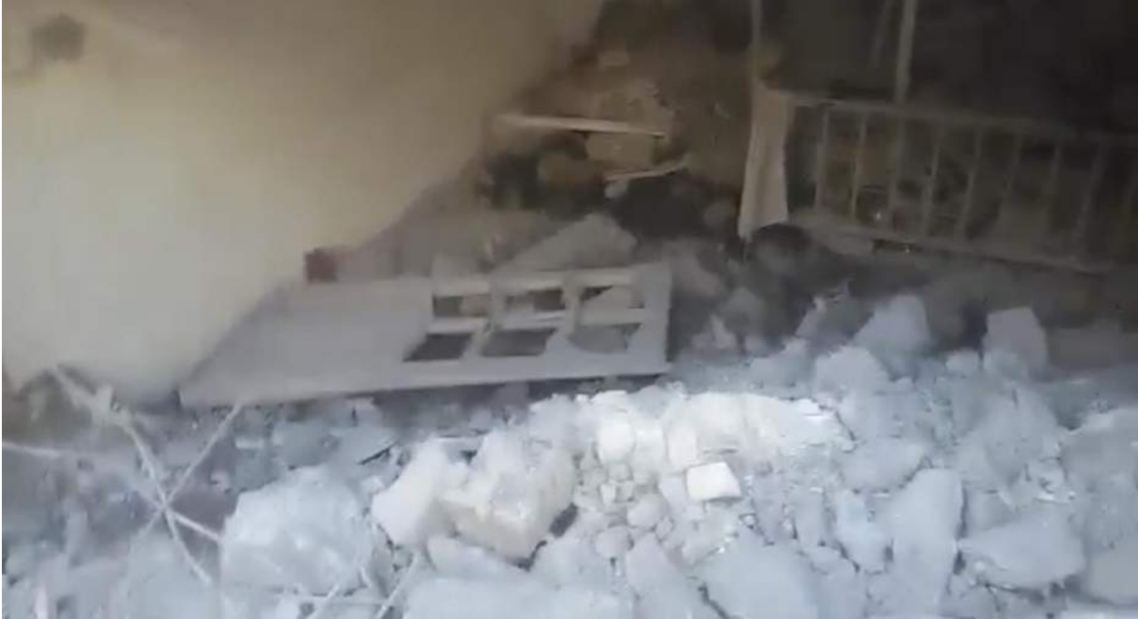
Video still of damage to the mosque, seen from the outside (SNHR; September 29, 2017)
