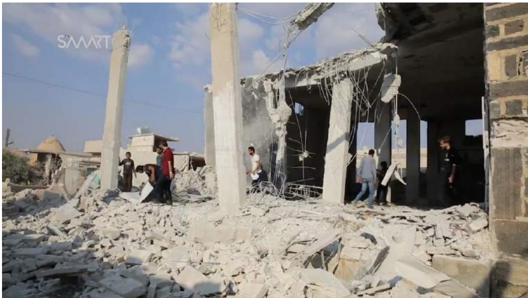
Video still of damage to the mosque (SNHR; September 22, 2017)
