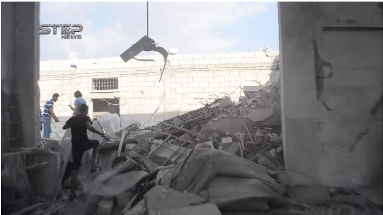
Video still of damage to the mosque (SNHR; September 22, 2017)
