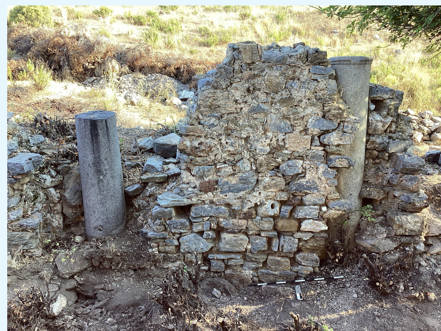
Northern wall of building showing encased columns from earlier structure
