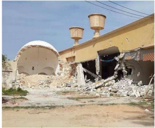
Destruction of the Sidi Bu Ghara Shrine in Tripoli, 2017 (Photo: Youssef al Khatali)
