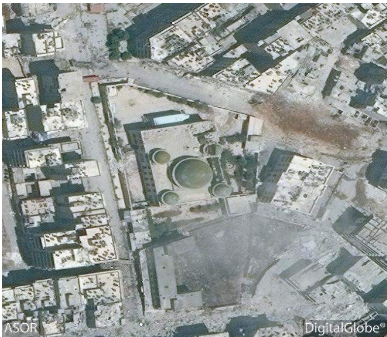
Salah ad Din Mosque seen with new damage to the western exterior wall. The minaret and dome on the northeastern corner were previously damaged in 2013 (DigitalGlobe; May 24, 2016).
