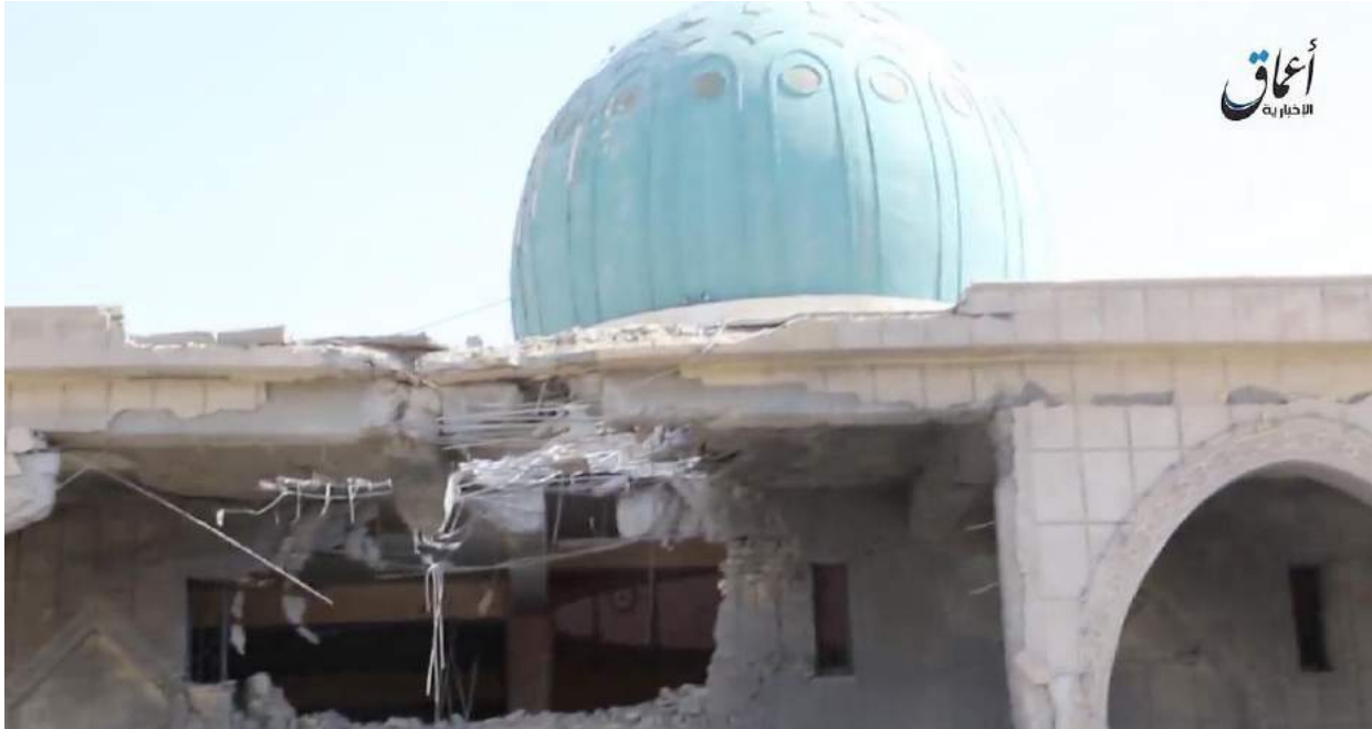
Detail of damage to Al Raqib Mosque (Amaq News Agency; May 23, 2016)
