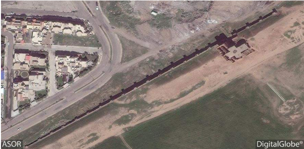
Adad Gate and city wall prior to destruction (ASOR CHI/DigitalGlobe; April 1, 2016)
