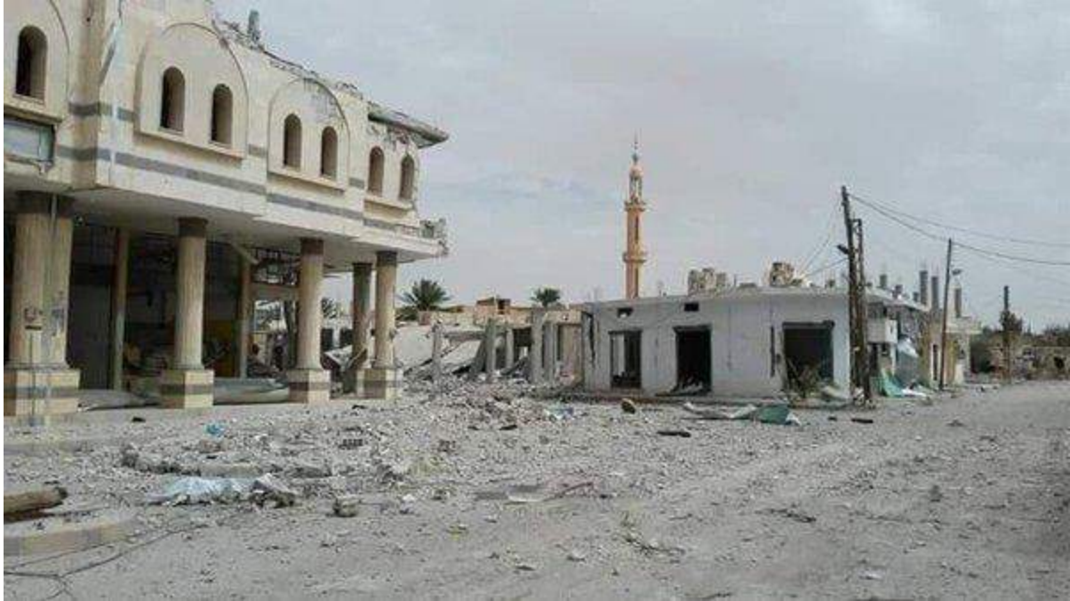
Damage around Al Kabir Mosque (Palmyra Coordination Committee; May 15, 2016)
