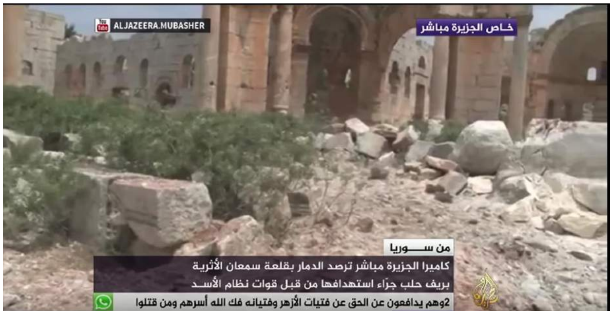
Damage to central courtyard and fallen pillar (facing northeast) (Al Jazeera Mubasher; May 16, 2016)
