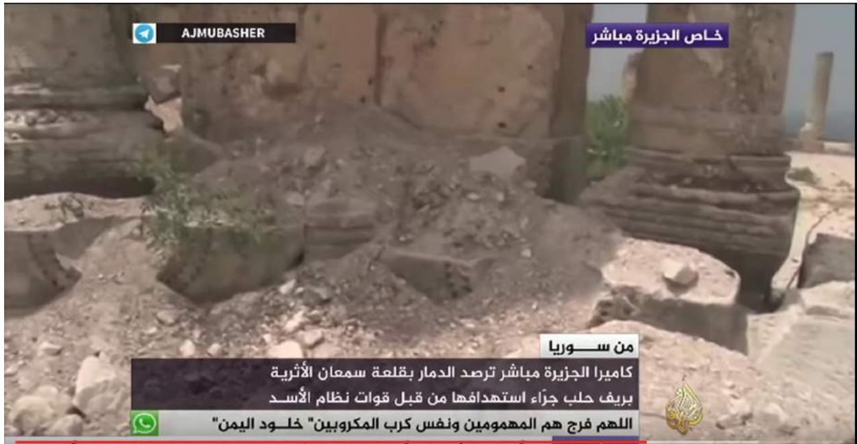
Damage and rubble in central courtyard (facing west) (Al Jazeera Mubasher; May 16, 2016)
