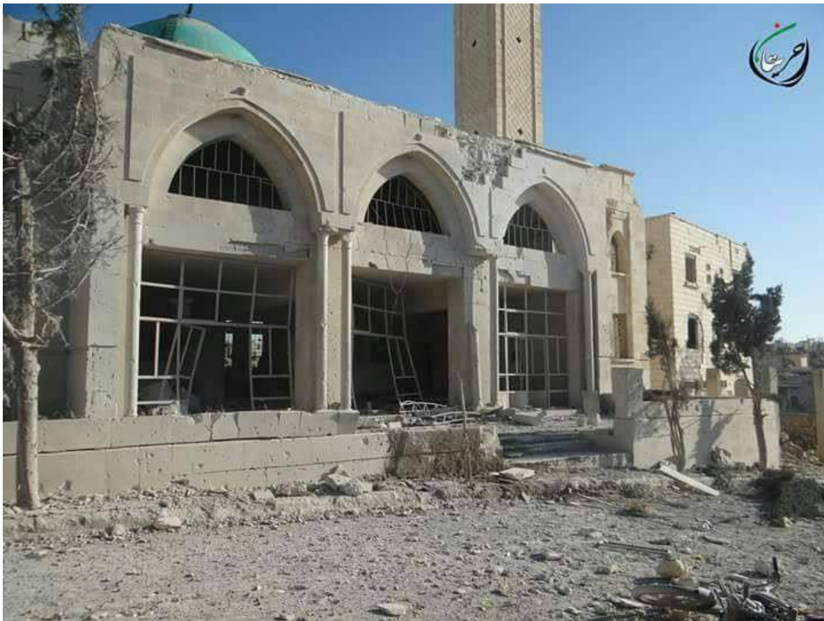
Damage to Al Bara bin Malek Mosque (SNHR; May 20, 2016)
