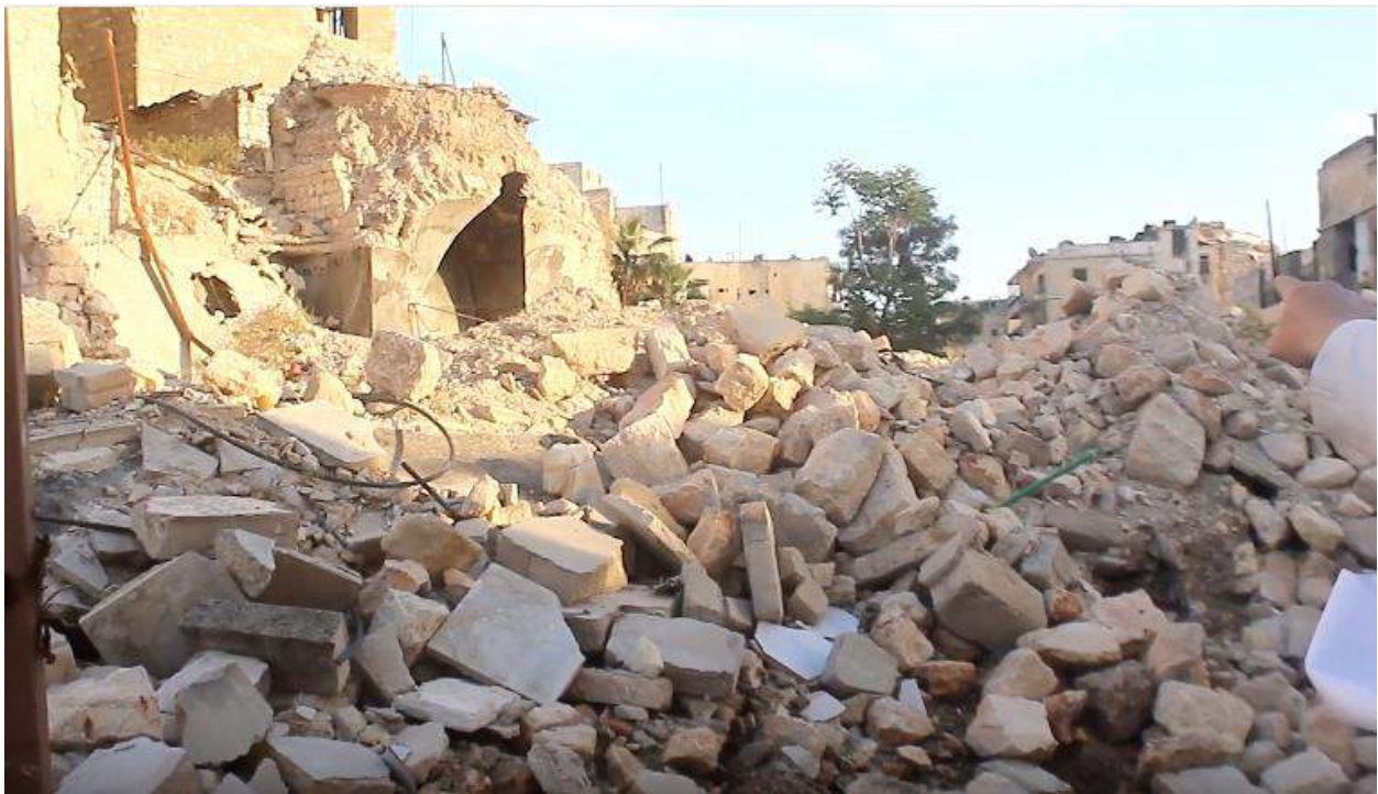
Damage to the Haddadin Mosque (Ahmed Melham; May 19, 2016)
