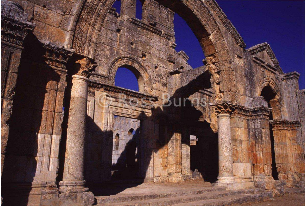
Pre-damage photo of central and eastern narthex arches (Ross Burns; December 24, 2013)
