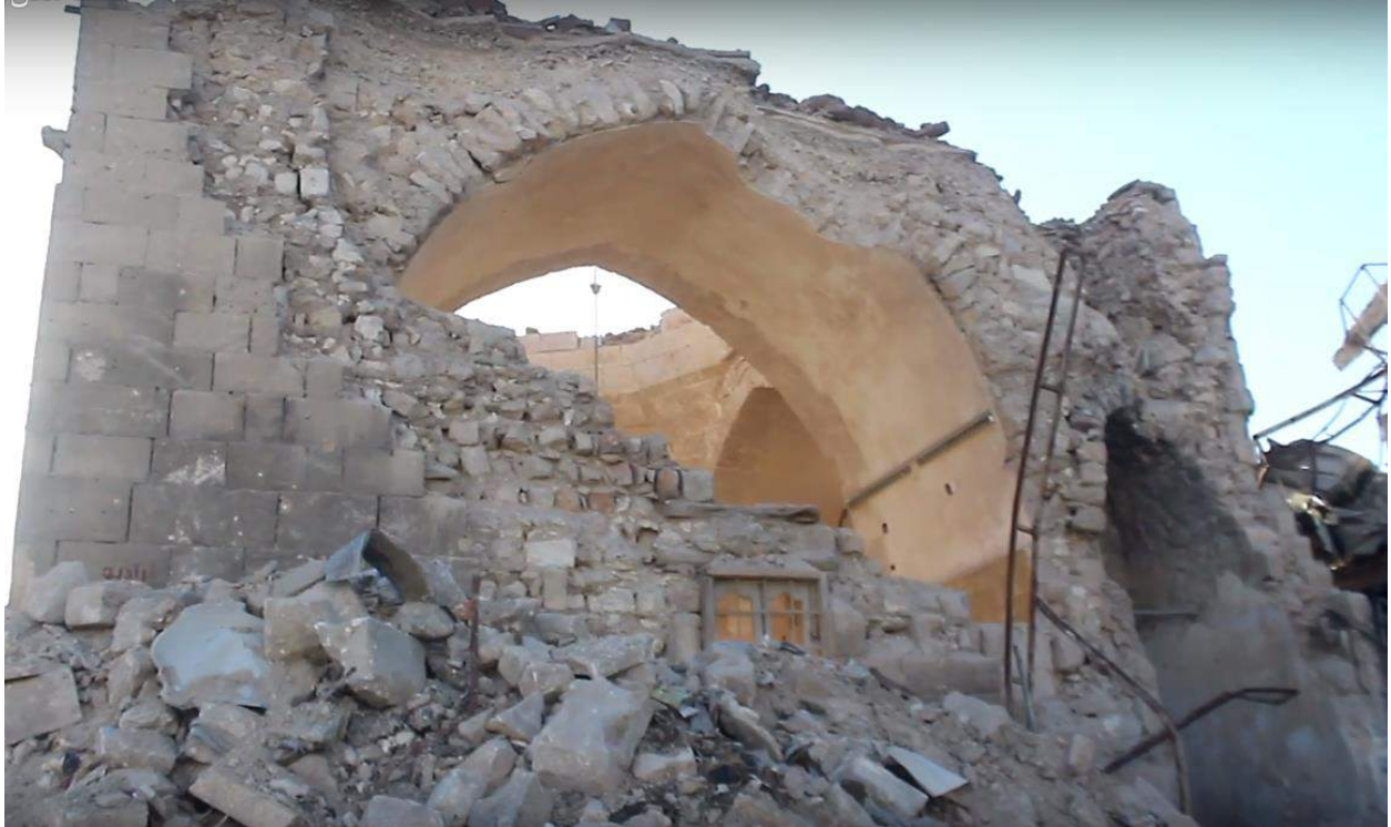
Video still of damage to an unidentified mosque (Ahmed Melham; May 19, 2016)
