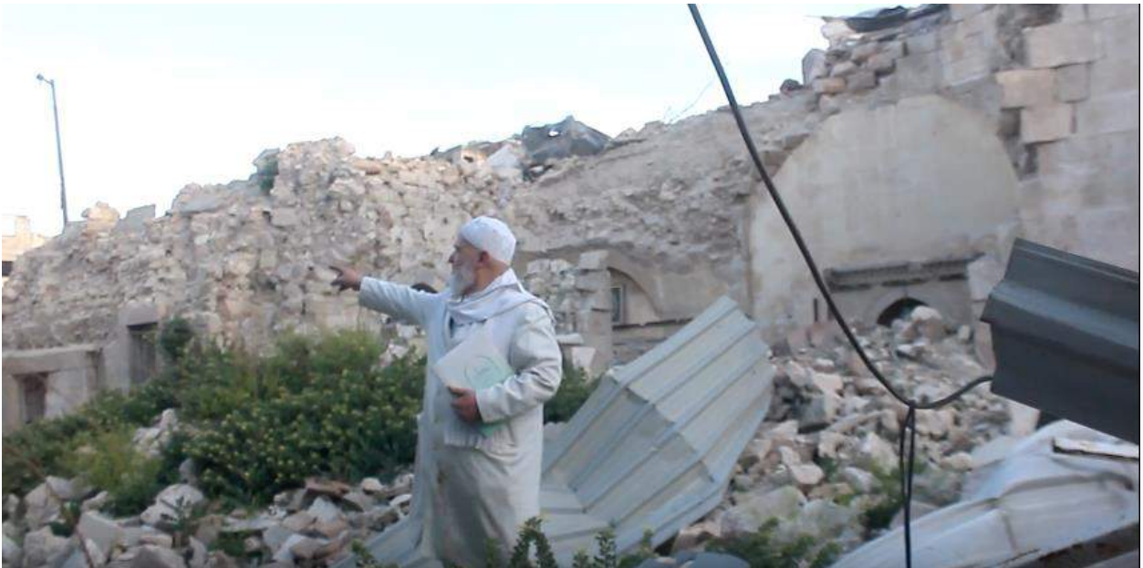
Video still of severe damage to Al Midani Mosque (Ahmed Melham; May 19, 2016)
