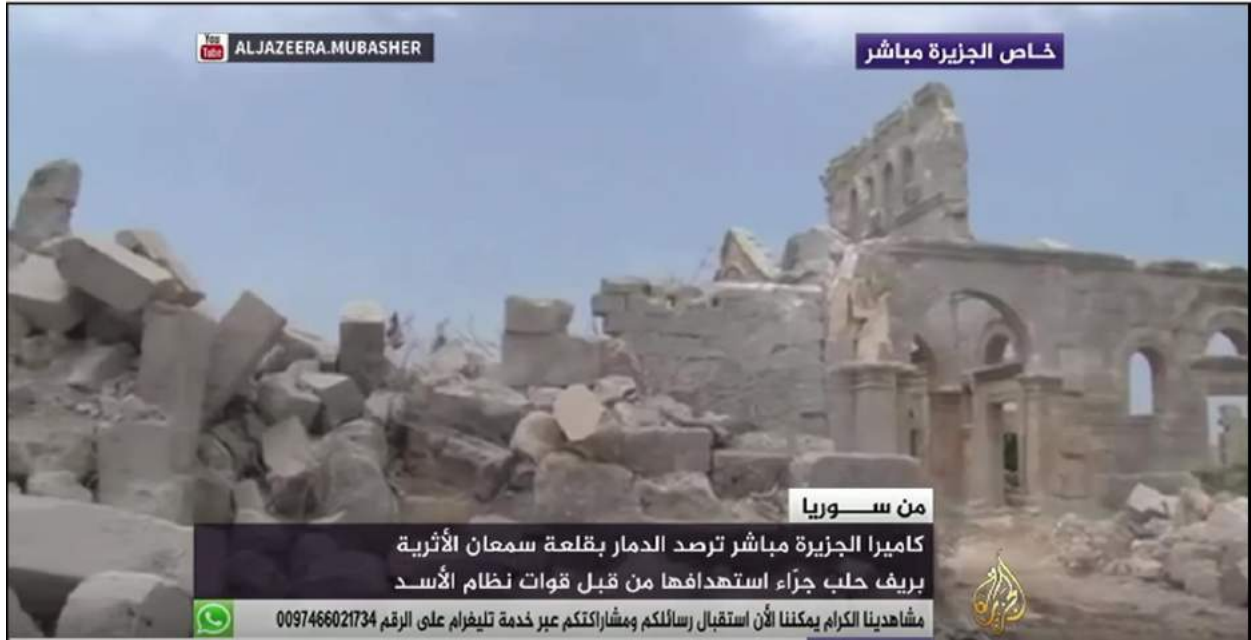
Destruction of western wall of monastery (facing west) (Al Jazeera Mubasher; May 16, 2016)
