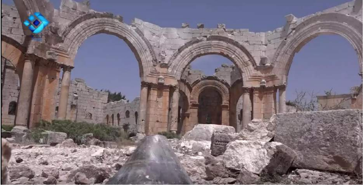
Damage to central courtyard with missile (facing north) (Wikalat Thiqa; May 13, 2016)
