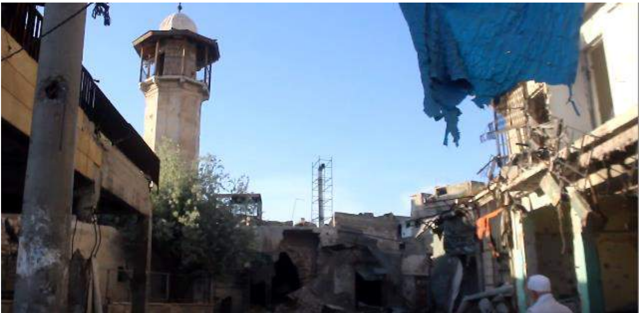
Video still of damage to an unidentified mosque (Ahmed Melham; May 19, 2016)
