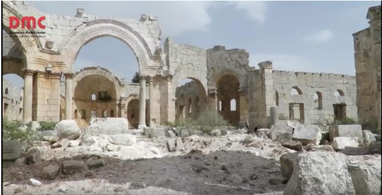
Damage to central courtyard of basilica with fallen pillar in middle left field (facing east) (Daretezza Media Center; May 15, 2016)
