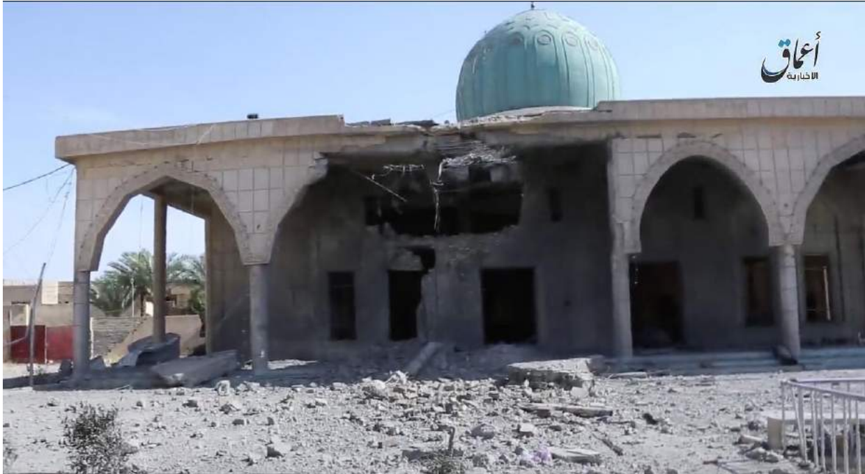
Damage to Al Raqib Mosque (Amaq News Agency; May 23, 2016)
