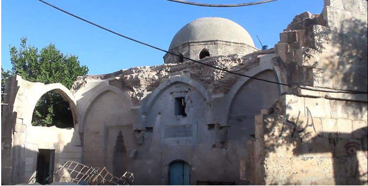
Video still of damage to Agha Jaq Mosque (Ahmed Melham; May 19, 2016)
