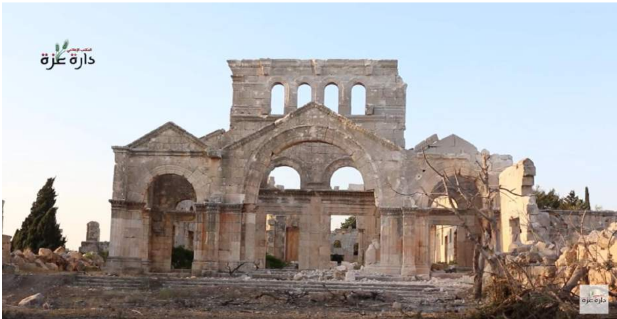
View of damage to facade of main entrance to Church of St. Simeon (looking north) (Daretezza Media Office; May 14, 2016)
