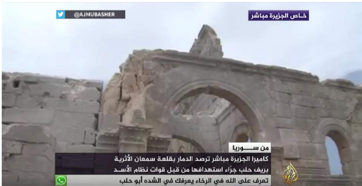
Damage to eastern exterior corner of narthex (Al Jazeera Mubasher; May 16, 2016)
