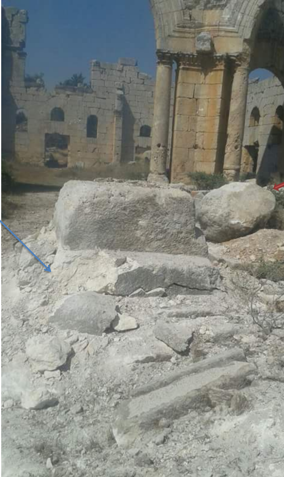
The pedestal (badly damaged) with the remaining fragment of St. Simeon's pillar knocked over to the right.
