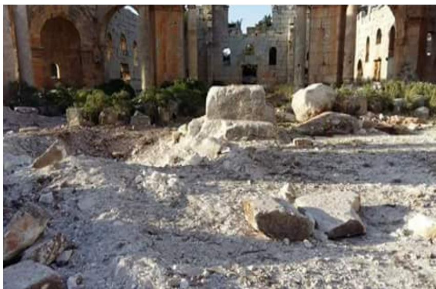
View of the damage caused by the airstrike .
