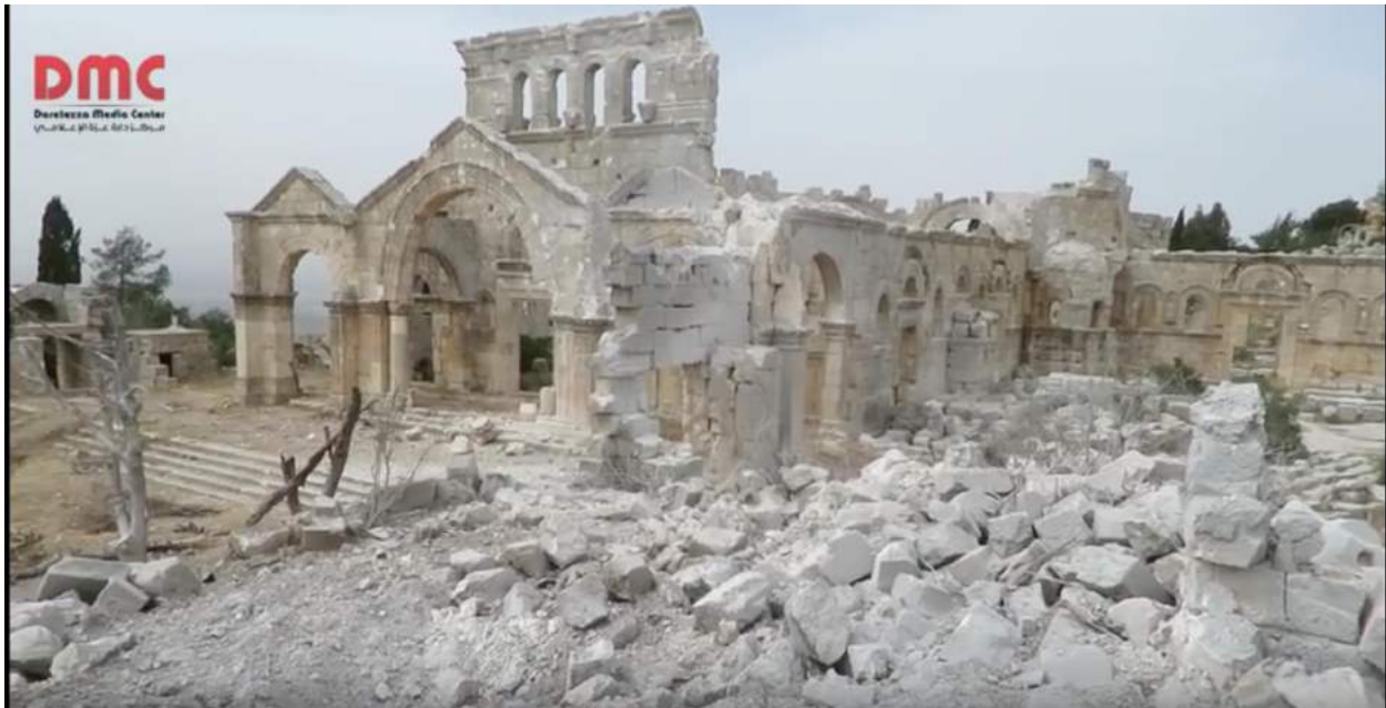
View of destruction of monastery (facing northwest) (Darezza Media Center; May 15, 2016)
