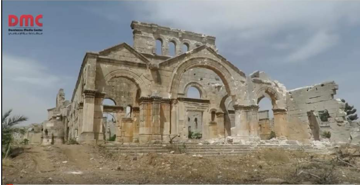
View of damage to facade of main entrance to Church of St. Simeon (looking north) (Daretezza Media Center; May 15, 2016)
