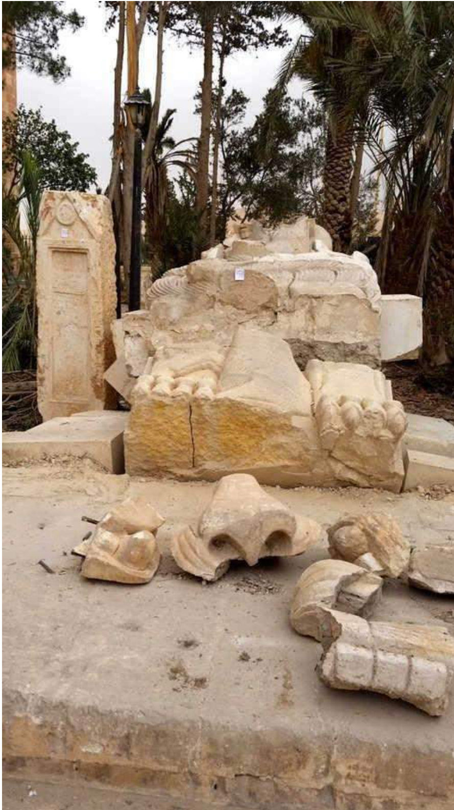
New photograph of damage to the Lion of al-Lāt (Dimashq al-An; April 12, 2016)
