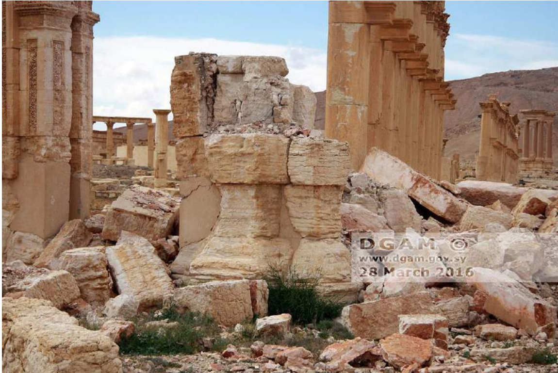
Rubble of Triumphal Arch facing west (DGAM; March 30, 2016)
