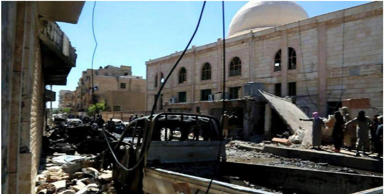
Damage to street outside of al-Nur Mosque (RBSS; April 1, 2016)
