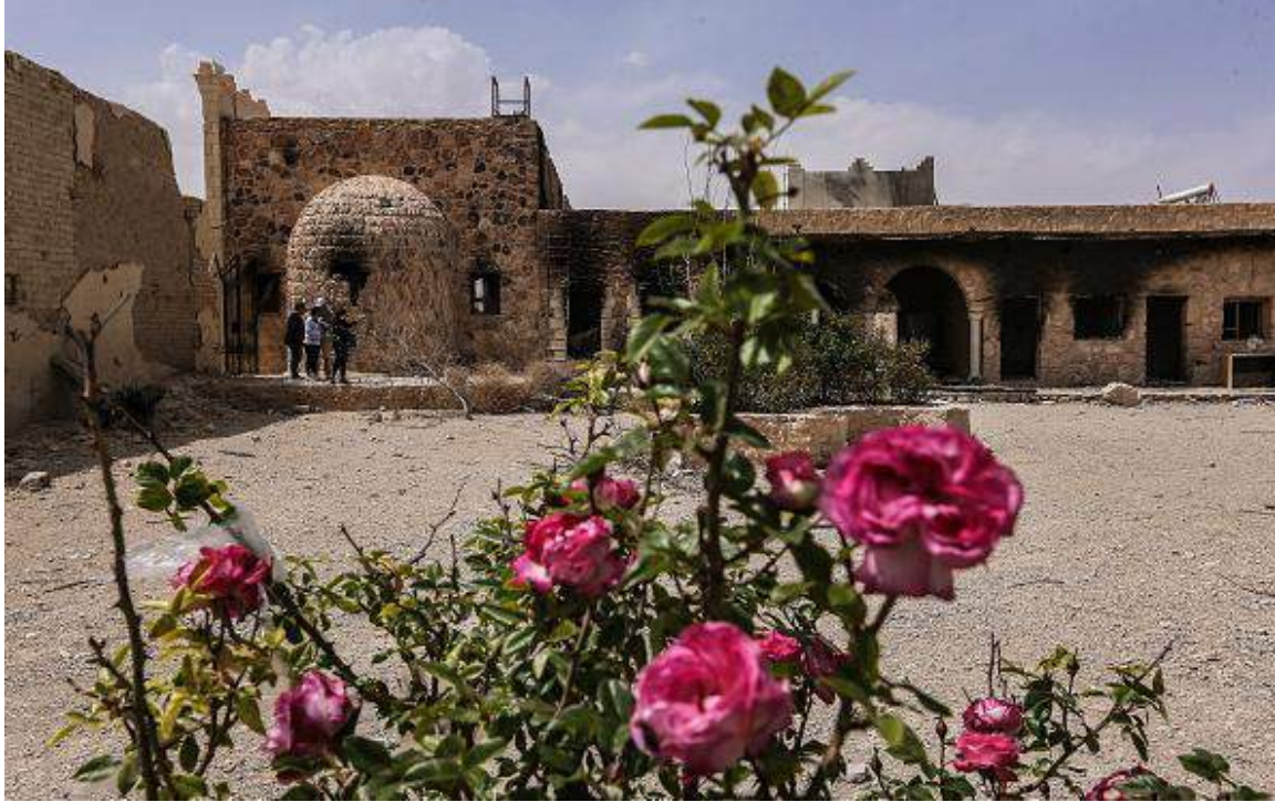
Damage to Mar Elian Monastery (Valery Sharifulin/Getty Images; April 7, 2016)
