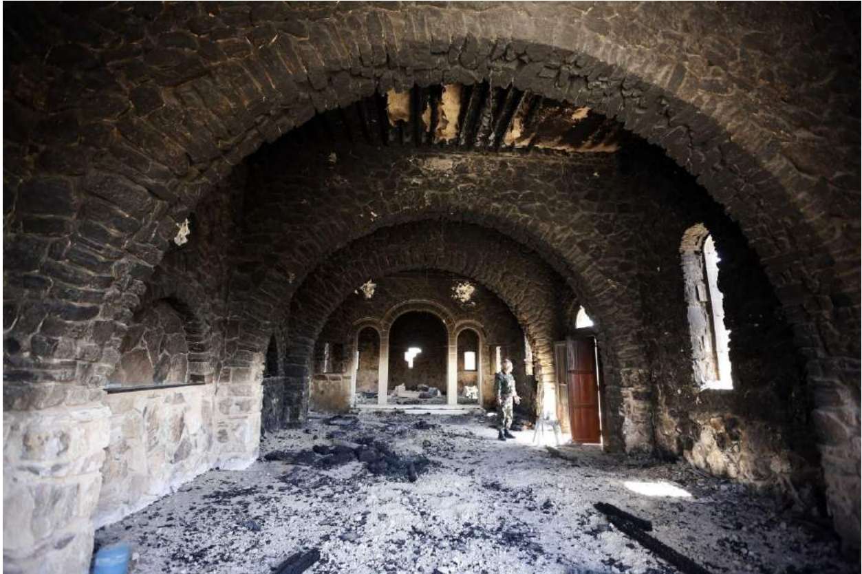
Damage to the interior of Mar Elian Monastery (AP; April 4, 2016)
