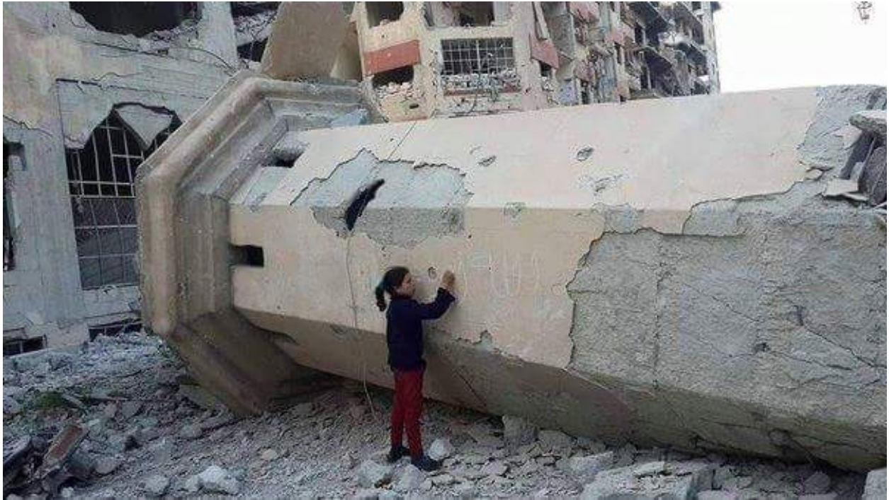
The collapsed minaret of the ar-Rawda Mosque (Conflict News/Twitter; March 30, 2016)
