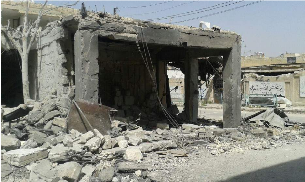
Damage surrounding al-Kabir Mosque (TDA; Provided to ASOR CHI on April 7, 2016)
