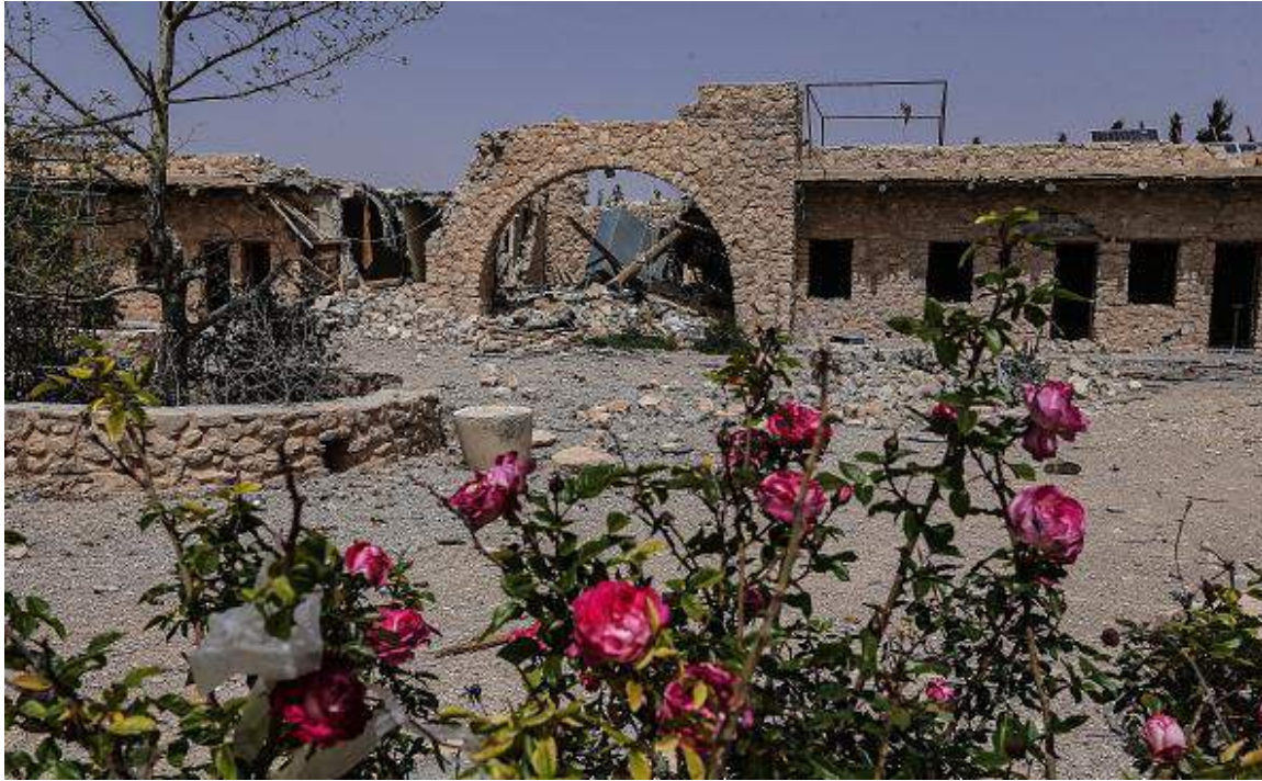
Damage to Mar Elia Monastery (Valery Sharifulin/Getty Images; April 7, 2016)
