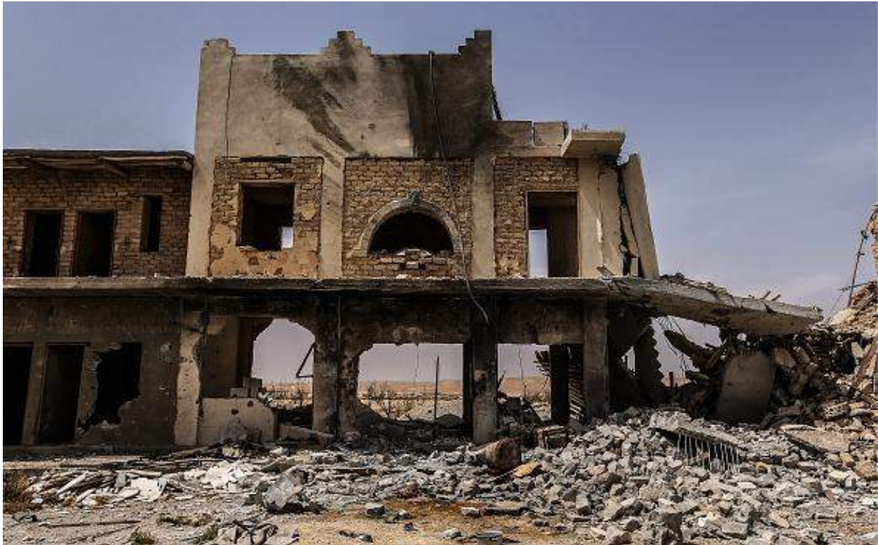
Detail of damage to Mar Elia Monastery (Valery Sharifulin/Getty Images; April 7, 2016)
