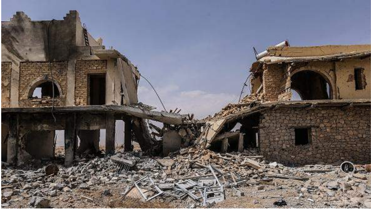
Damage to Mar Elia Monastery (Valery Sharifulin/Getty Images; April 7, 2016)
