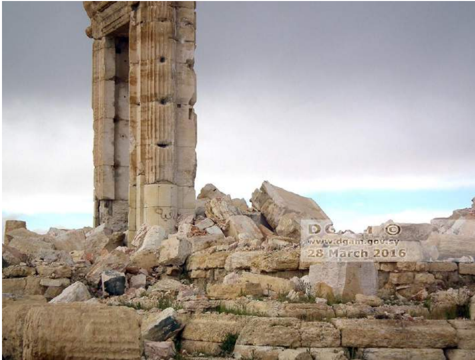
Destroyed cella of Temple of Bel, with graffiti on monumental doorway facing northeast (DGAM; March 30, 2016)
