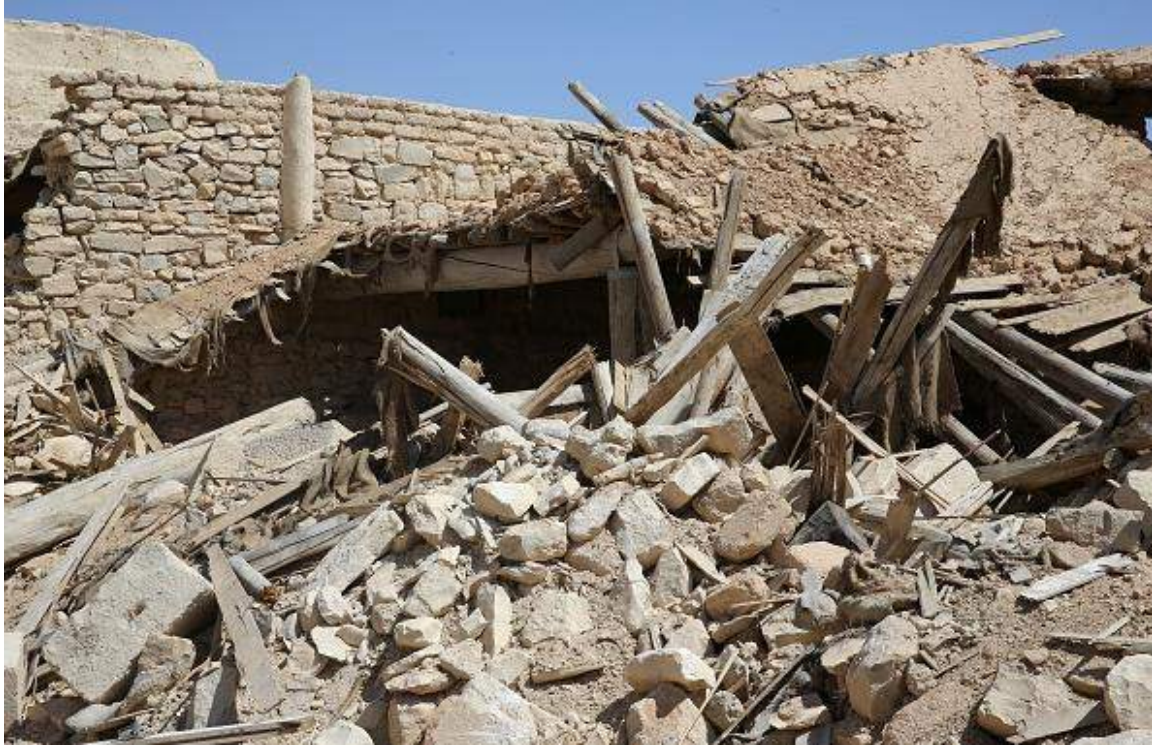
Damage to Mar Elia Monastery (Joseph Eid/Getty Images; April 4, 2016)
