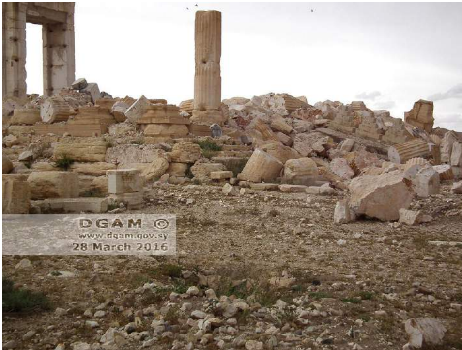
Destroyed cella of Temple of Bel with monumental doorway facing northwest (DGAM; March 30, 2016)
