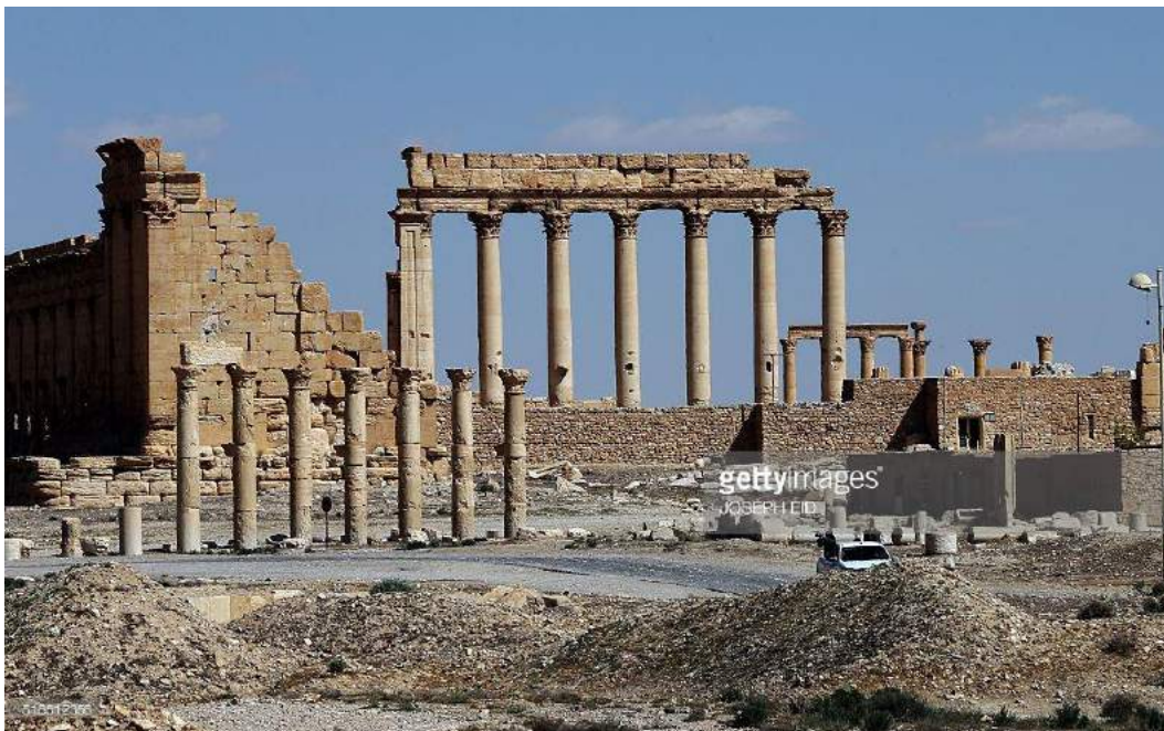
Exterior western wall of Temple of Bel with columns of via sacra in front, and piles of debris in foreground (Joseph Eid/Getty; March 31, 2016) 121
