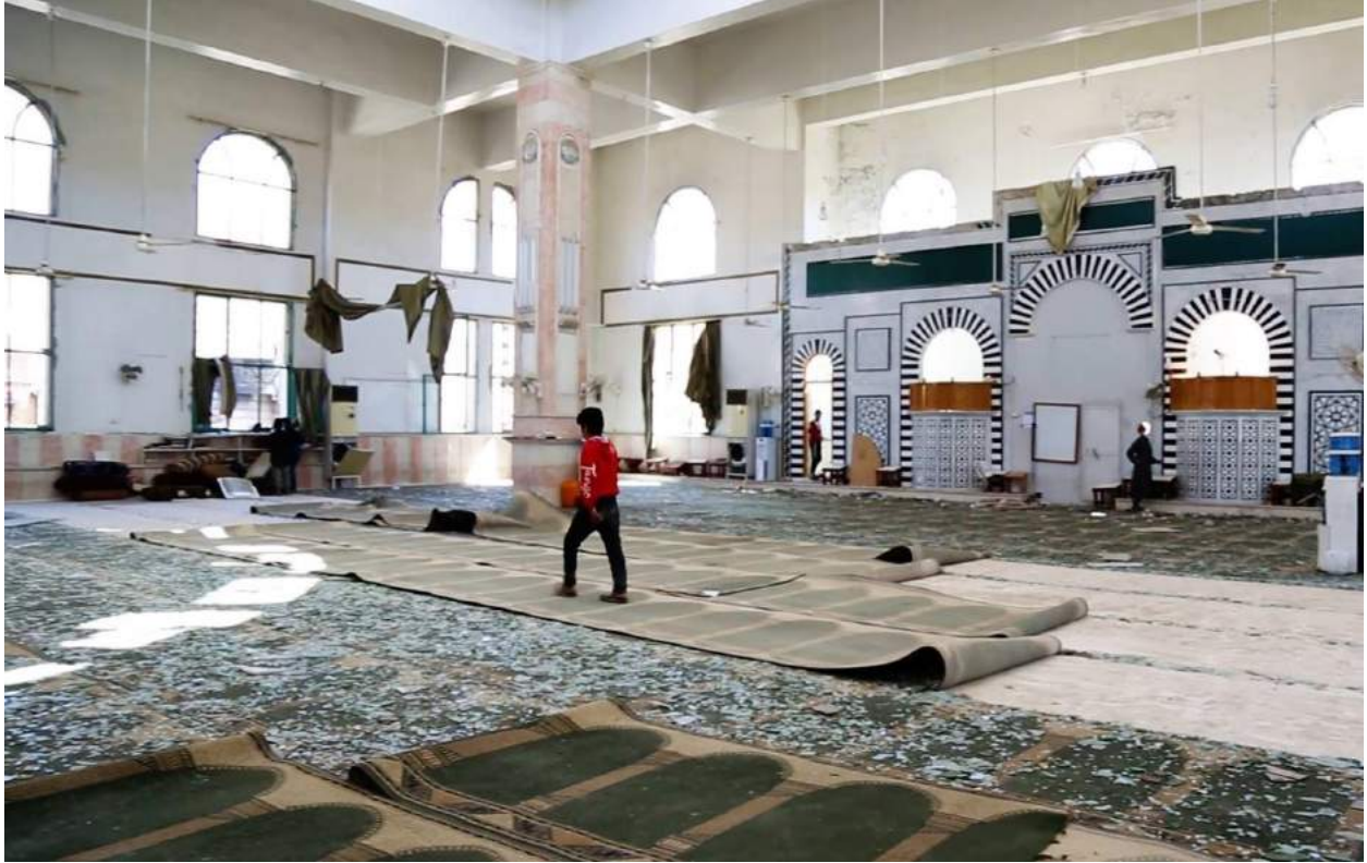
Broken glass and debris inside al-Nur Mosque (RBSS; April 1, 2016)
