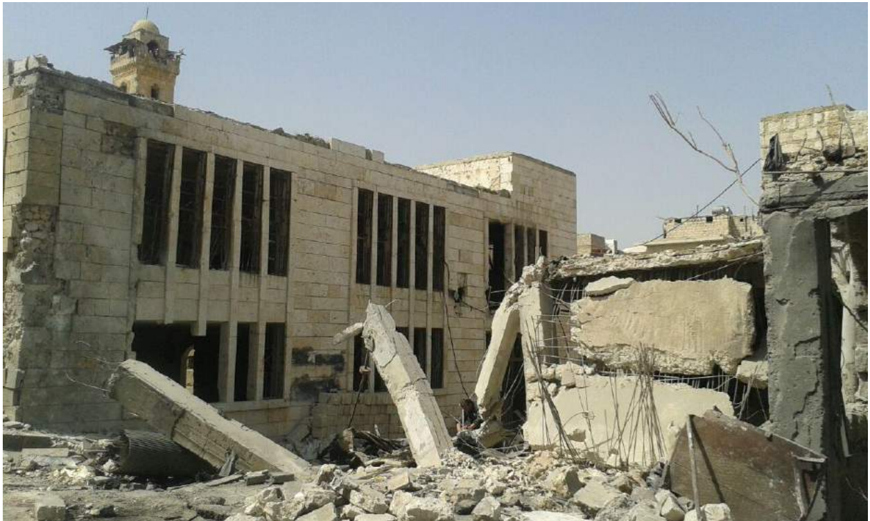
Damage to the exterior of al-Kabir Mosque (TDA; Provided to ASOR CHI on April 7, 2016)
