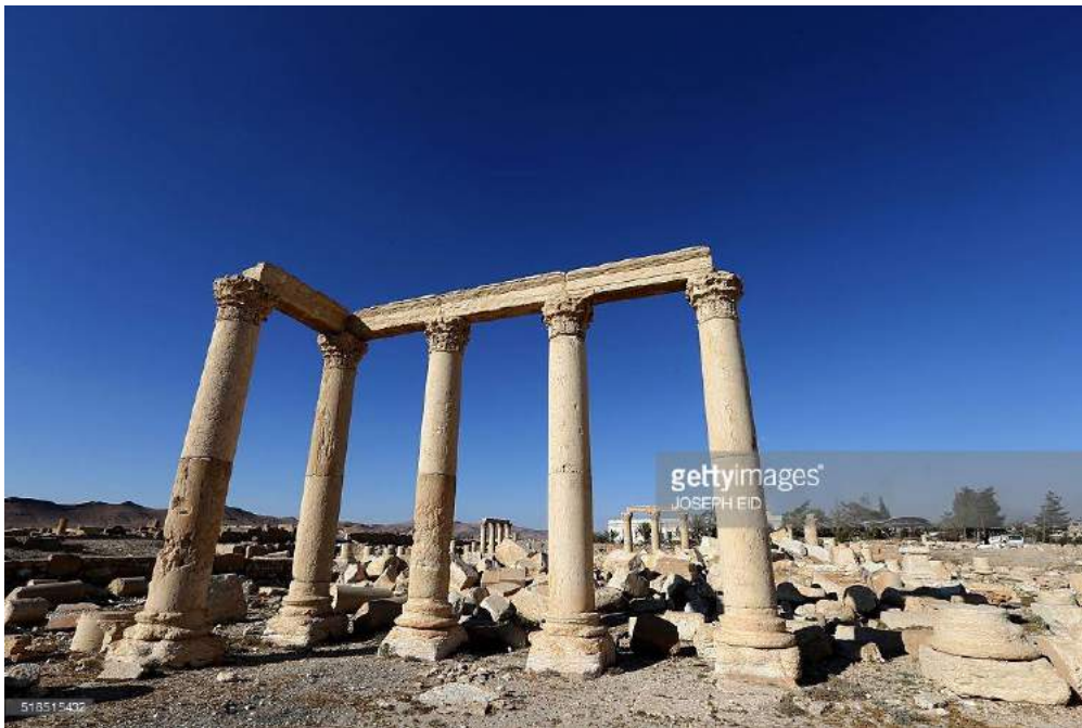
Undamaged portico of Temple of Baal-Shamin southwest courtyard facing northeast (Joseph Eid/Getty; March 31, 2016) 113
