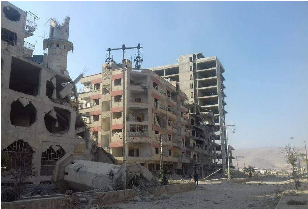
Damage to ar-Rawda Mosque and minaret (SNHR; March 30, 2016)
