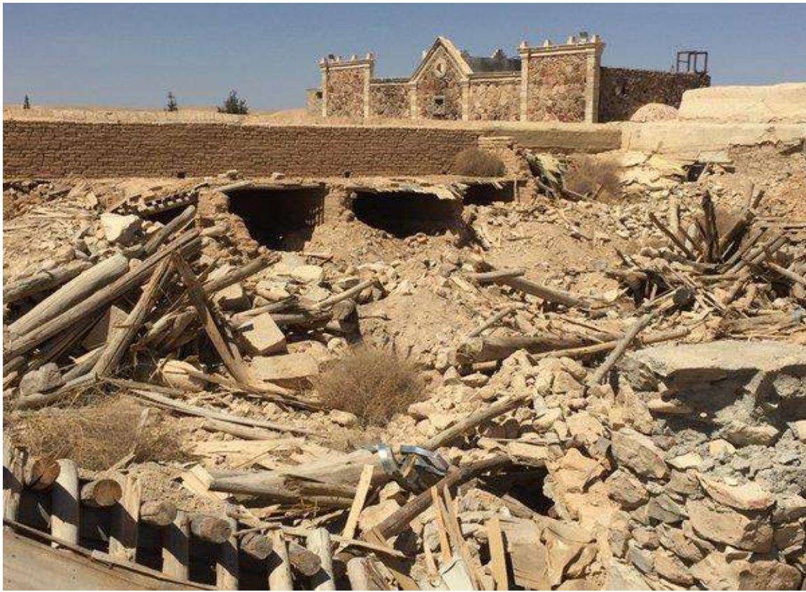
Damage to Mar Elia Monastery (Lindsey Hilsum; April 4, 2016)
