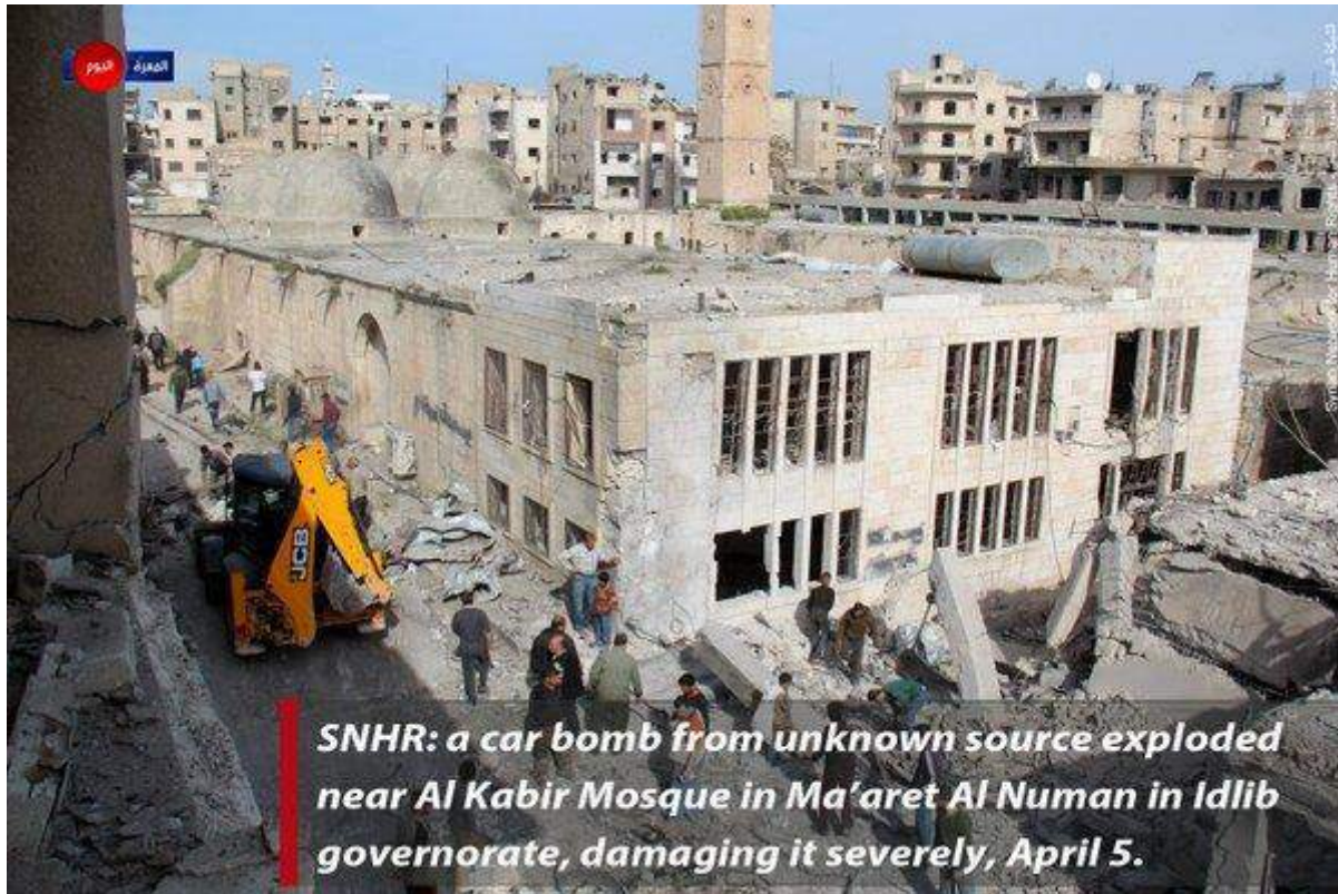
Damage to southeast side of al-Kabir Mosque (SNHR; April 5, 2016)
