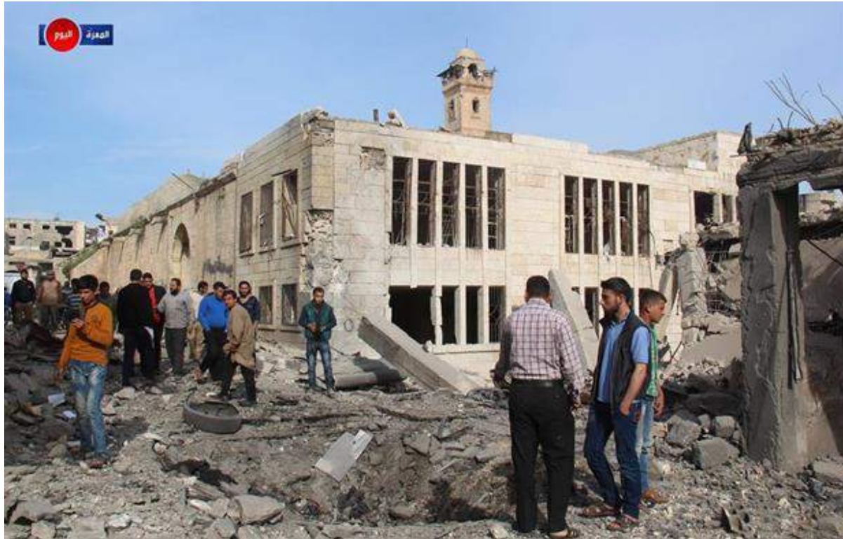
Damage to southeast side of al-Kabir Mosque (Now Media; April 5, 2016)
