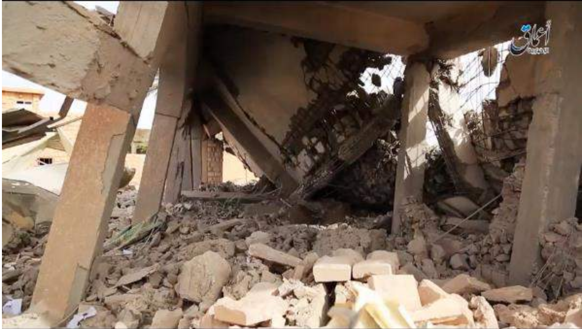
Still image of the damage to Al-Farooq Mosque (Internet Archive; March 15, 2016)
