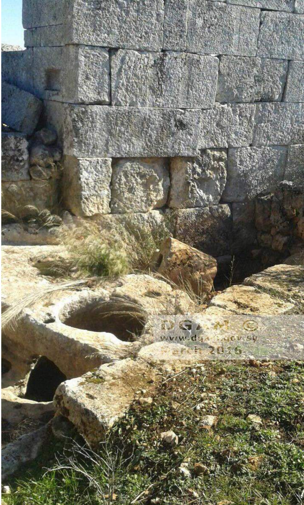
Possible damage from illegal excavation at Dahes (DGAM; March 9, 2016)
