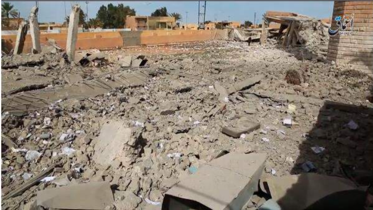
Still image of the damage to Al-Farooq Mosque (Internet Archive; March 15, 2016)
