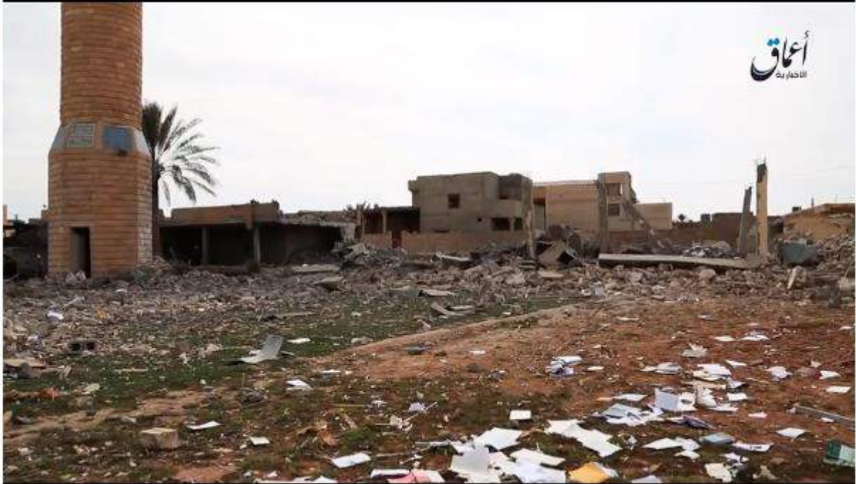
Still image of the damage to the surrounding area of Al-Farooq Mosque (Internet Archive; March 15, 2016)
