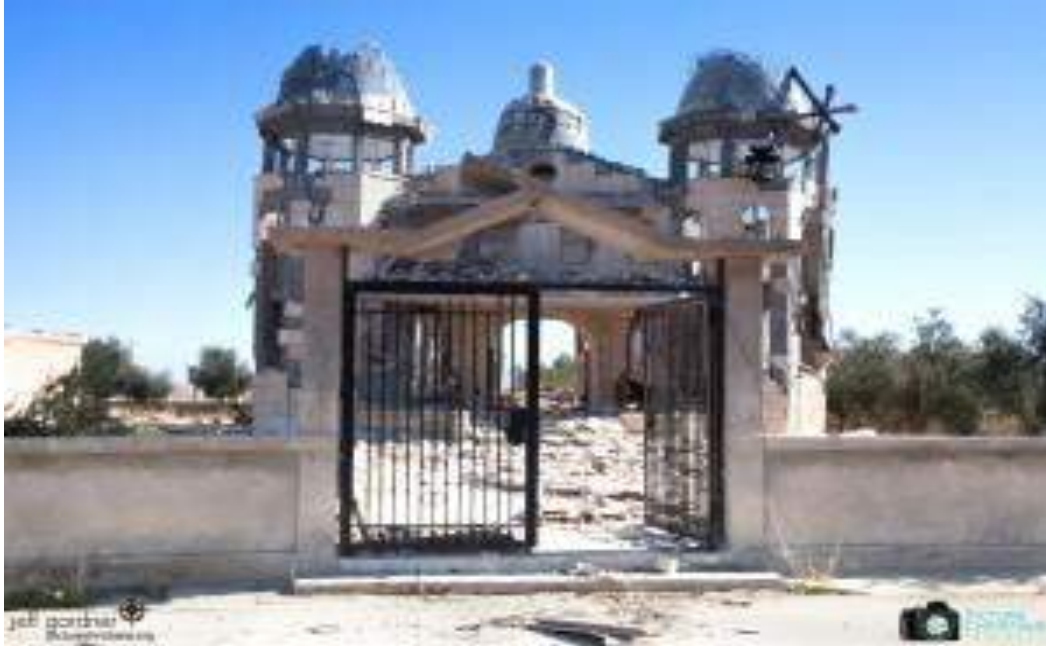
Damage to Mar Shimon Church, Abu Tina (The Stream; January 16, 2016)
