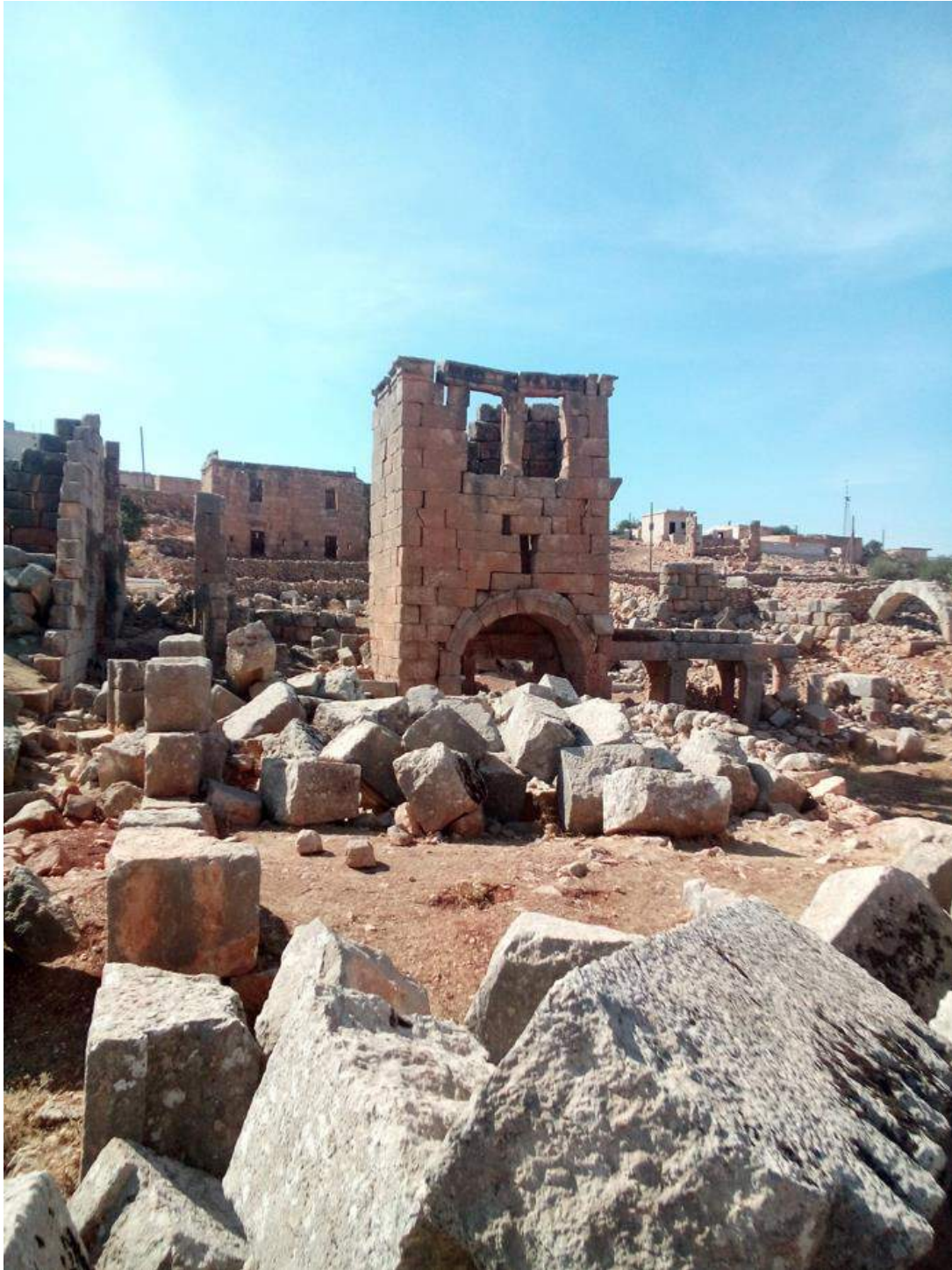
Damage due to weathering and neglect
