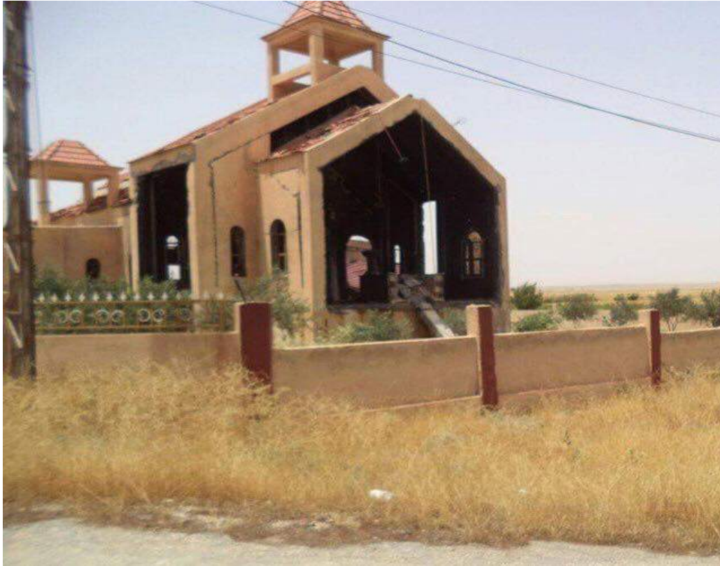
Damage to Mar Giorgis Church, Qabr Shamiya (Halmon.net; Posted June 5, 2015)
