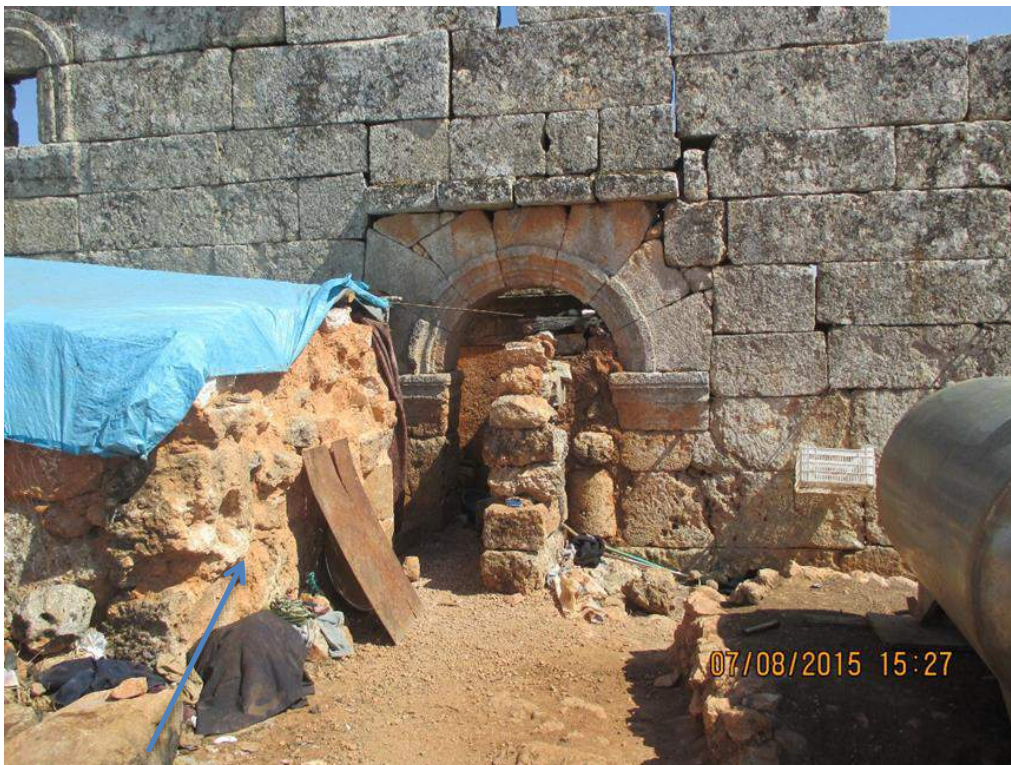
Human occupation and reuse of buildings. Note use of local stone, mud, and straw in building construction.
