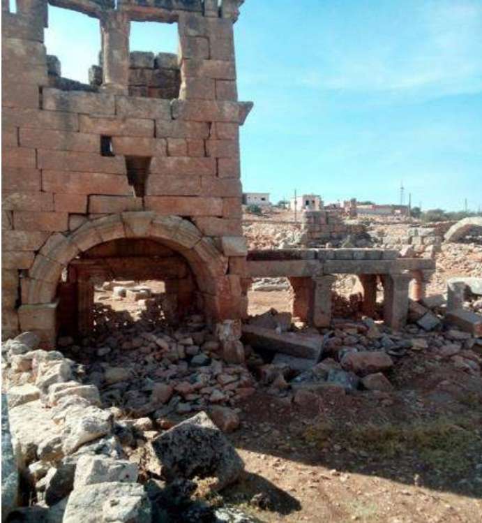
Damage caused by neglect
