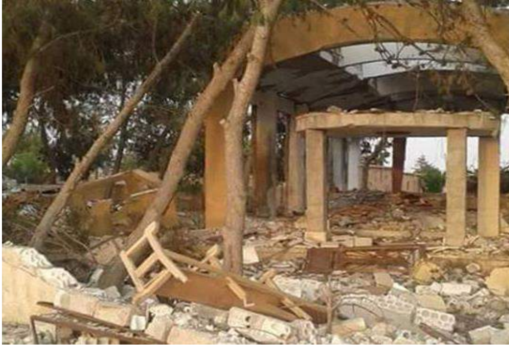
Extensive damage to Mar Sleewa Church, Tel Talaa (Halmon.net; Posted April 15, 2015)
