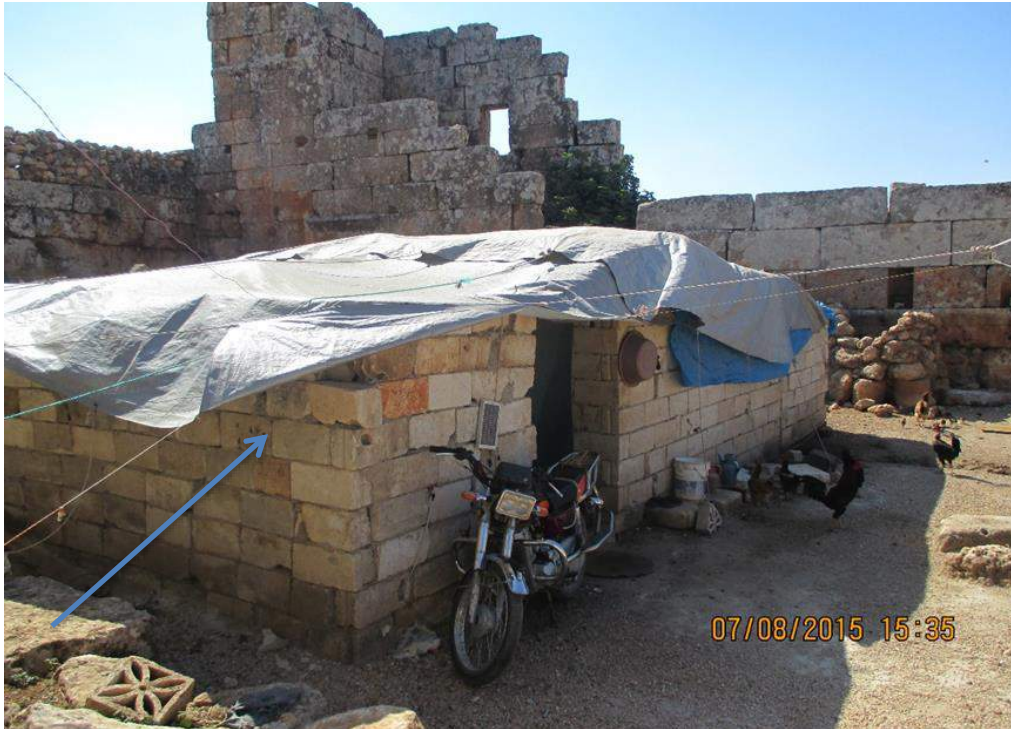
Partial or temporary dwelling structures with plastic tarpaulin for a roof.
