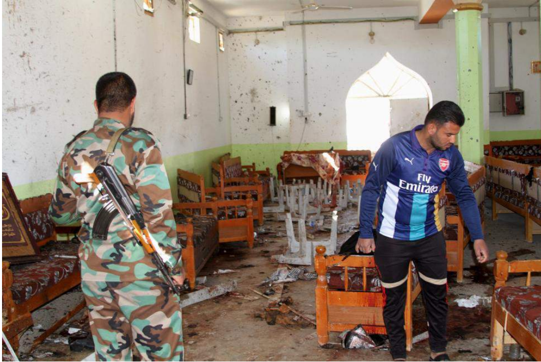
Interior of the Shia Mosque in Muqdadiya showing material damage (Reuters; March 1, 2016)
