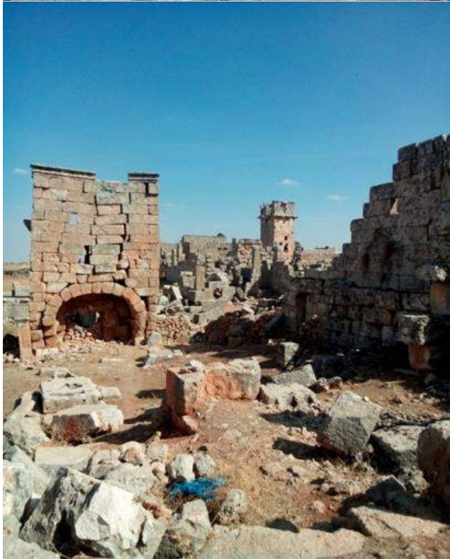
Damage caused by neglect
