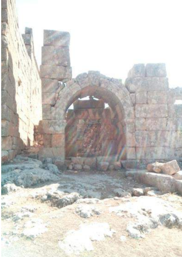
Damage caused by neglect
