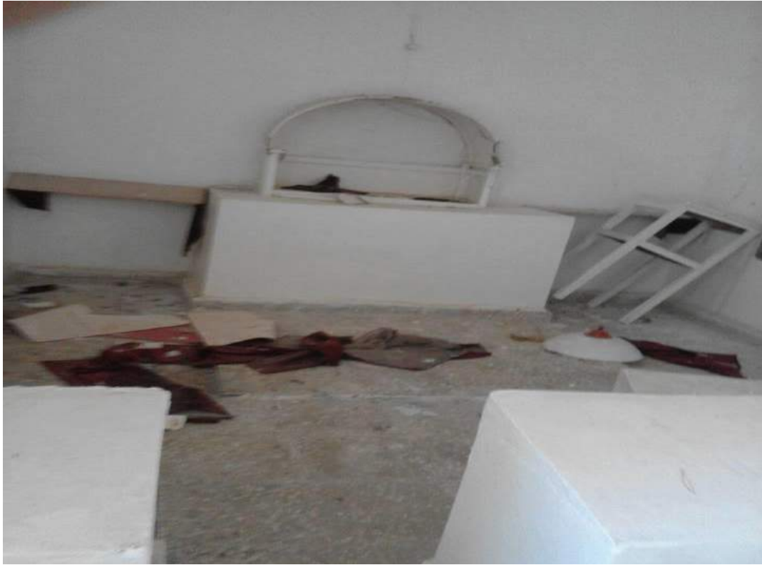
Damage to Mar Shimon Prusbai Church, Tel Kharita (Halmon.net; Posted June 16, 2015)
