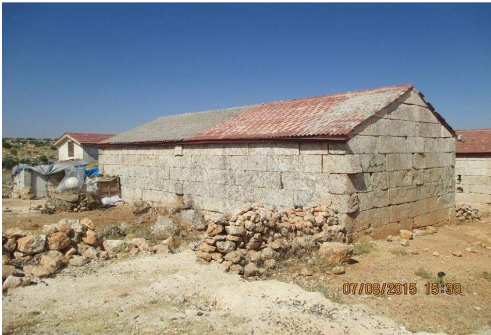
Human occupation and reuse of buildings at Serjilla by displaced Syrian refugees. The stone buildings provide shelter from the weather and the indiscriminate bombardment by regime forces. Some structures are permanent whilst others appear partial or temporary.
