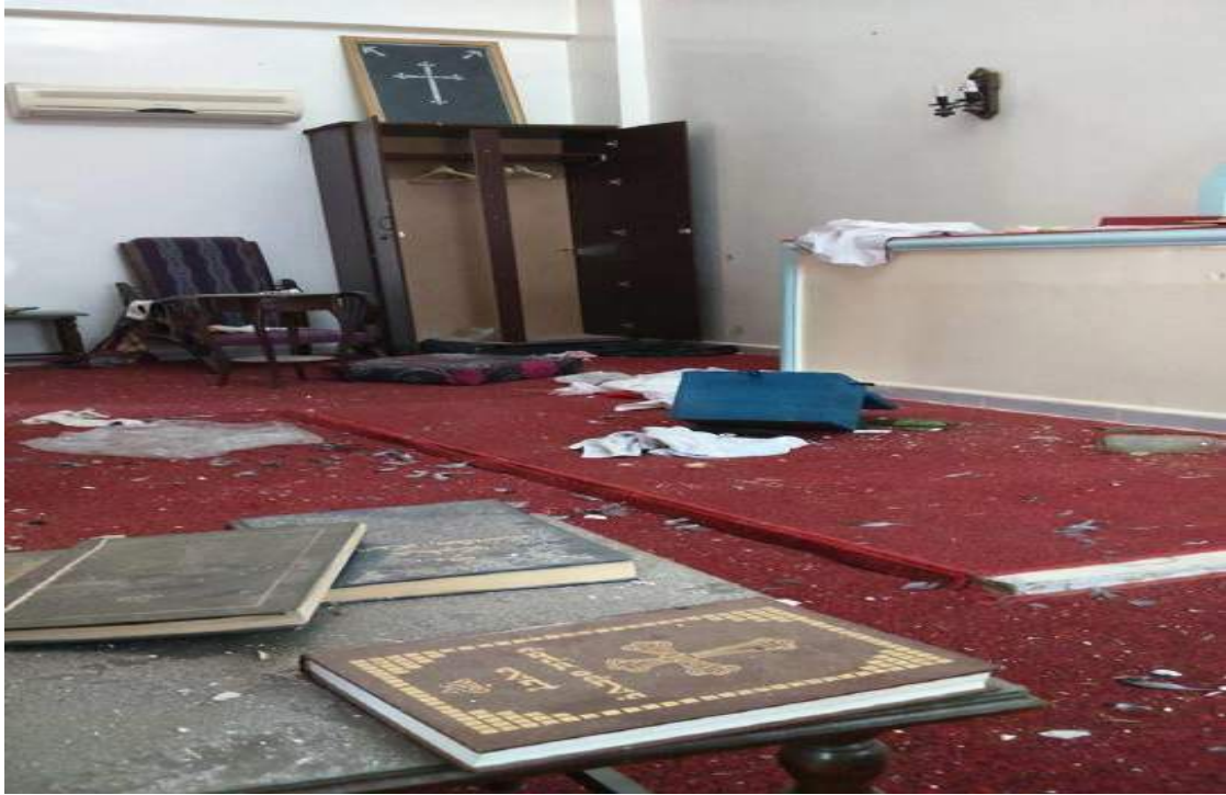
Interior damage to Mar Sawa Church, Tel Jadiya (Halmon.net; Posted June 5, 2015)
