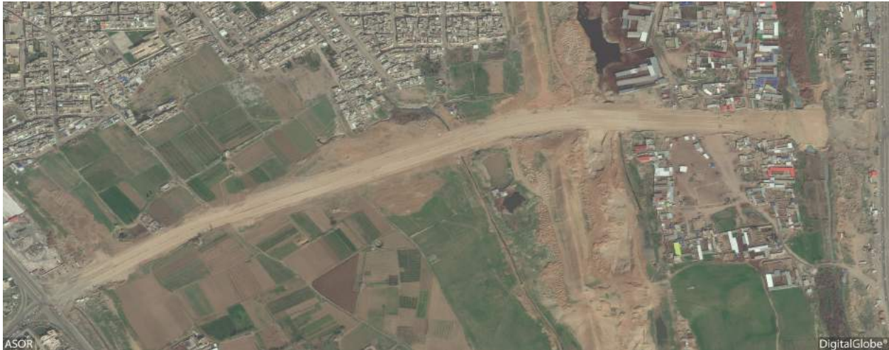
Damage from new four-lane road in southern half of Nineveh (DigitalGlobe; February 12, 2016)
