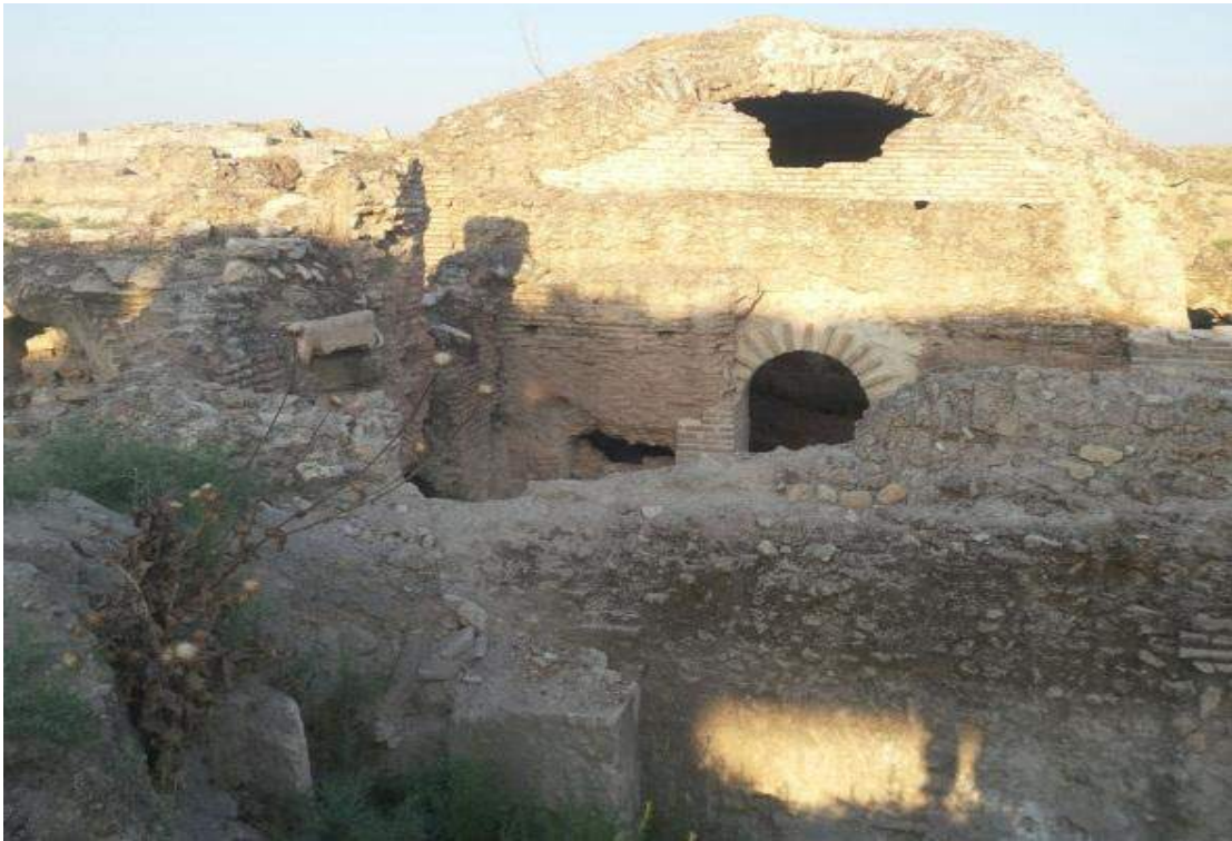
Damage from Combat and Exposure to the Elements
