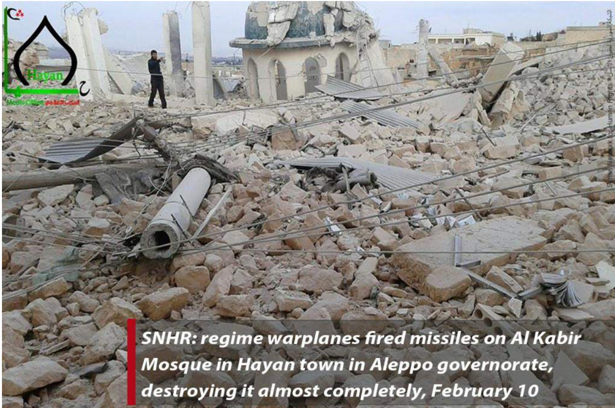
Destruction to Al Kabir Mosque (SNHR; February 10, 2016)
