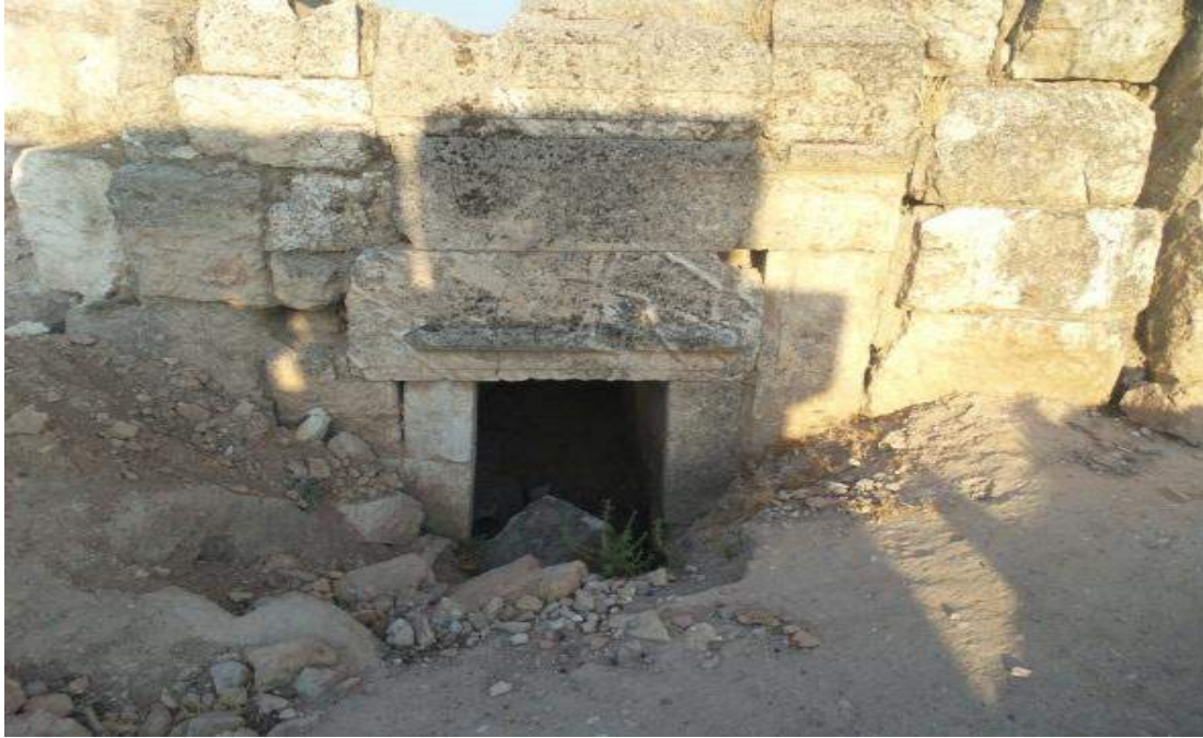
Evidence of Looting
