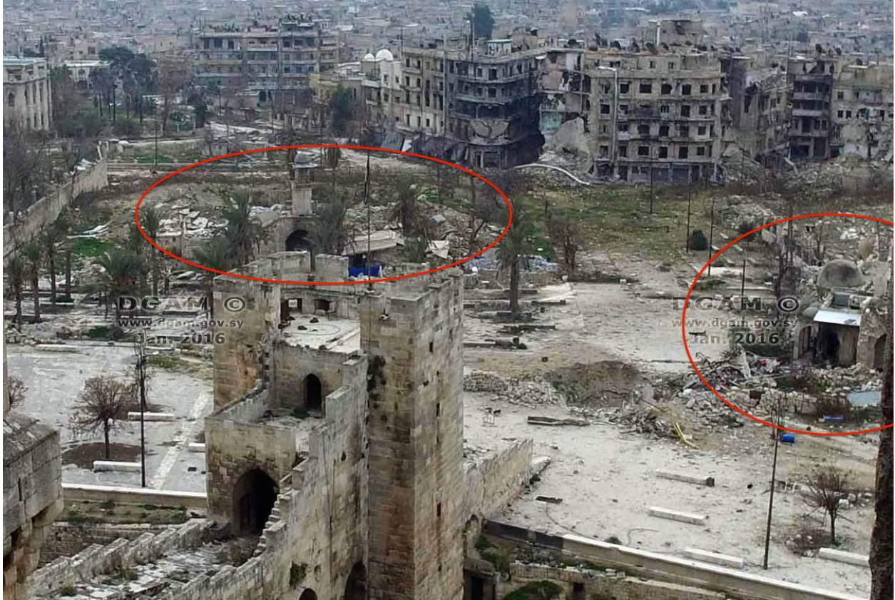
Severe damage to Sultaniyah Mosque and Khan al-Shouneh (DGAM; published February 1, 2016)
