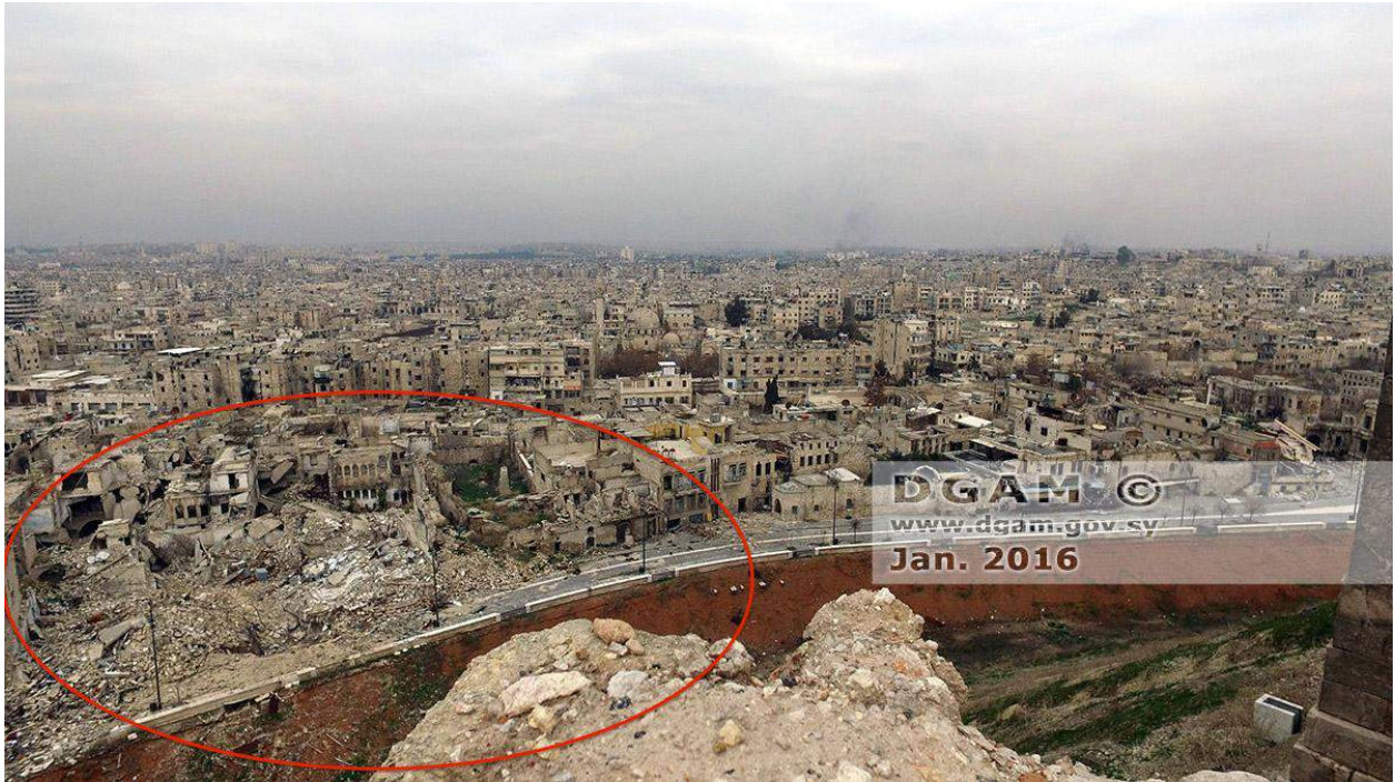
Destruction of buildings on Hawl al-Qalaa St. (DGAM; published February 15, 2016)
