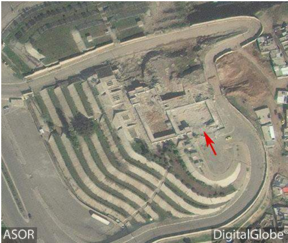
New damage to the courtyard wall of the Nebi Yunus Complex (DigitalGlobe; February 12, 2016)
