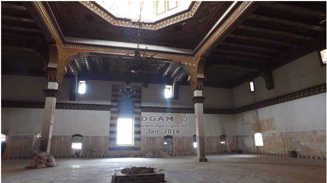
Removal of wooden panels on walls and pillars, removal or destruction of stained glass windows, damage to chandelier and fountain in Mamluk Throne Hall (DGAM; published February 1, 2016)
