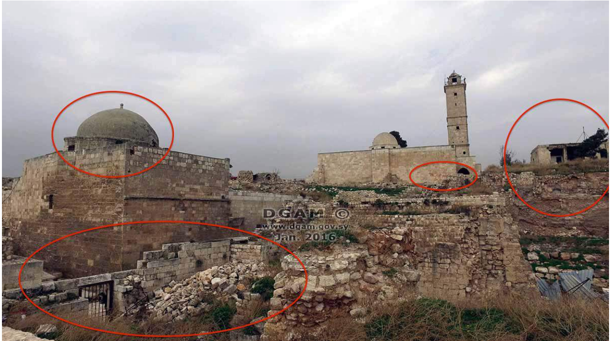
Damage to dome of Ibrahim Mosque, debris in Ayyubid palace and Temple of Hadad area, severe damage to Citadel Museum, graffiti on al-Kabir Mosque (DGAM; published February 1, 2016)
