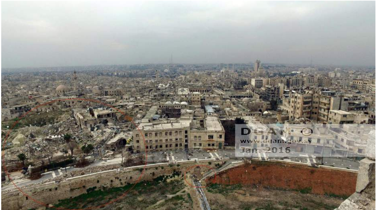
Damage to outer wall of Citadel and destruction of Carlton Citadel Hotel (DGAM; published February 15, 2016)
