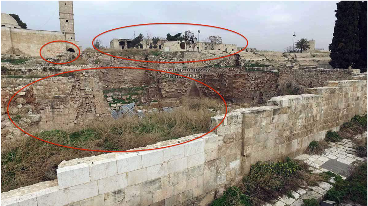
Debris in Ayyubid palace and Temple of Hadad area, severe damage to Citadel Museum, graffiti on al-Kabir Mosque (DGAM; published February 1, 2016)
