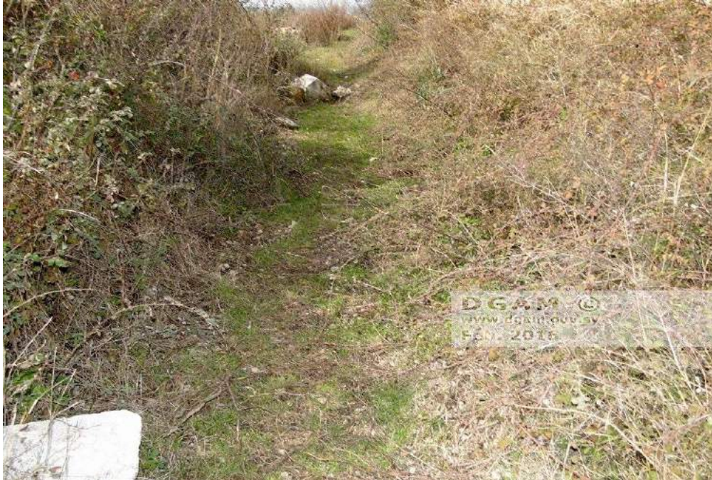
Overgrown vegetation (DGAM; February 16, 2016)
