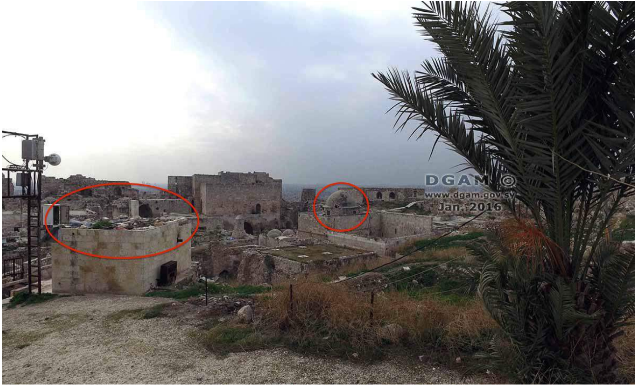
Trash and debris on roof of structure adjacent to theater, damage to dome of Ibrahim Mosque (DGAM; published February 1, 2016)
