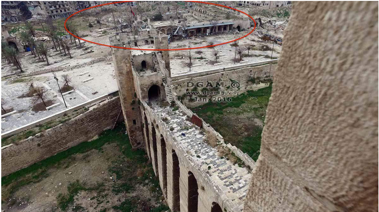
Destruction of Khan al-Shouneh and Khusrawiyah Mosque (DGAM; published February 1, 2016)
