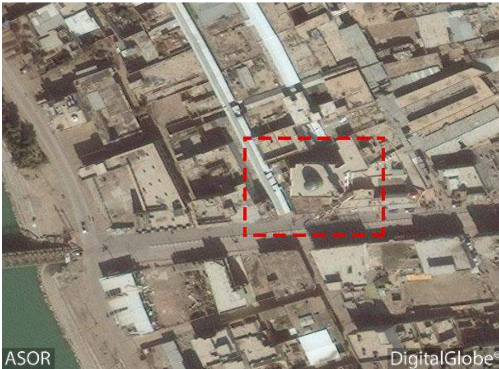
al-Hajj Shaker al-Dahi Mosque, Fallujah, Iraq with no discernible damage (January 29, 2016)
