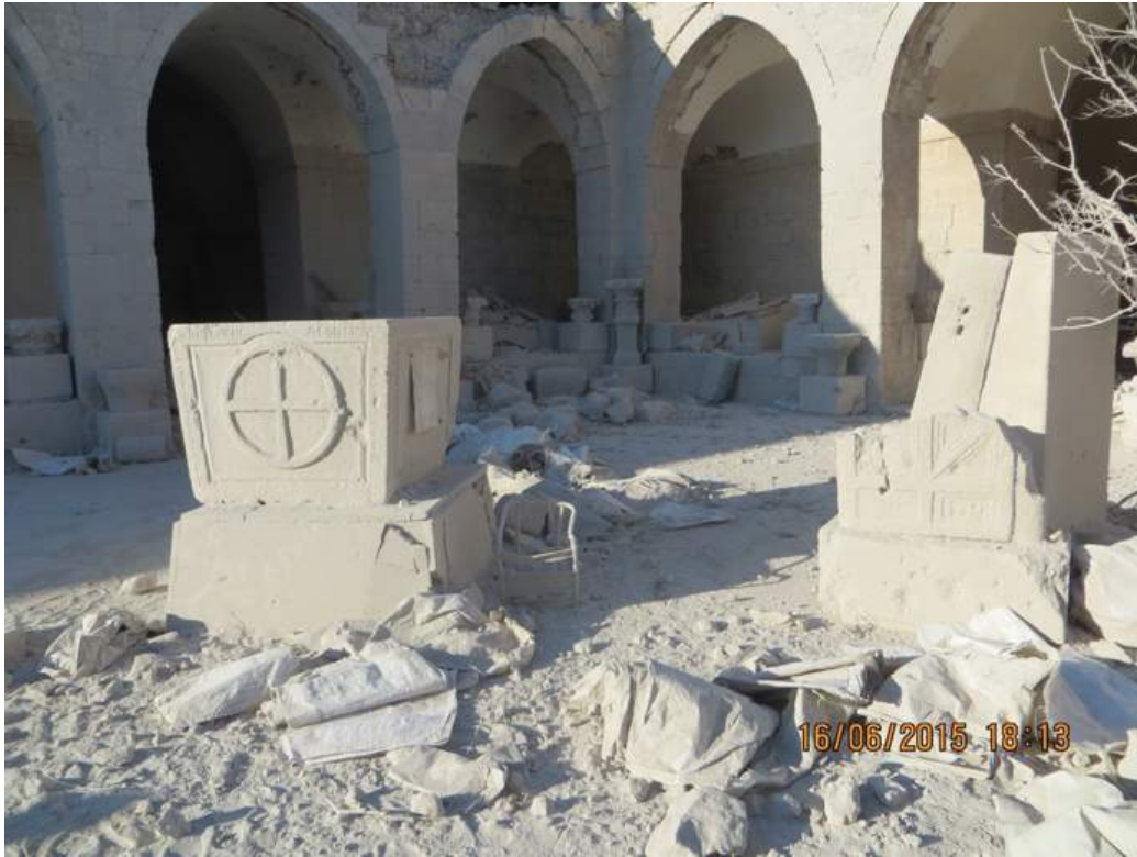
Sand bags scattered due to the explosion.
