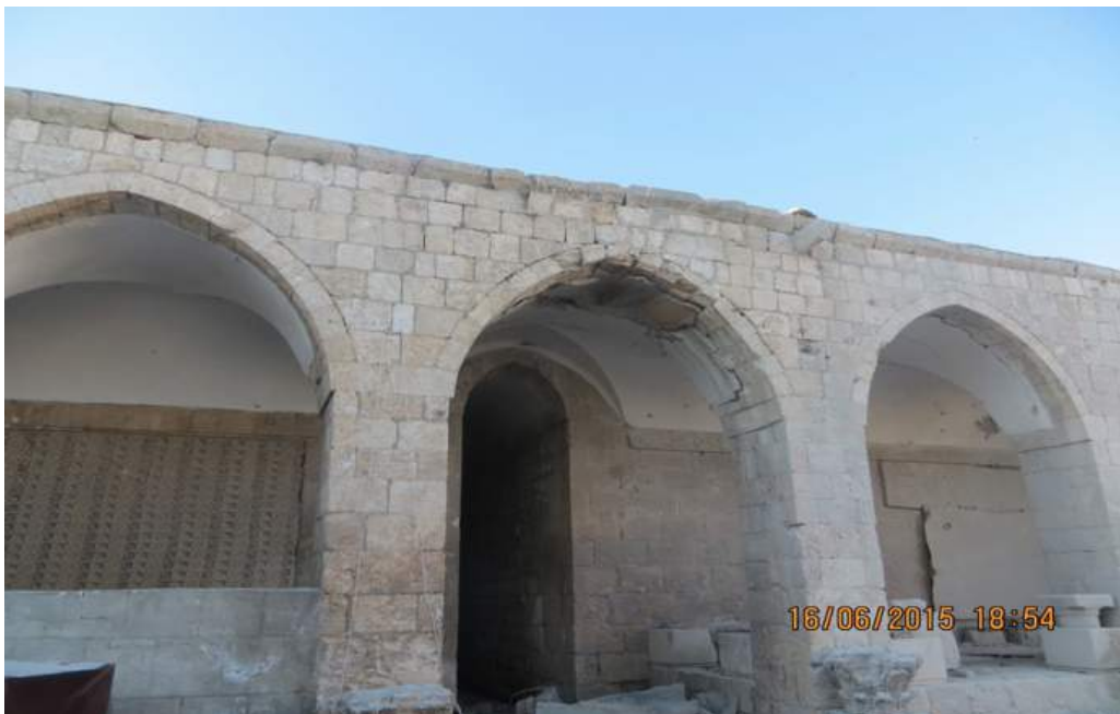
The front, which was repaired earlier.
