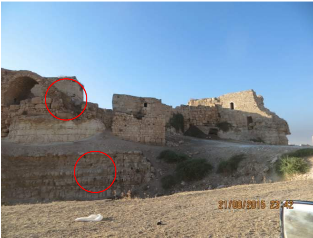
Locations that need urgent repairs to fortify calcareous layer beneath the citadel
