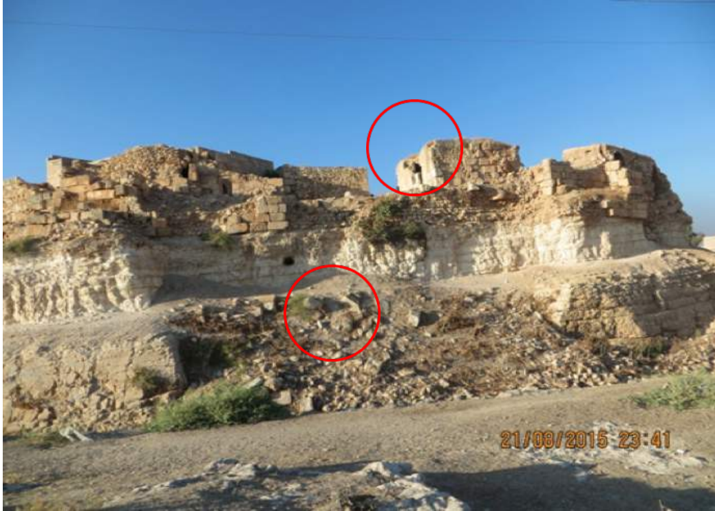
Locations that need urgent repairs to fortify calcareous layer beneath the citadel
