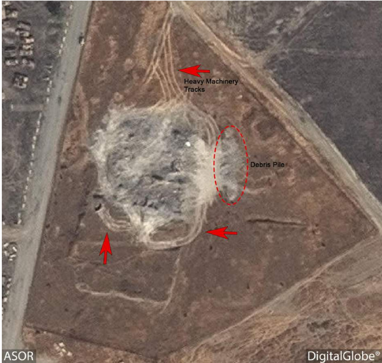
Monastery of St. Elijah — now mounds of rubble with tire tracks (marked with red arrows) and a new debris pile (DigitalGlobe; September 28, 2014)
