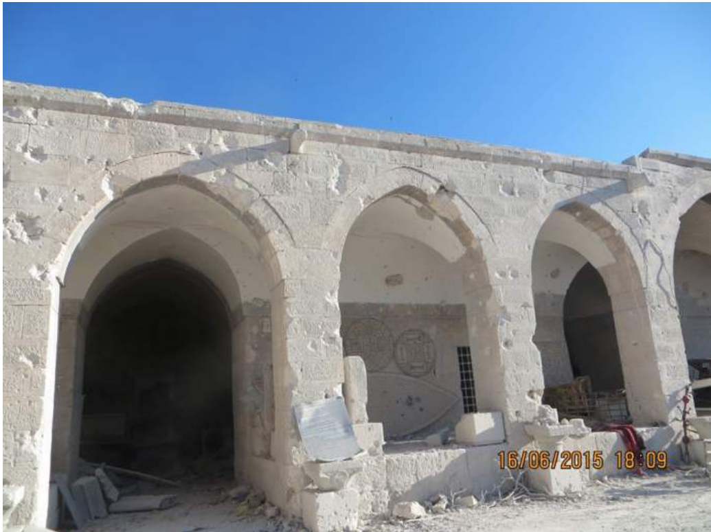
The entrance of the first wing.
