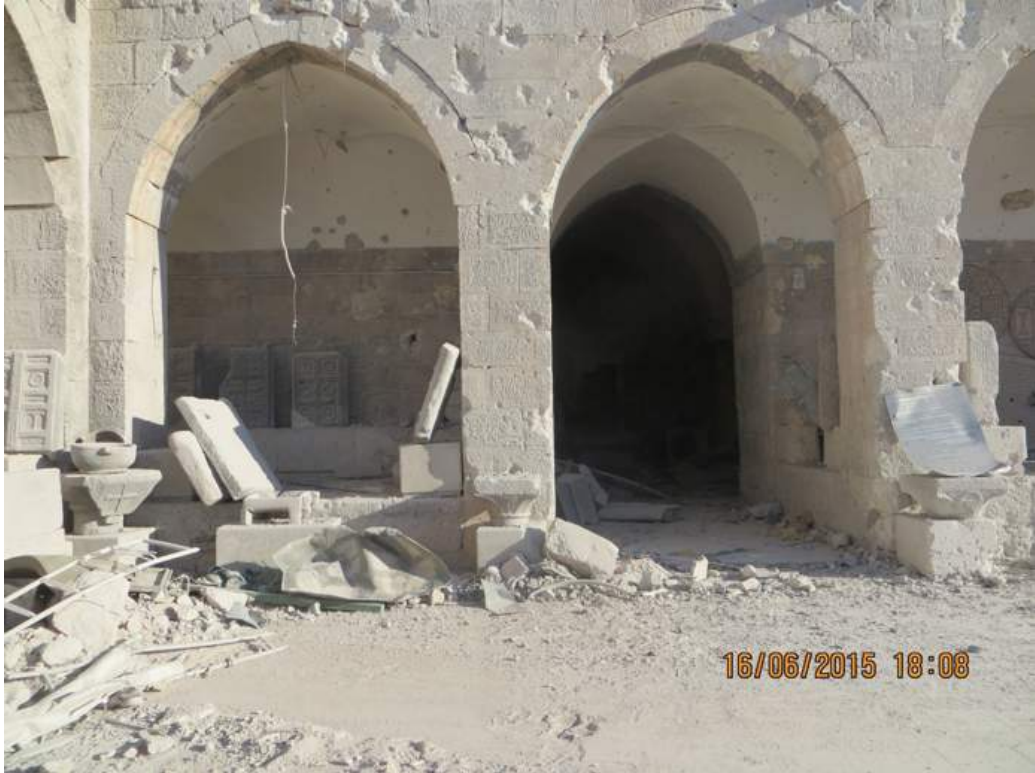
The entrance of the first wing.
