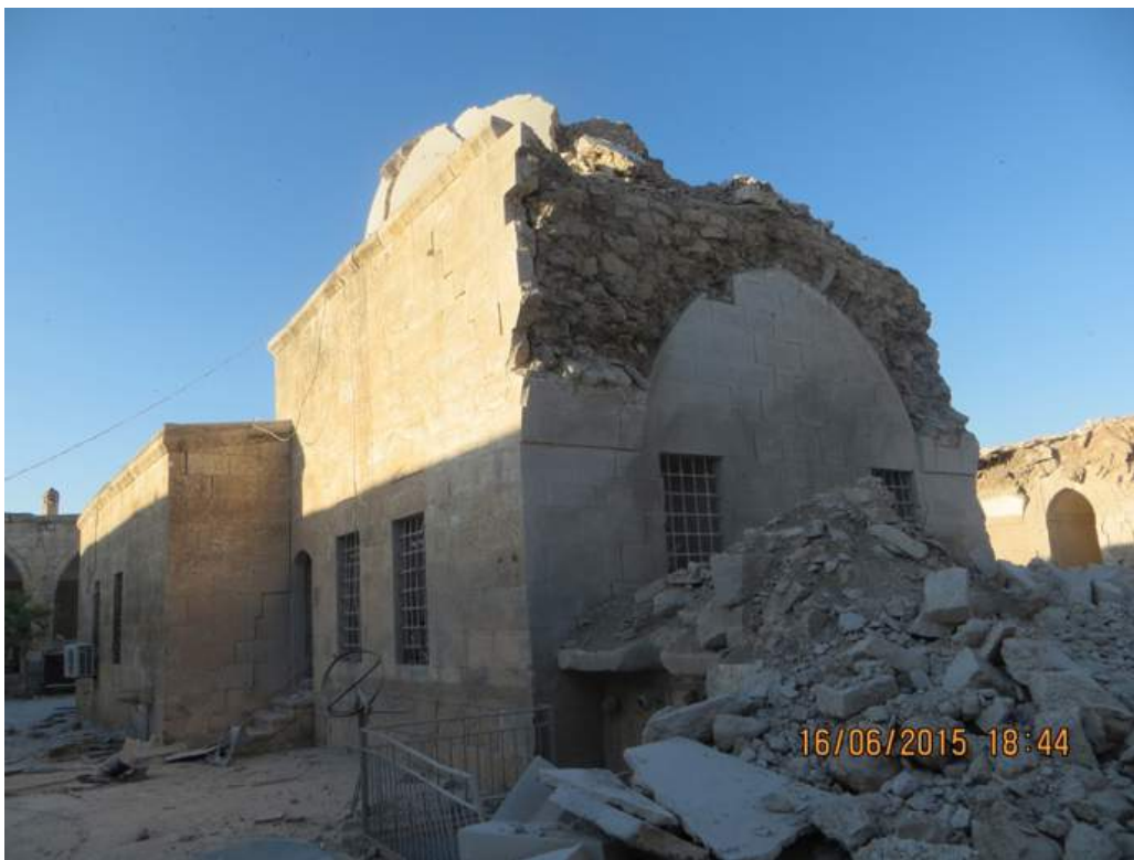
The southeastern corner of the mosque
