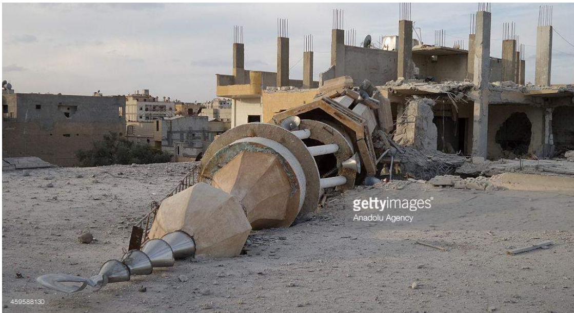
Collapse of Hinni Mosque minaret (Anadolu Agency Getty Images; November 26, 2014)
