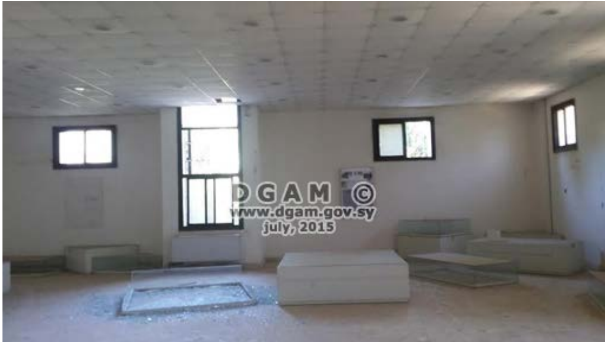
Museum of Daraa, interior damage (DGAM; July, 3, 2015)
