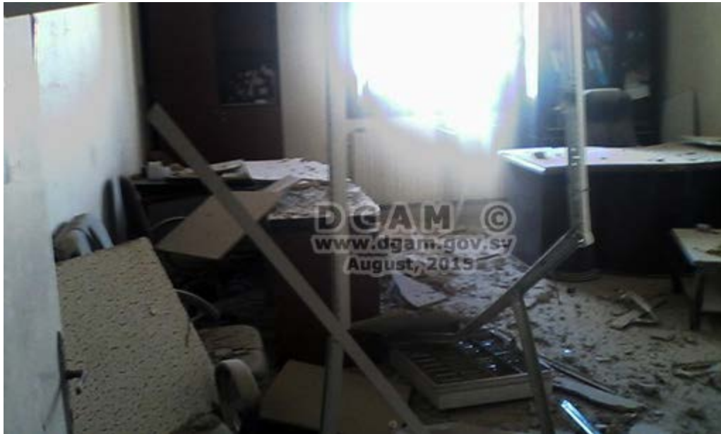
Museum of Daraa, interior damage (DGAM; August 12, 2015)
