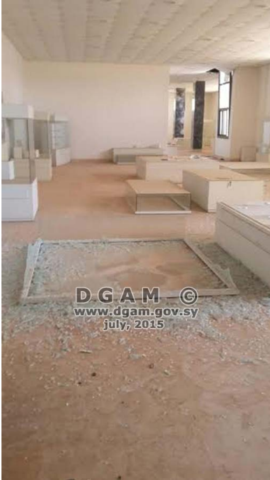
Museum of Daraa, interior damage (DGAM; July, 3, 2015)
