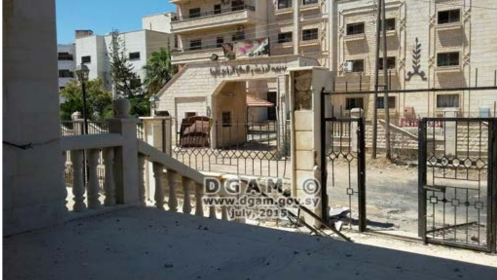
Museum of Daraa, exterior damage (DGAM; July, 3, 2015)
