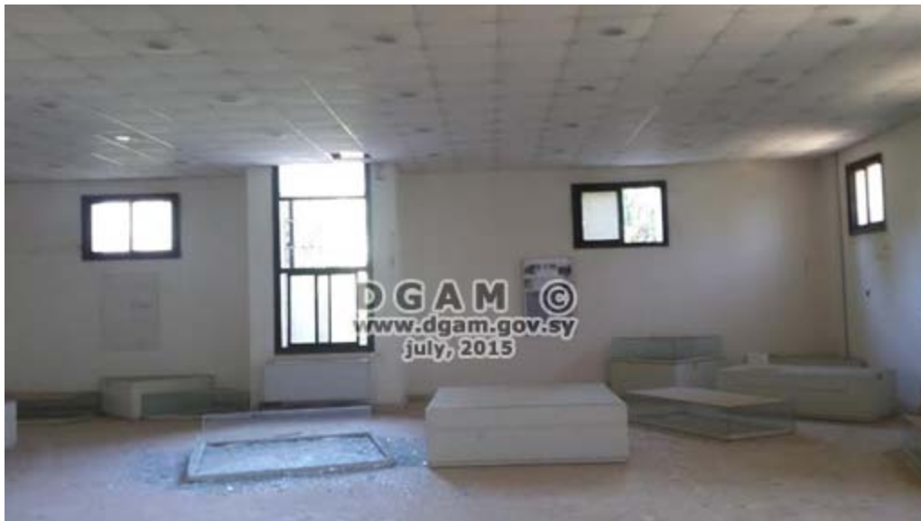
Museum of Deraa, interior damage (July 3, 2015; DGAM)
