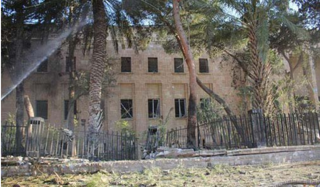
Museum of Palmyra, exterior damage (July 29, 2015; DGAM)
