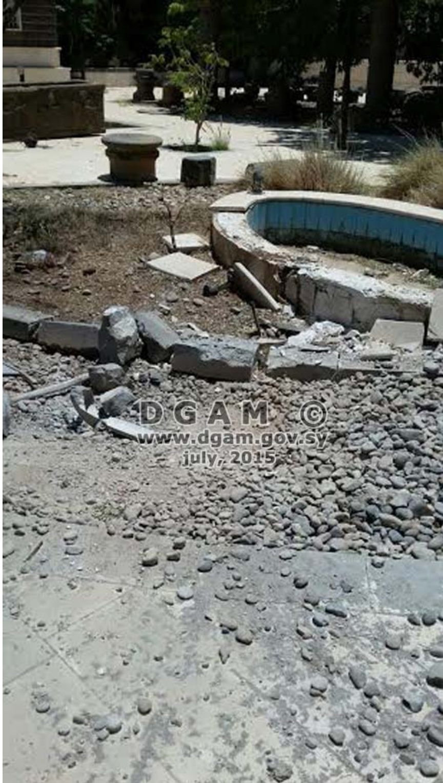
Museum of Deraa, exterior damage (July 3, 2015; DGAM)
