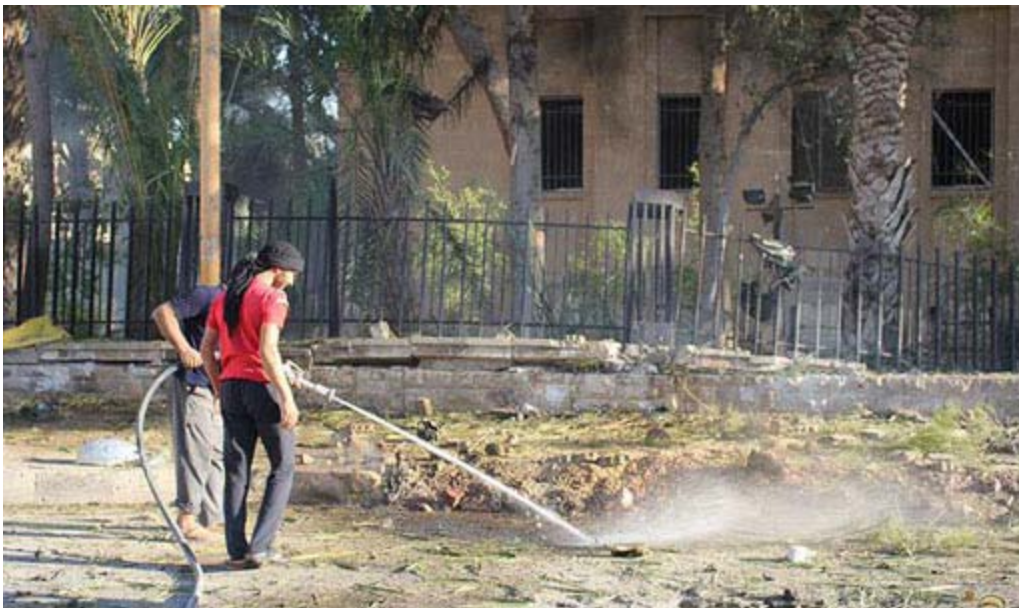
Museum of Palmyra, exterior damage (July 29, 2015; DGAM)
