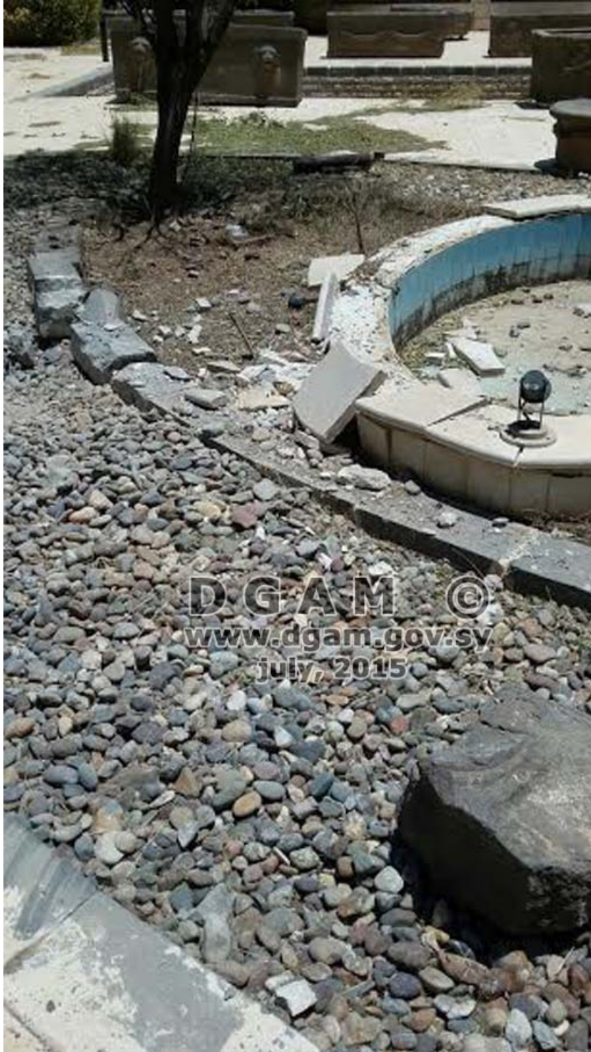
Museum of Deraa, exterior damage (July 3, 2015; DGAM)
