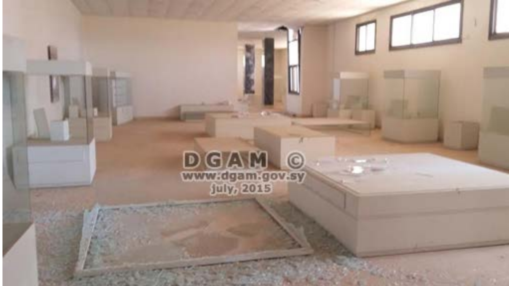
Museum of Daraa, interior damage (DGAM; July 3, 2015)
