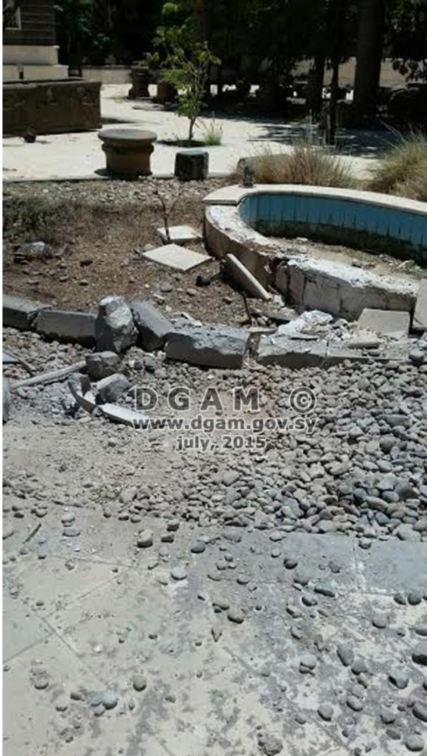
Museum of Daraa, exterior damage (DGAM; July 3, 2015)
