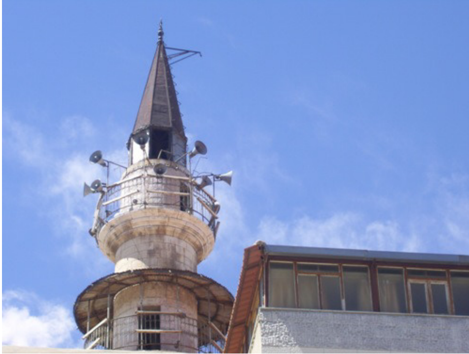
Image showing damage to Great Mosque of Jobar, exterior, minaret (APSA)
