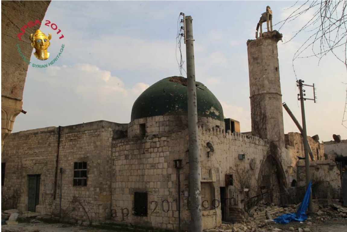
The current state of the Bardabak (Qastal al-Haramia) Mosque, Qastal al-Harami neighborhood, Aleppo (APSA)
