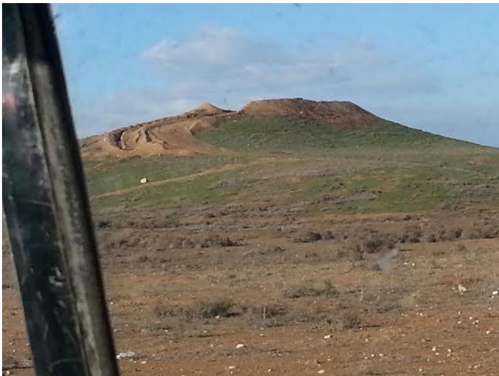
Bulldozing at Tell Harmal (DGAM)
