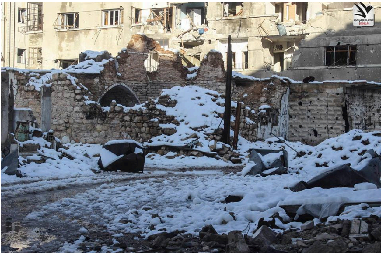
Image showing damage to Great Mosque of Jobar, exterior (APSA)
