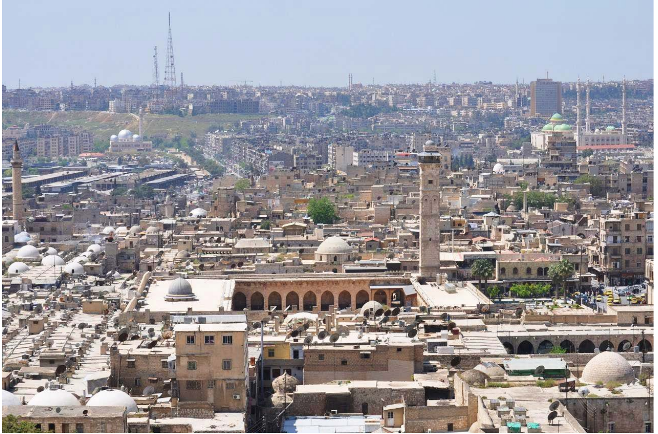
The area damaged by the tunnel bomb (bottom right), photographed from the citadel in 2010 by Brandt Maxwell. ( http://www.geographylists.com/syria_aleppo2.html )
