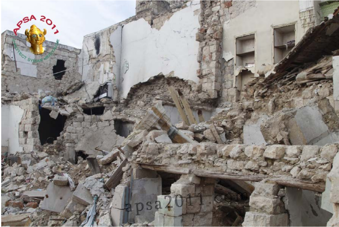
Damage to the Al-Muhtaseb Mosque in Aleppo (APSA)
