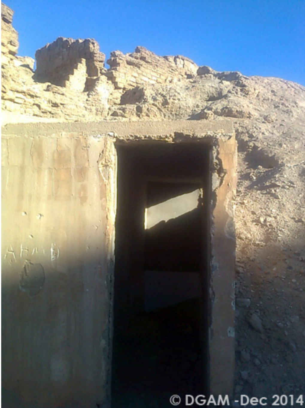
Dura Europos: Illegal excavations and vandalism of the visitor's center (DGAM).
