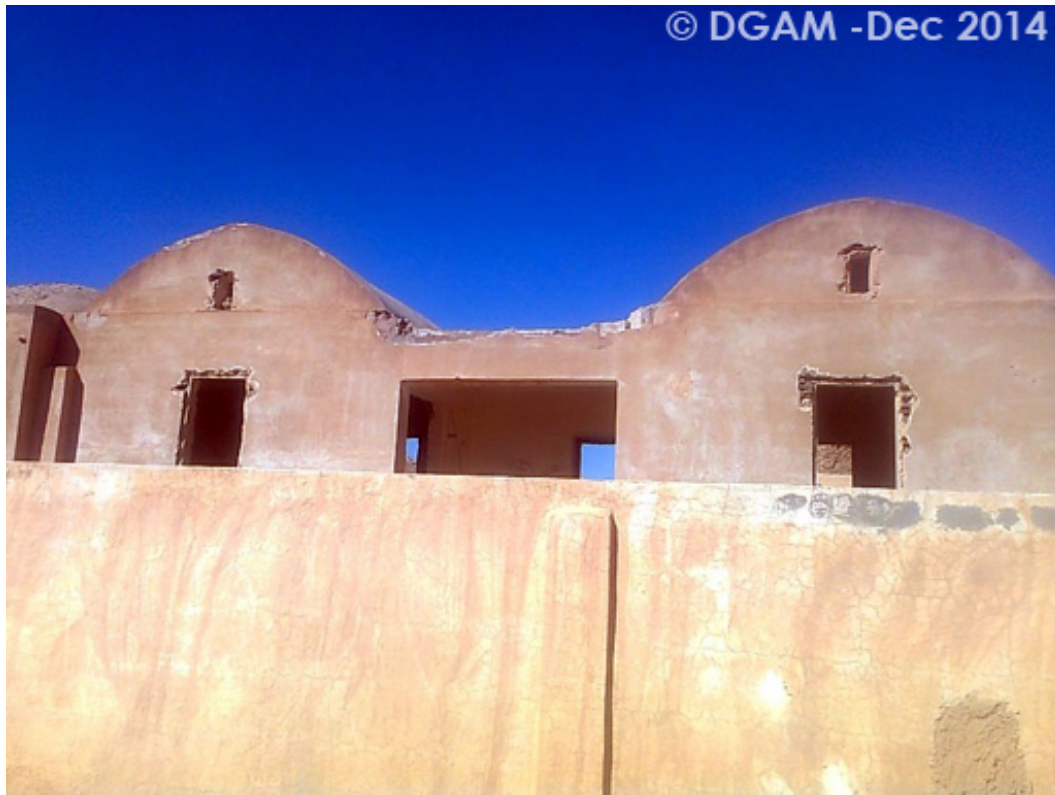
Dura Europos: Illegal excavation and vandalism of the exc. headquarters (DGAM).
