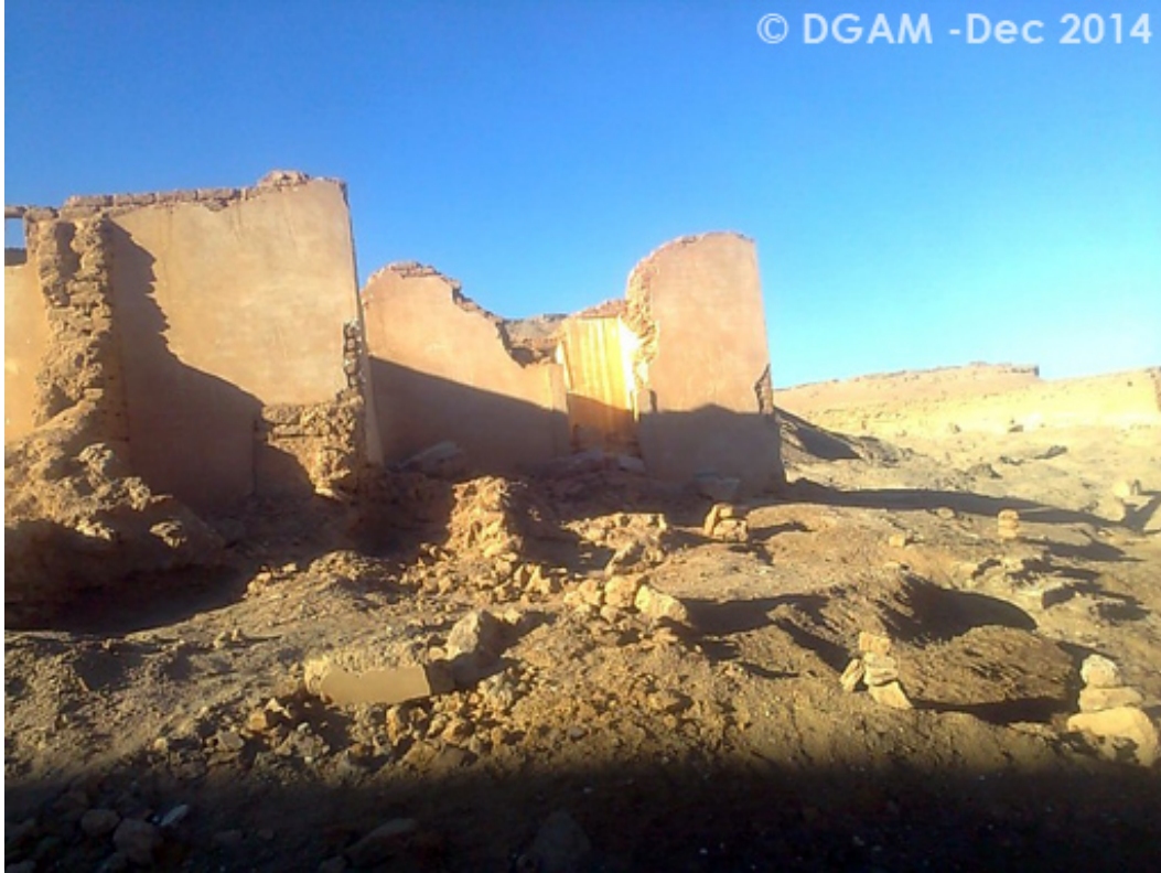
Dura Europos: Illegal excavations and vandalism of the visitor's center (DGAM).
