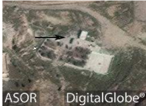
Shrine of Sheikh Nasr al Din post destruction with some of the structure still intact (DigitalGlobe; March 7, 2015)
