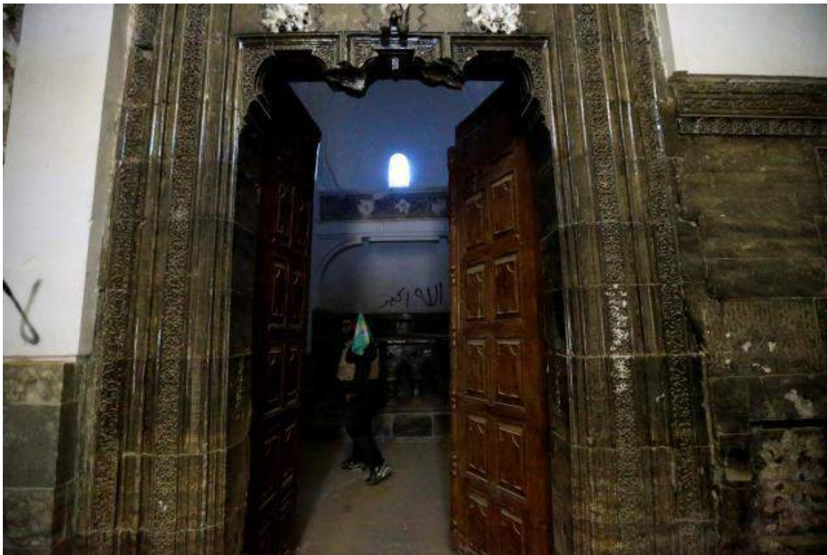
Damage and graffiti on the inside of Mar Behnam Monastery (Reuters; November 21, 2016)
