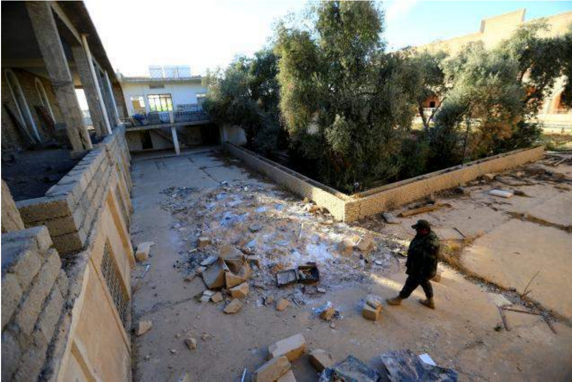
Damage at Mar Behnam Monastery (Reuters; November 21, 2016)
