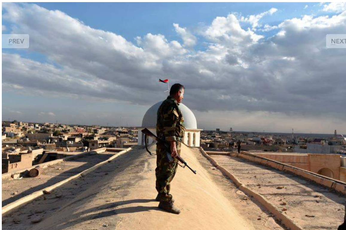
Damage seen on the roof of Mar Yohanna Church (Thomas Goisque; November 20, 2016)
