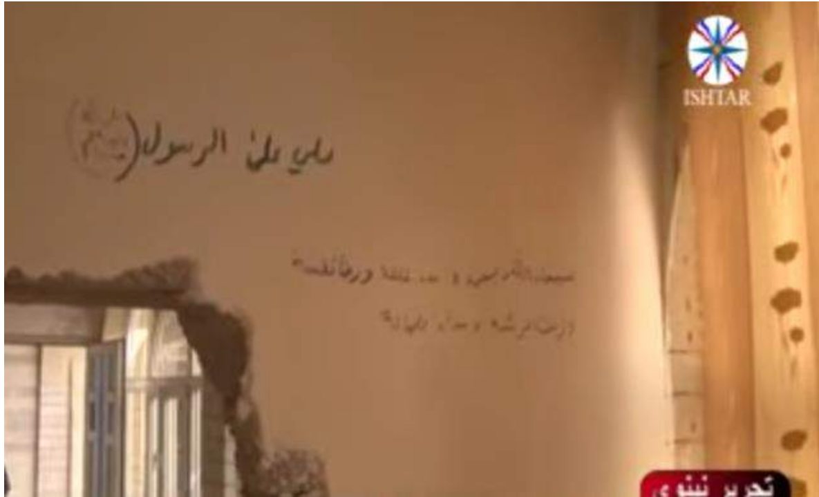
Video still of graffiti inside Mar Gerges Church in Bahzani (Ishtar TV; November 11, 2016)
