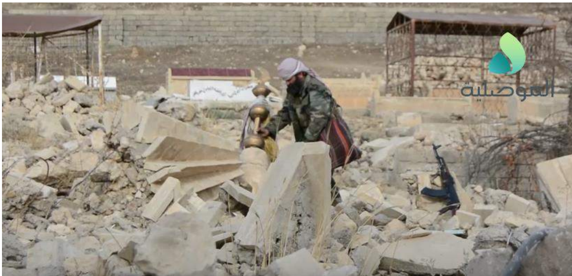
Video still of a Yezidi fighter examining damage to Shrine of Sheikh Babik (Mosul Channel TV; November 11, 2016)
