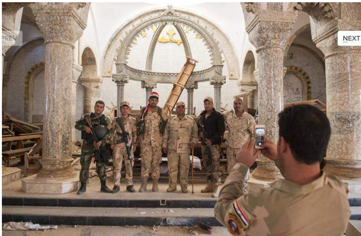
Limited damage to the nave of Mar Yohanna Church (Thomas Goisque; November 20, 2016)
