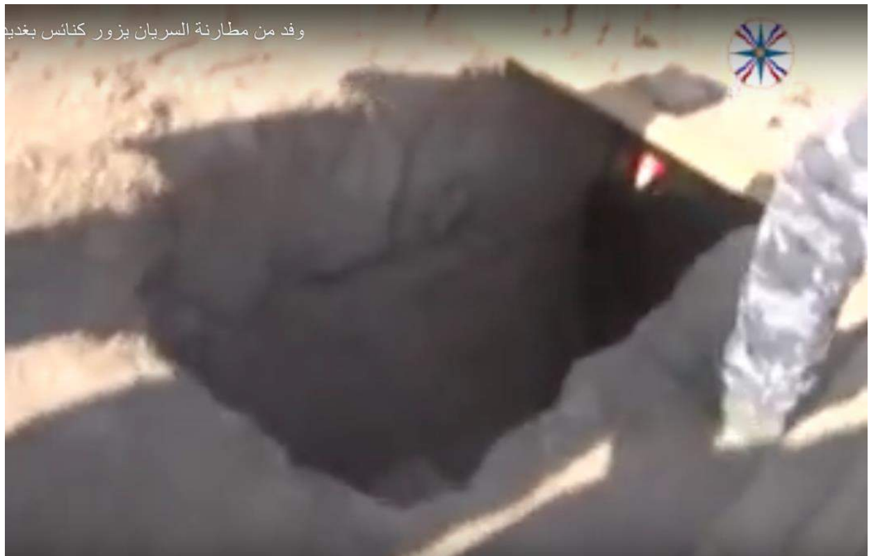
Video still of a tunnel dug inside Mart Shmone Church (IshtarTV; November 23, 2016)
