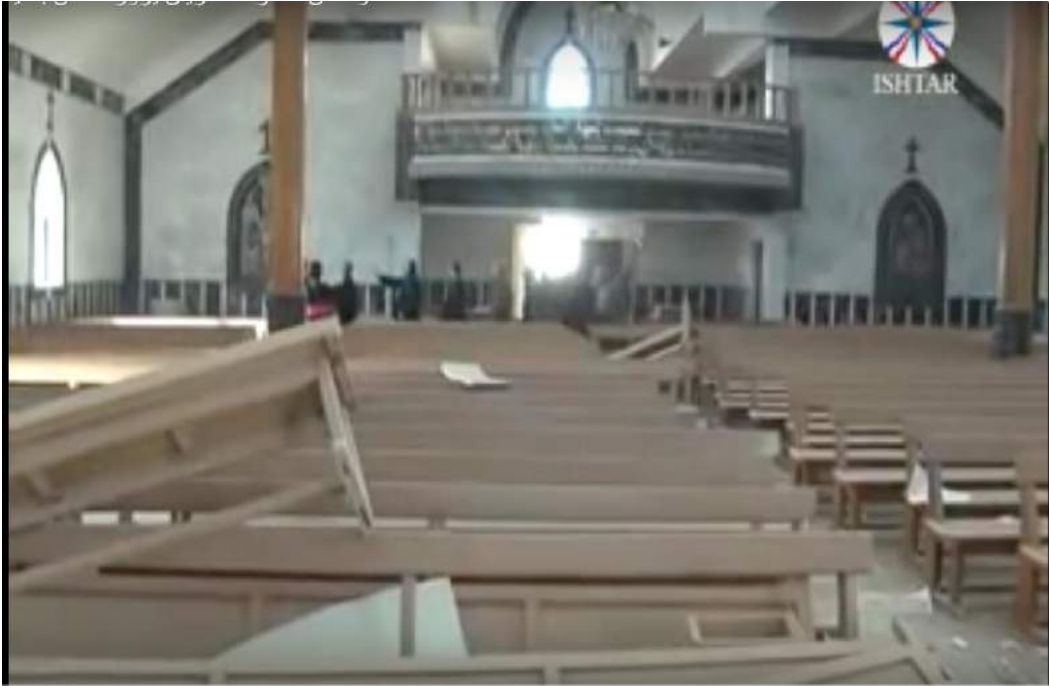
Video still of damage inside of Mar Gerges Church in Bakhdida (IshtarTV; November 23, 2016)
