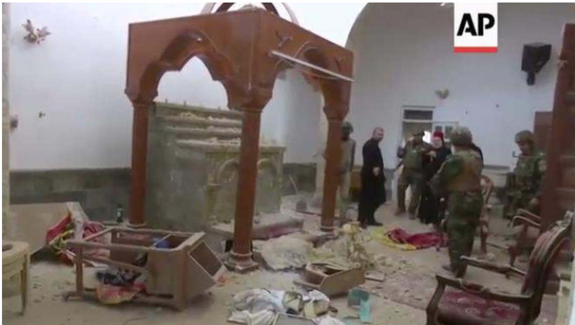
Video still of damage to an altar inside Mart Shmone Church in Bashiq (AP; November 18, 2016)
