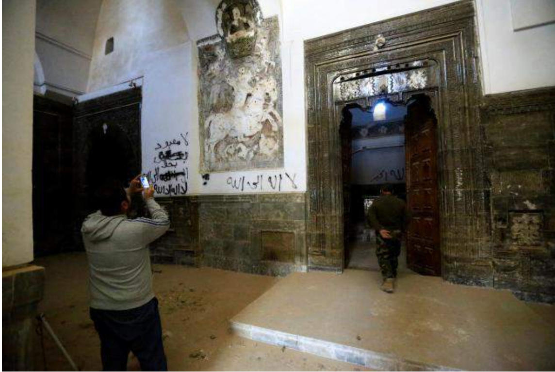
Damage and graffiti on the inside of Mar Behnam Monastery (Reuters; November 21, 2016)
