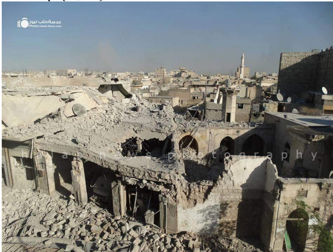
Severe damage to Barsin Mosque (SNHR; November 18, 2016)
