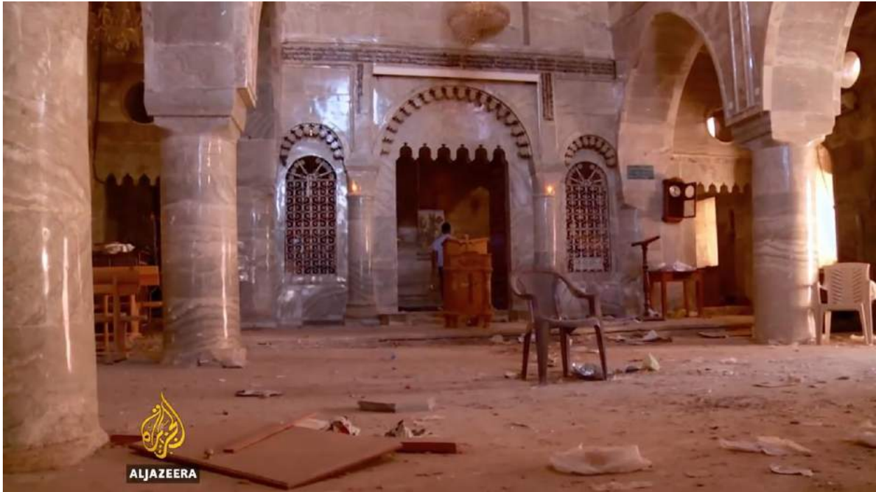
Video still of damage to the interior of Mar Gerges Church (Al Jazeera; November 21, 2016)
