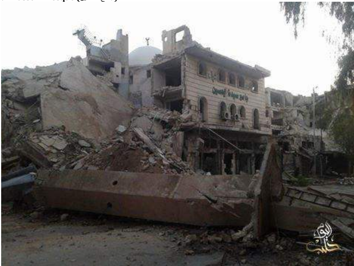
Collapse of the minaret of al-Hussein Mosque (November 17, 2016)
