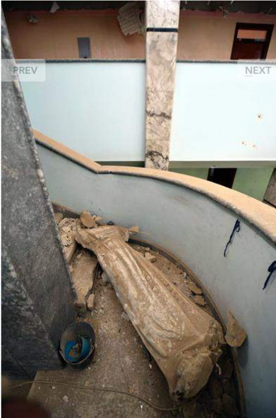
Damage to a statue at Dar Mar Polis Church Services (Thomas Goisque; November 20, 2016)
