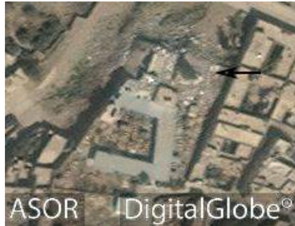
Shrine of Meleke Miran Sadiq post destruction with some of the structure still intact (DigitalGlobe; September 28, 2014)
