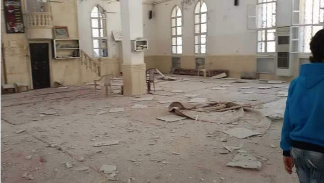
Debris in the interior of al-Hussein Mosque (SNHR; November 20, 2016)
