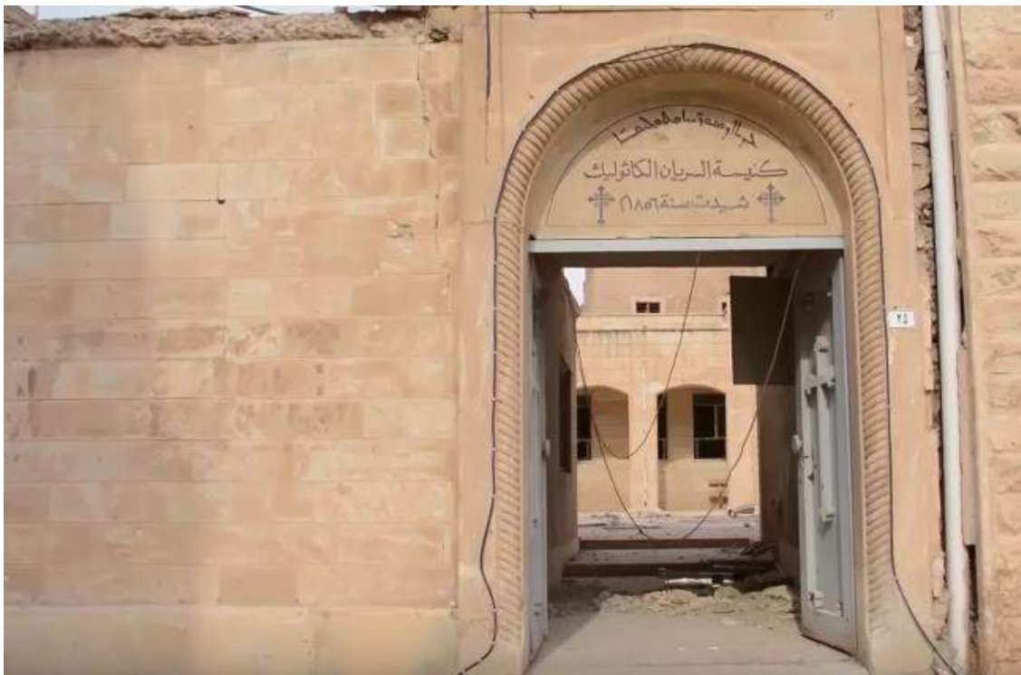
Damage to Mart Mariam Church in Bashiqa (Mosul Channel TV; November 11, 2016)
