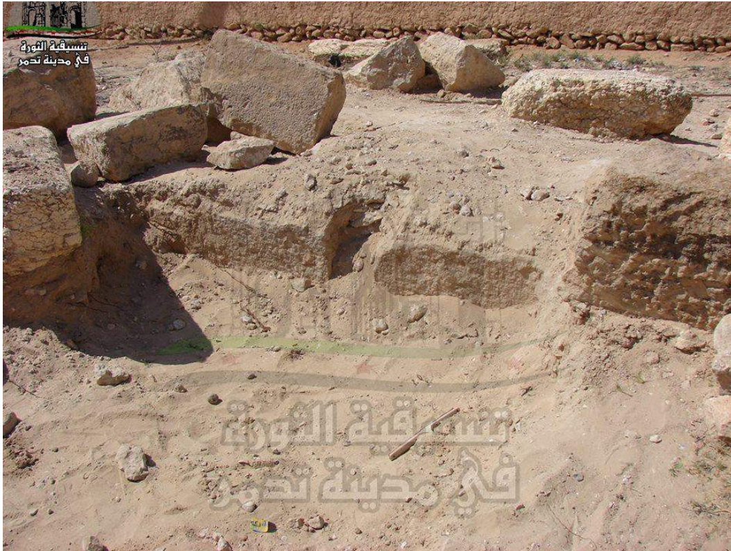
Illegal excavation and damage to a structure at Palmyra (Palmyra Coordination Committee; November 24, 2016)
