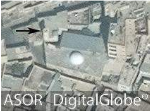
al-Mashatiya Mosque with partial collapse of the minaret visible (DigitalGlobe; October 19, 2016)
