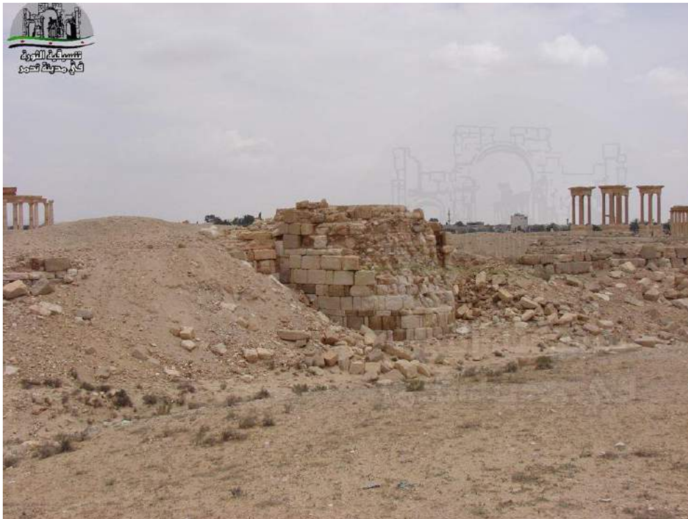
Illegal excavation and damage to a structure at Palmyra (Palmyra Coordination Committee; November 24, 2016)
