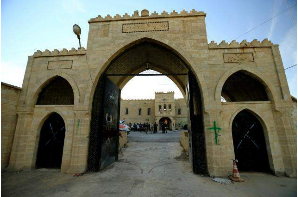
Graffiti and damage to Mar Behnam Monastery (Reuters; November 21, 2016)
