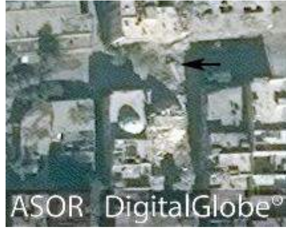
al-Hussein Mosque with collapsed minaret (DigitalGlobe; November 19, 2016)
