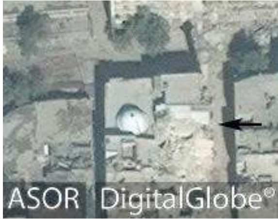
al-Hussein Mosque prior to damage to minaret. Note the previously damaged buildings on the south side (DigitalGlobe; October 19, 2016)
