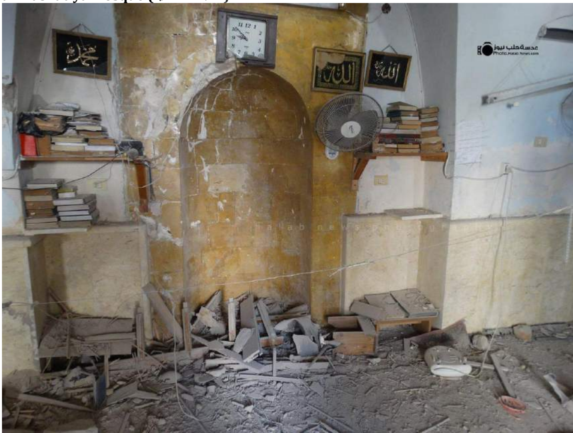
Damage to the interior of al-Mashatiya Mosque (SNHR; November 20, 2016)
