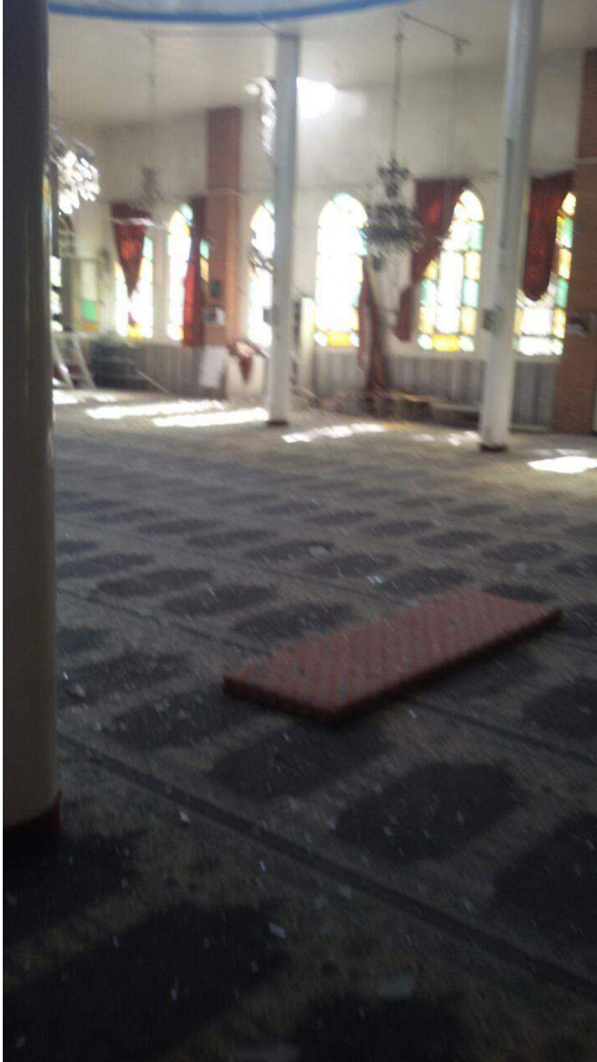
Interior damage to al-Kabir Mosque in Jisreen (SNHR; November 18, 2016)
