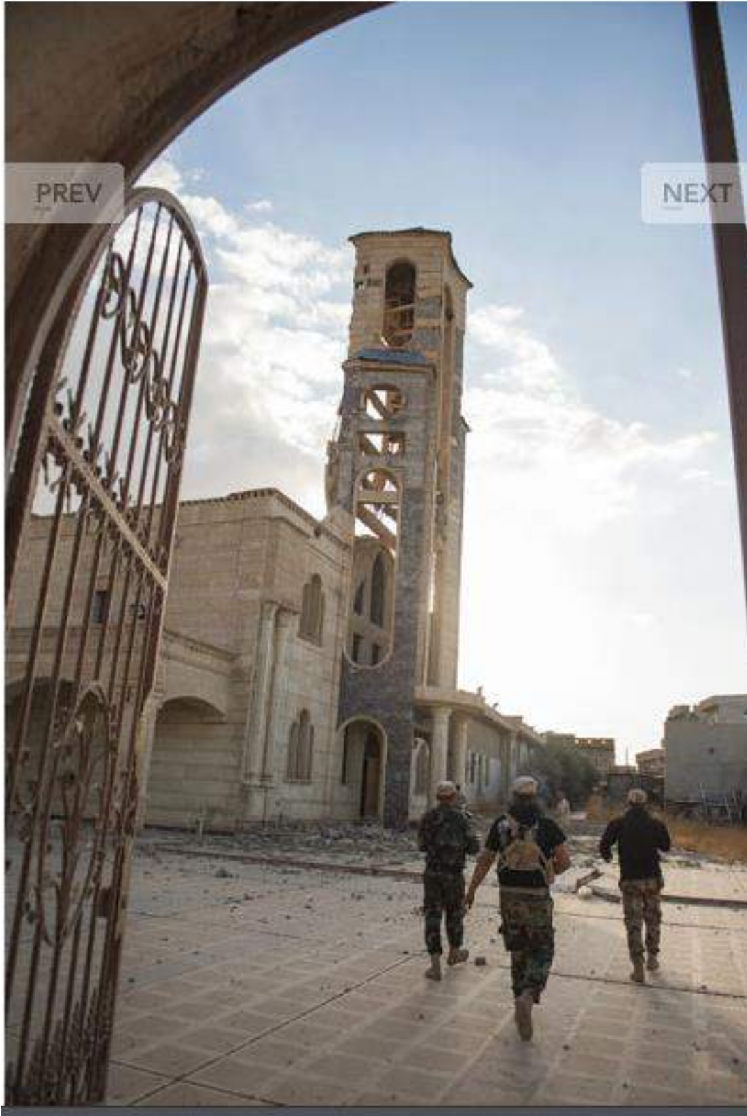
Damage to the front of Mar Yohanna Church and the bell tower (Thomas Goisque; November 20, 2016)
