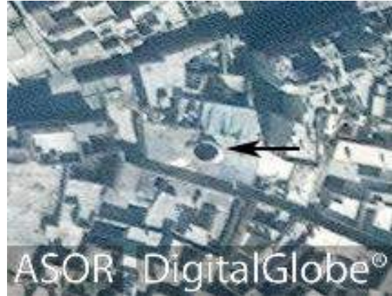
al-Mashatiya Mosque with dome collapsed (DigitalGlobe; November 27, 2016)
