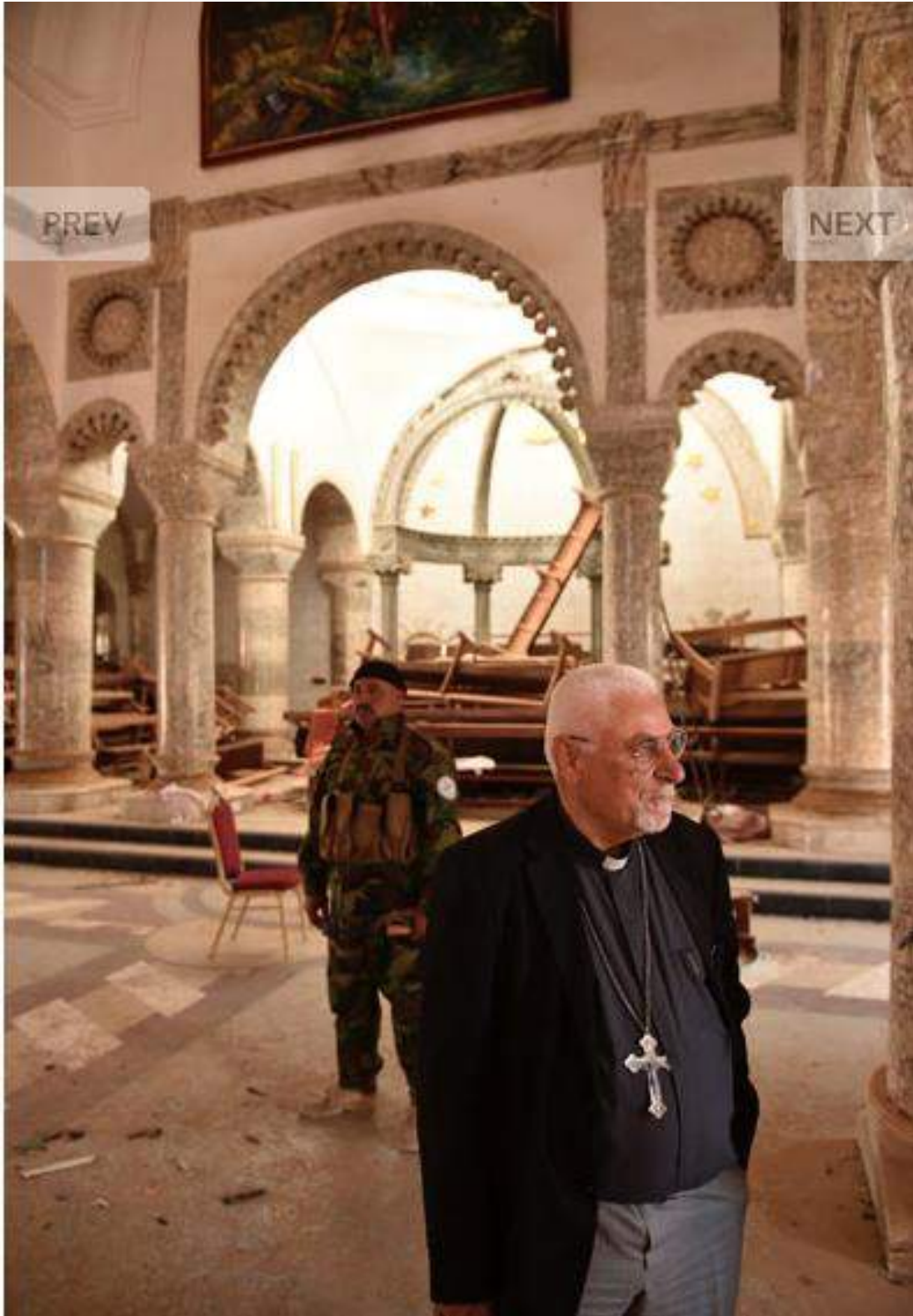
A priest inspects the damage to the inside Mar Yohanna Church (Thomas Goisque; November 20, 2016)
