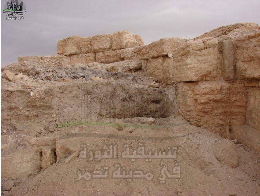
Illegal excavation and damage to a structure at Palmyra (Palmyra Coordination Committee; November 24, 2016)
