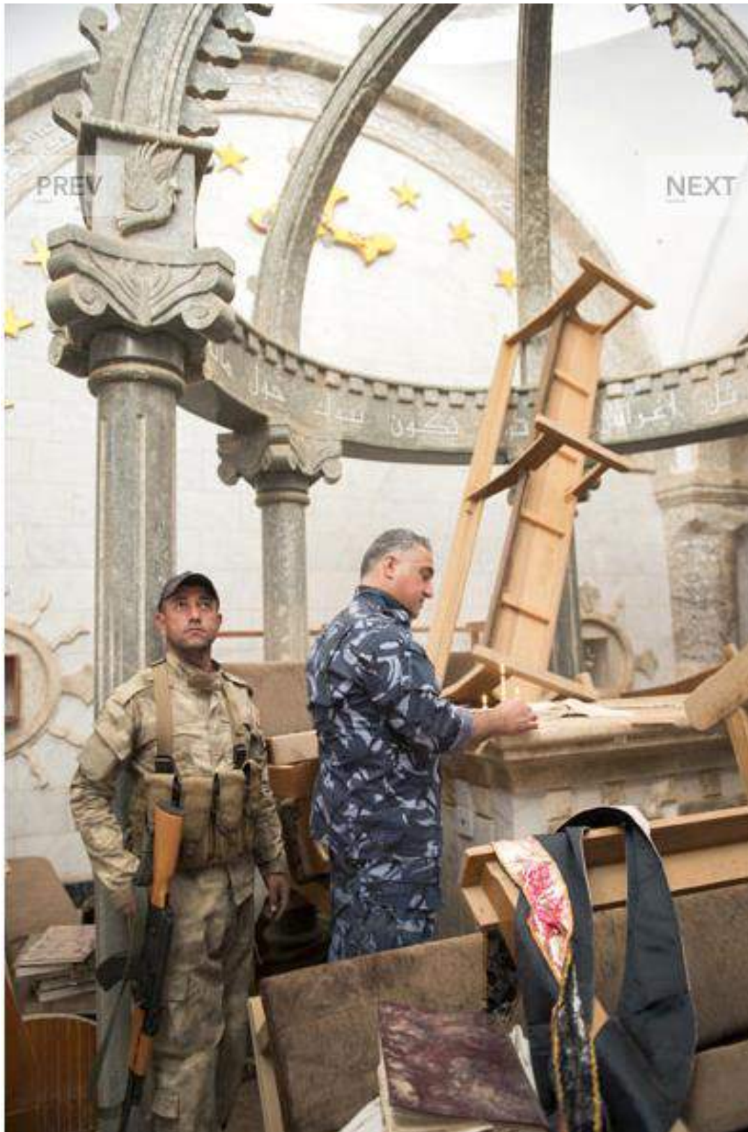
Damage to the inside of Mar Yohanna Church (Thomas Goisque; November 20, 2016)
