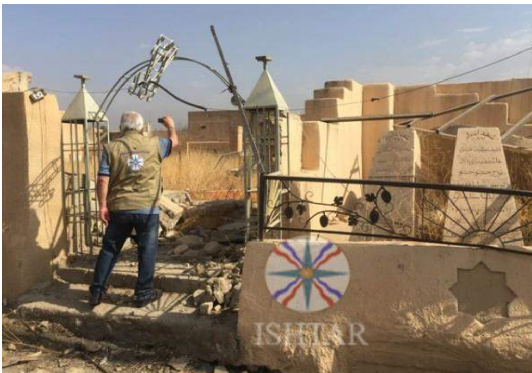
Damage to a gate at Mar George Church (Ishtar TV; October 31, 2016)
