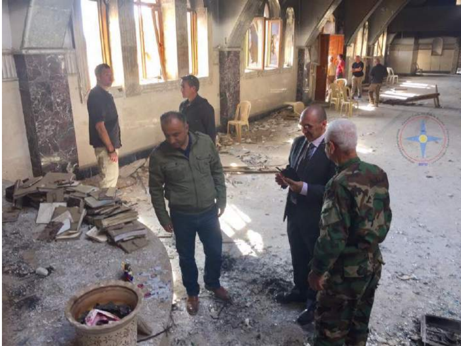
Members of the French Consulate in Erbil tour the damage inside the Church of Saints Behnam and Sarah (NPU; November 14, 2016)
