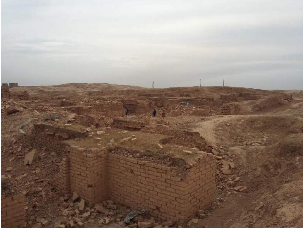
Damage to Northwest Palace at Nimrud (Courtesy of Max Delaney, AFP; November 15, 2016)
