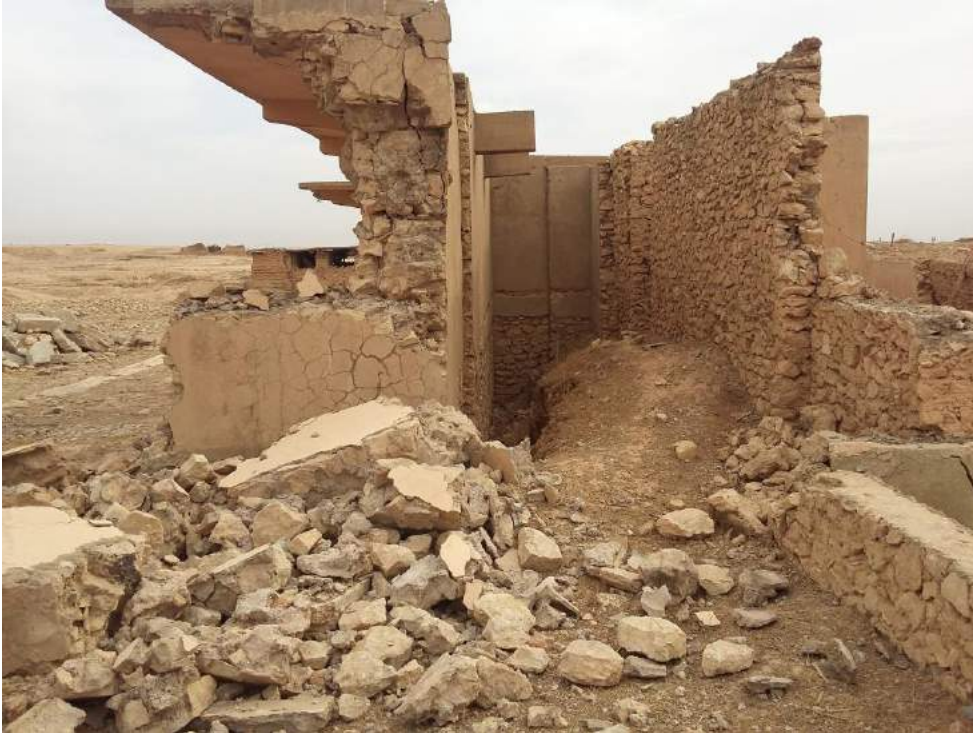
Gate D wall looking towards shrine (Courtesy of Max Delaney, AFP; November 15, 2016)
