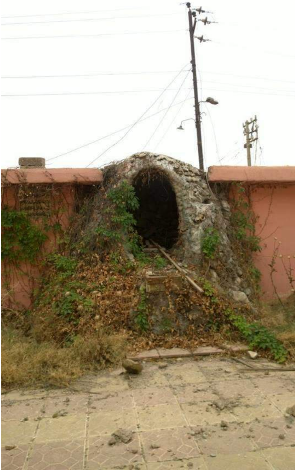
The exterior Mar Ada al-Rasool Church where a statue had been removed (Karamlesh; October 28, 2016)
