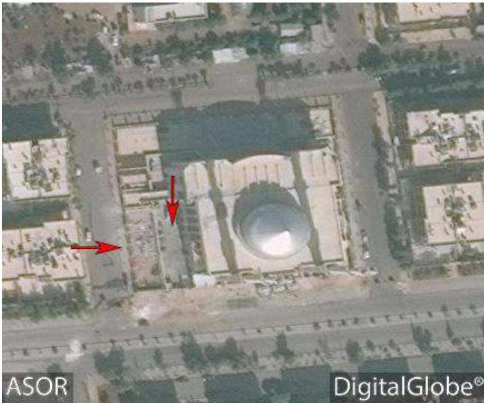
Zain al-Abideen Mosque with visible damage to the western courtyard noted with the red arrows (DigitalGlobe; November 8, 2016)
