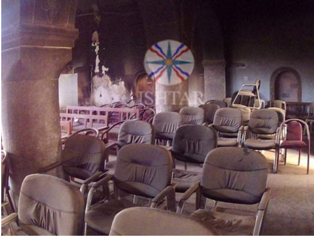
Damage to the interior of the Virgin Mary Church (Ishtar TV; October 31, 2016)
