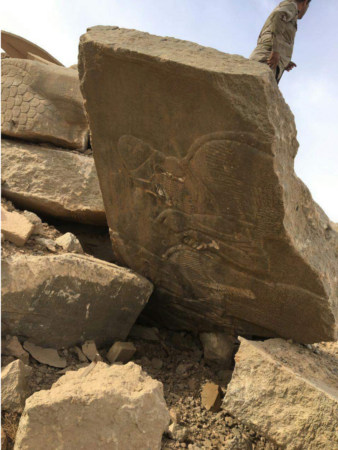
Damage to stone reliefs at Nimrud from the Northwest Palace (Al Harith Al Shwely; November 15, 2016)
