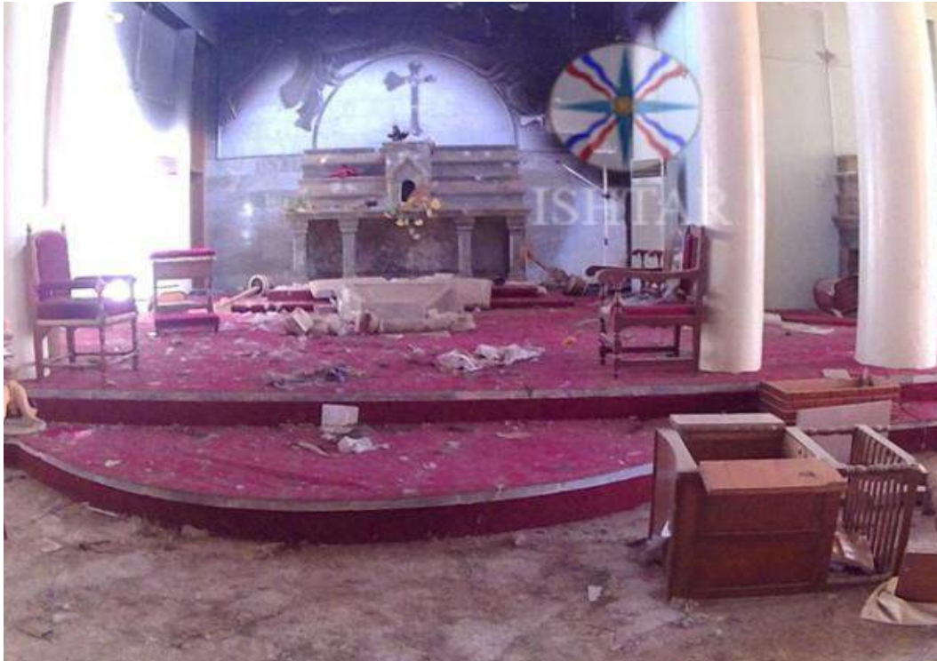
Detail of damage to Mar Ada al-Rasool Church (Ishtar TV; October 31, 2016)
