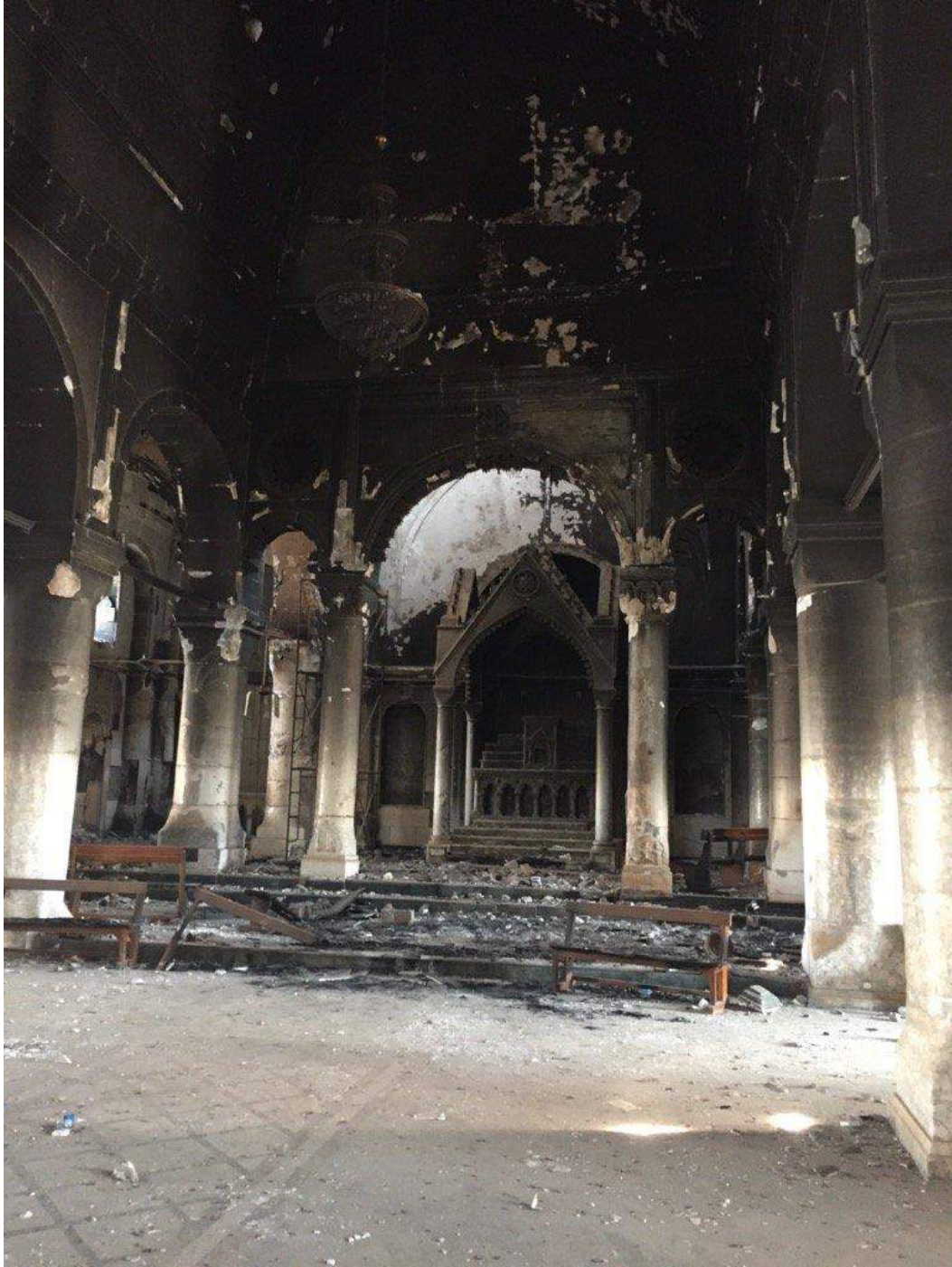
Damage to the interior of the al-Tahira Church (Twitter; October 25, 2016)
