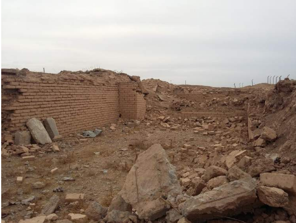
Damage to Northwest Palace (Courtesy of Max Delaney, AFP; November 15, 2016)
