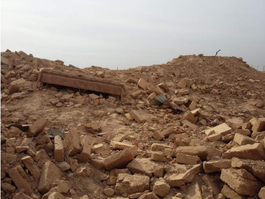
Damage to the Northwest Palace at Nimrud (Courtesy of Max Delaney, AFP; November 15, 2016)
