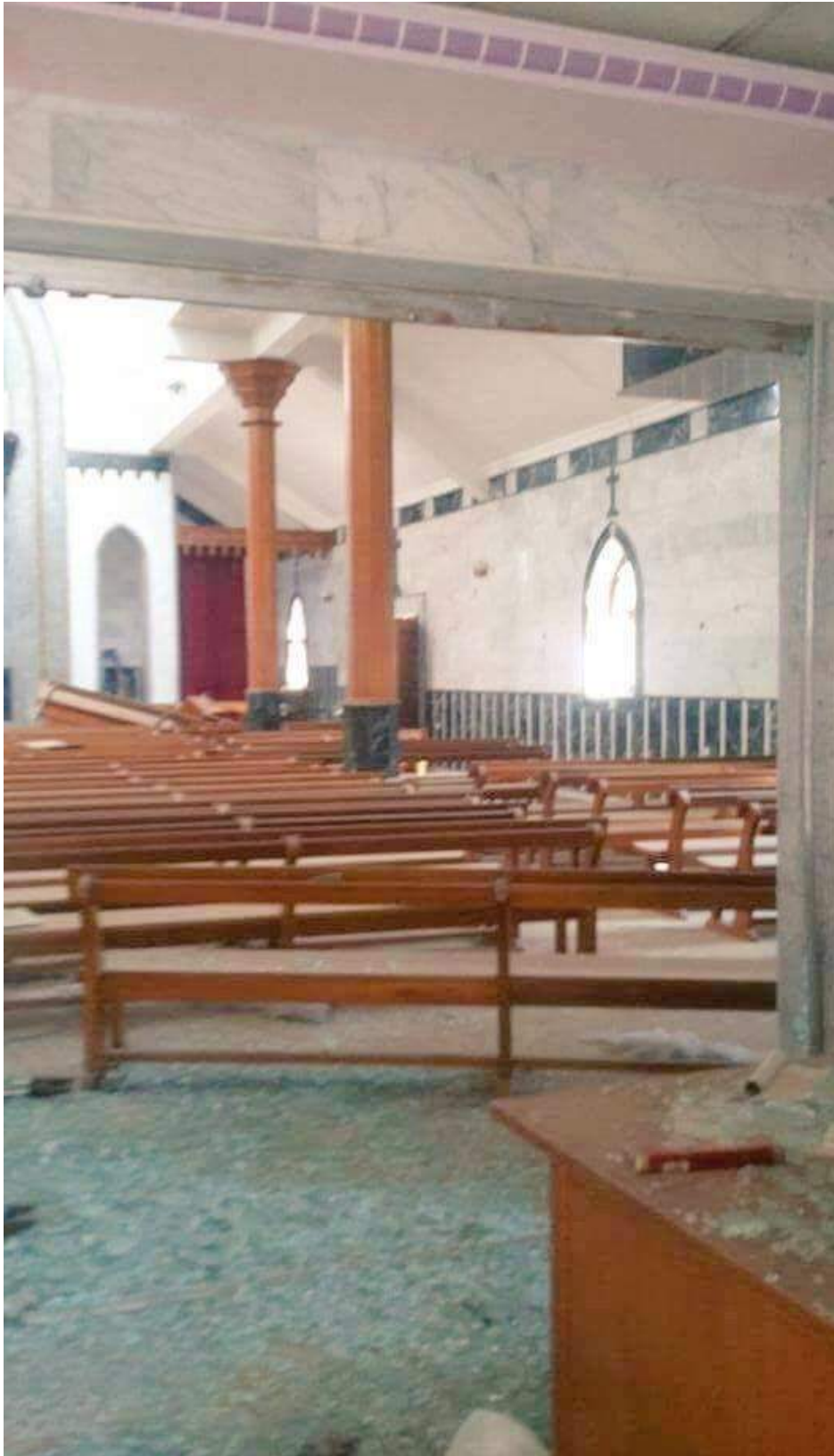
Damage to Mar Gerges Church (Christian of Iraq; October 28, 2016)
