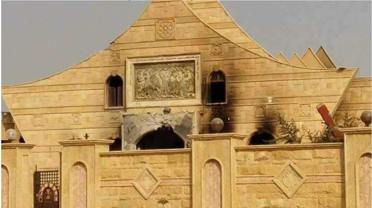
Damage to the Church of Saints Behnam and Sarah (Twitter; October 28, 2016)
