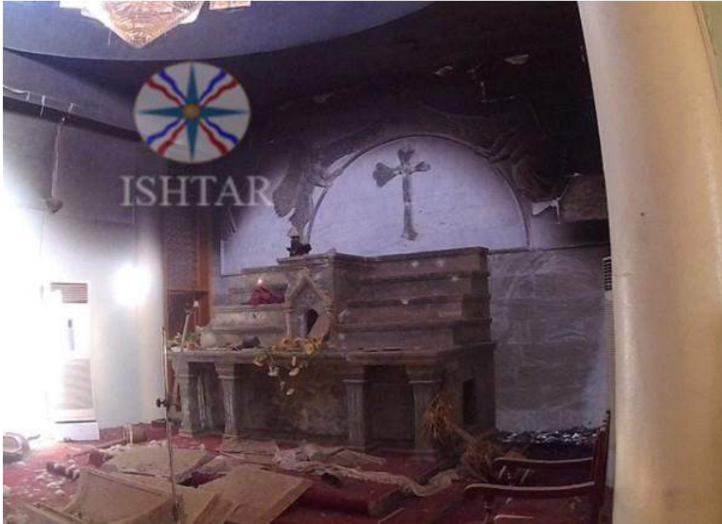
Detail of damage to Mar Ada al-Rasool Church (Ishtar TV; October 31, 2016)
