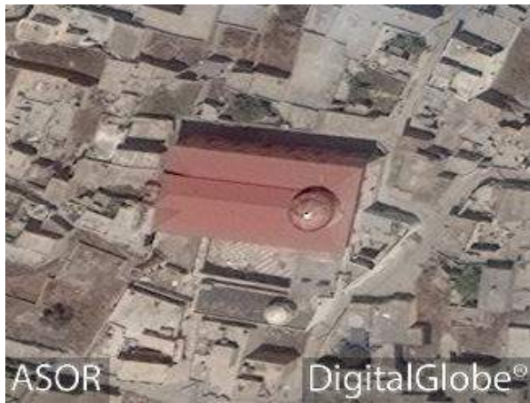
Mar Qoryaqos Church with roof still intact (DigitalGlobe; May 21, 2016)
