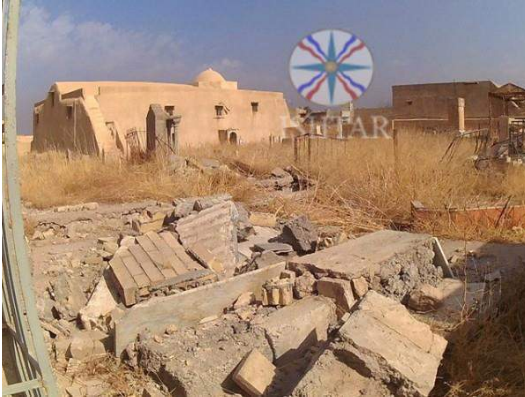
Damage surrounding Mar George Church (Ishtar TV; October 31, 2016)
