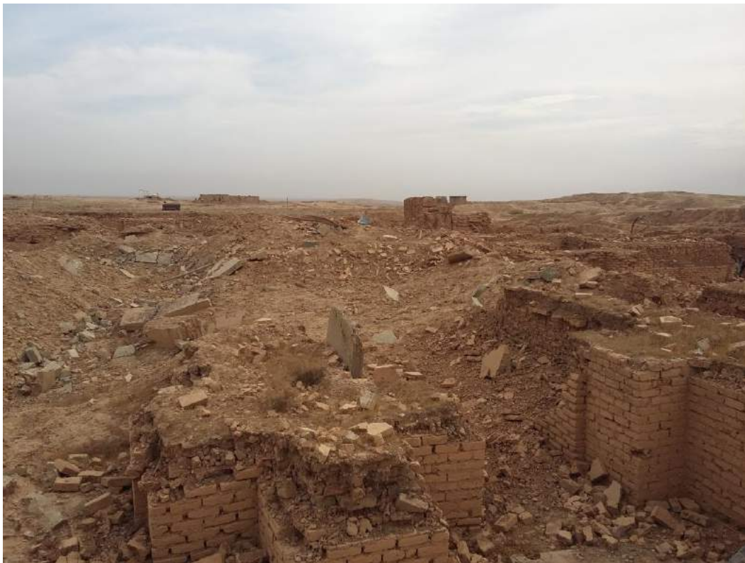
Damage to Northwest Palace at Nimrud (Courtesy of Max Delaney, AFP; November 15, 2016)
