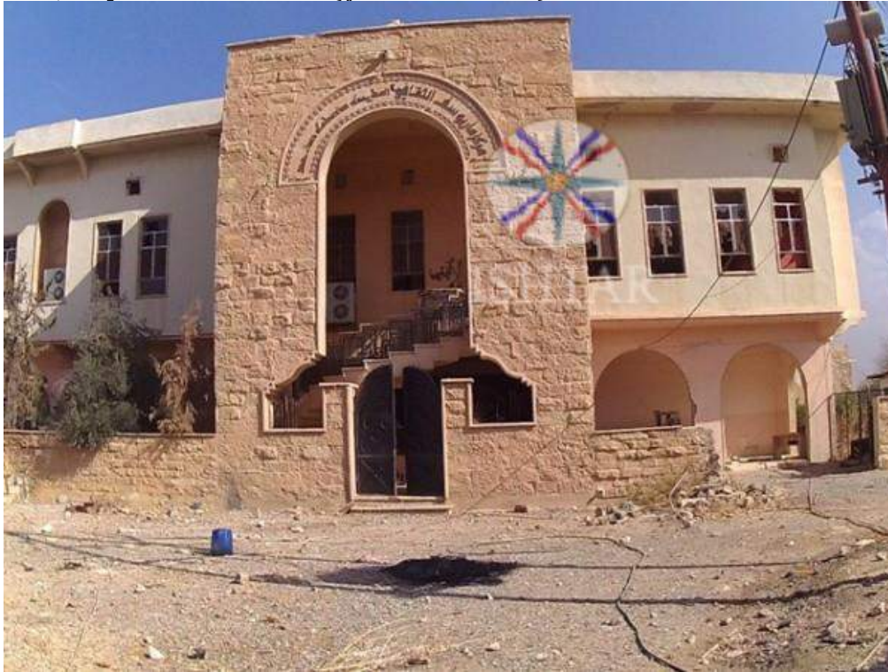
Damage to Mar Joseph Cultural Center (Ishtar TV; October 31, 2016)
