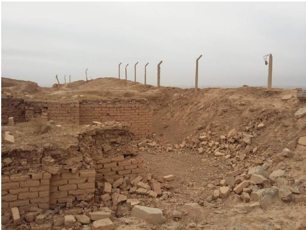
Damage to Northwest Palace at Nimrud (Courtesy of Max Delaney, AFP; November 15, 2016)
