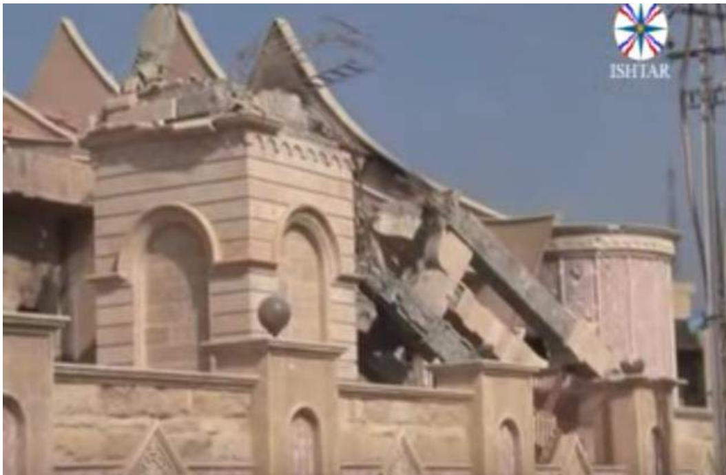
Video still of the fallen tower at the Church of Saints Behnam and Sarah (Ishtar TV; October 31, 2016)
