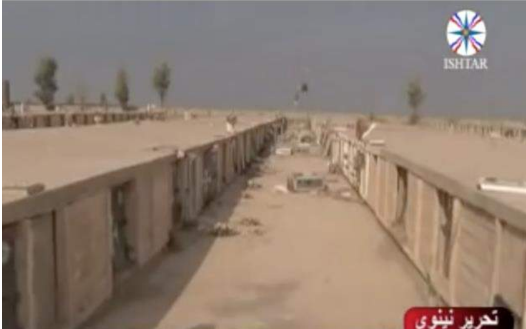
Video still of damage at Resurrection Cemetery (Ishtar TV; November 8, 2016)
