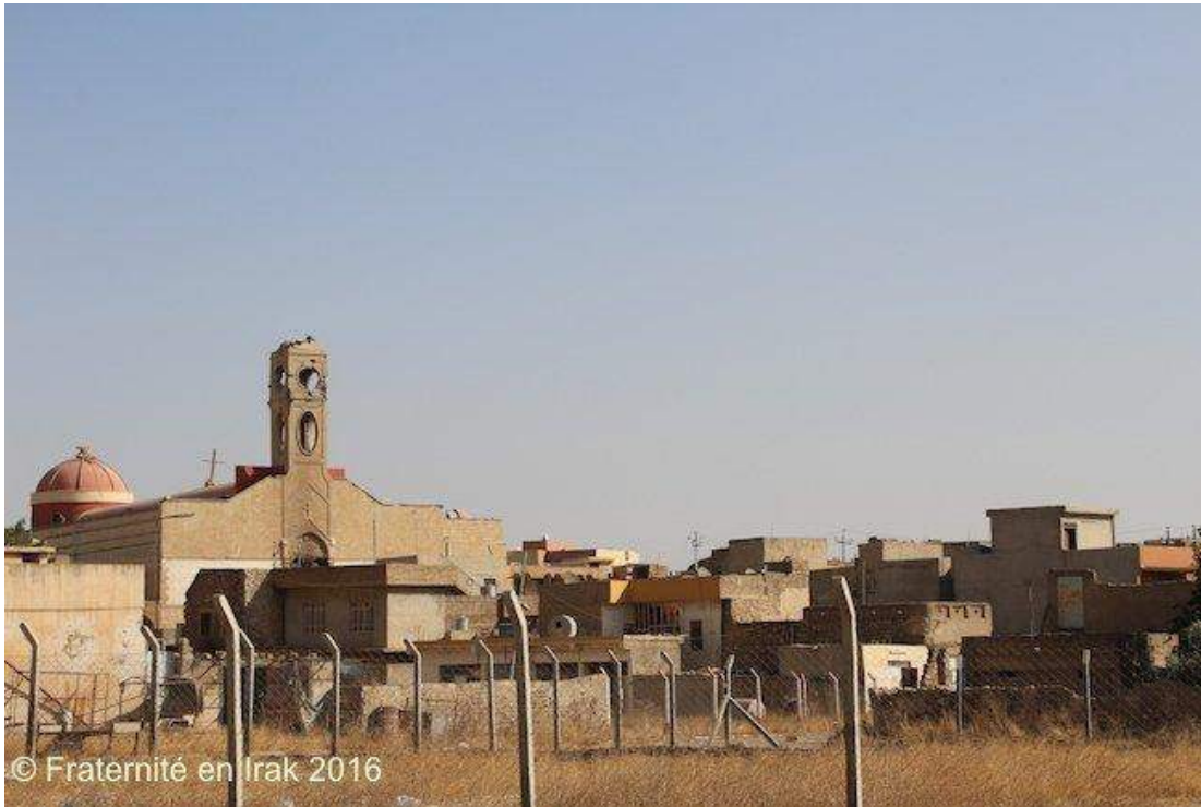
Damage to al-Tahira Church (Fraternité en Irak; November 4, 2016)
