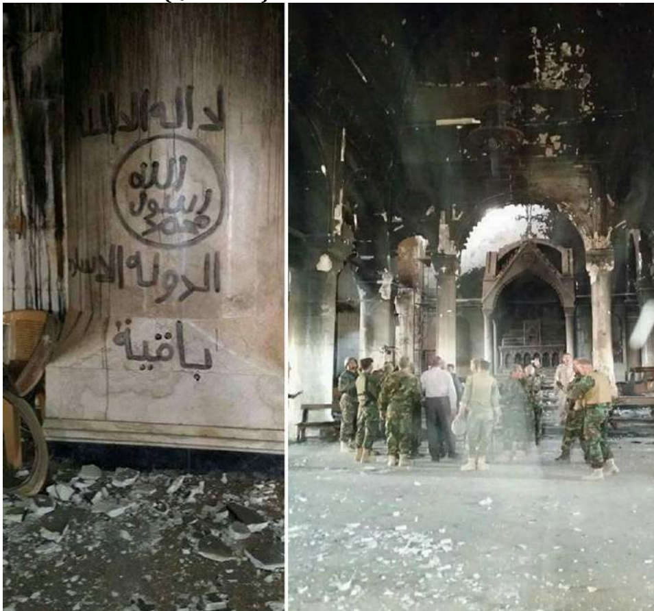
Damage to the al-Tahira Church (Twitter; October 24, 2016)
