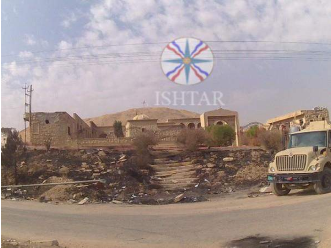
Damage to the area surrounding Mar Barbara Church (Ishtar TV; October 31, 2016)
