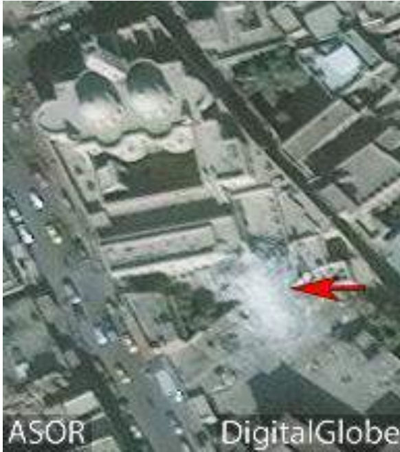
No change to the damaged area of the church (DigitalGlobe; November 12, 2016)
