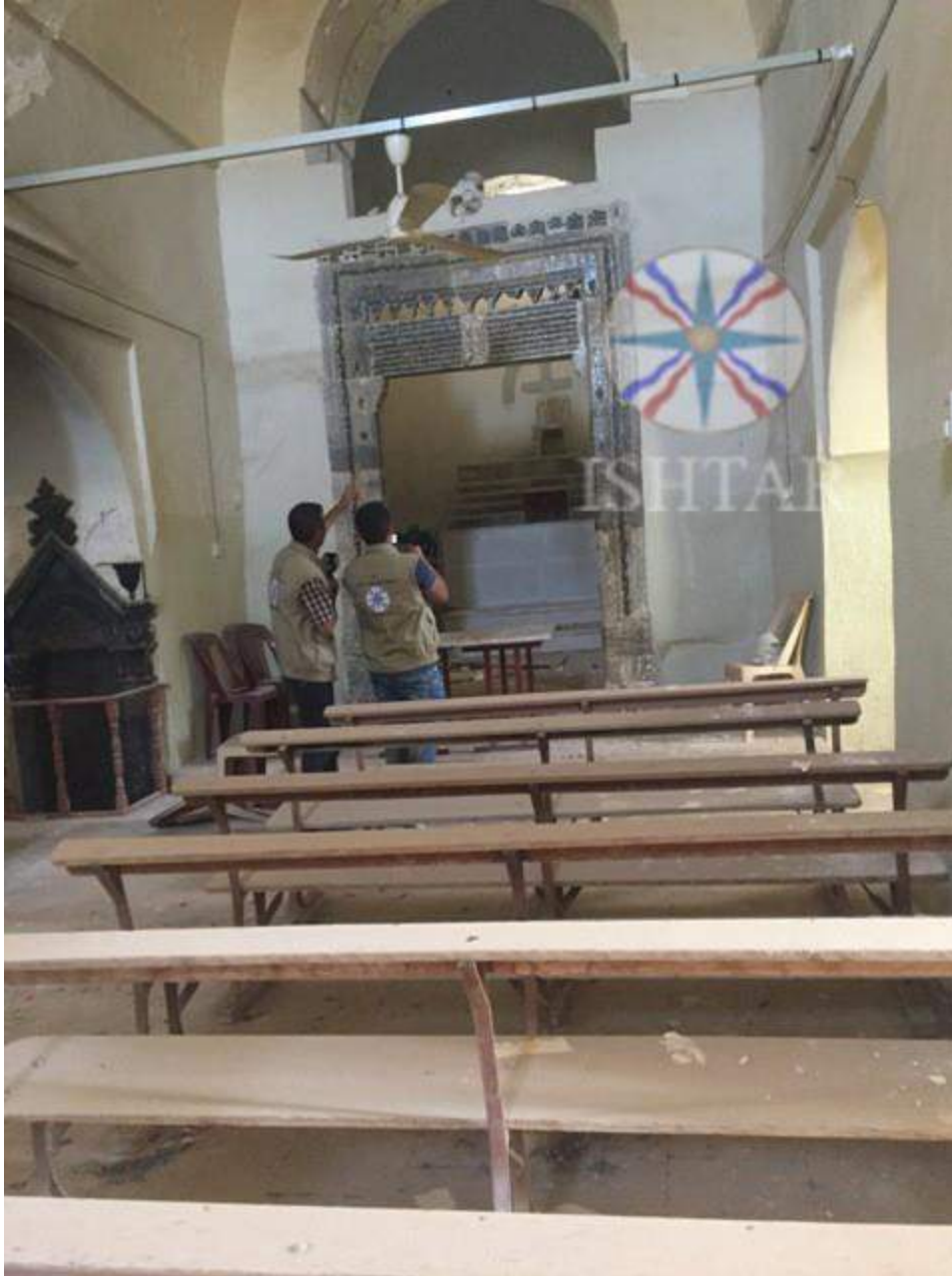
Damage to the interior of Mar George Church (Ishtar TV; October 31, 2016)
