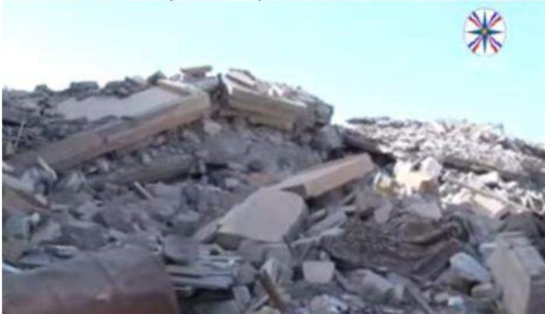
Video still of the complete destruction of Deir Mar Banat (Ishtar TV; October 31, 2016)
