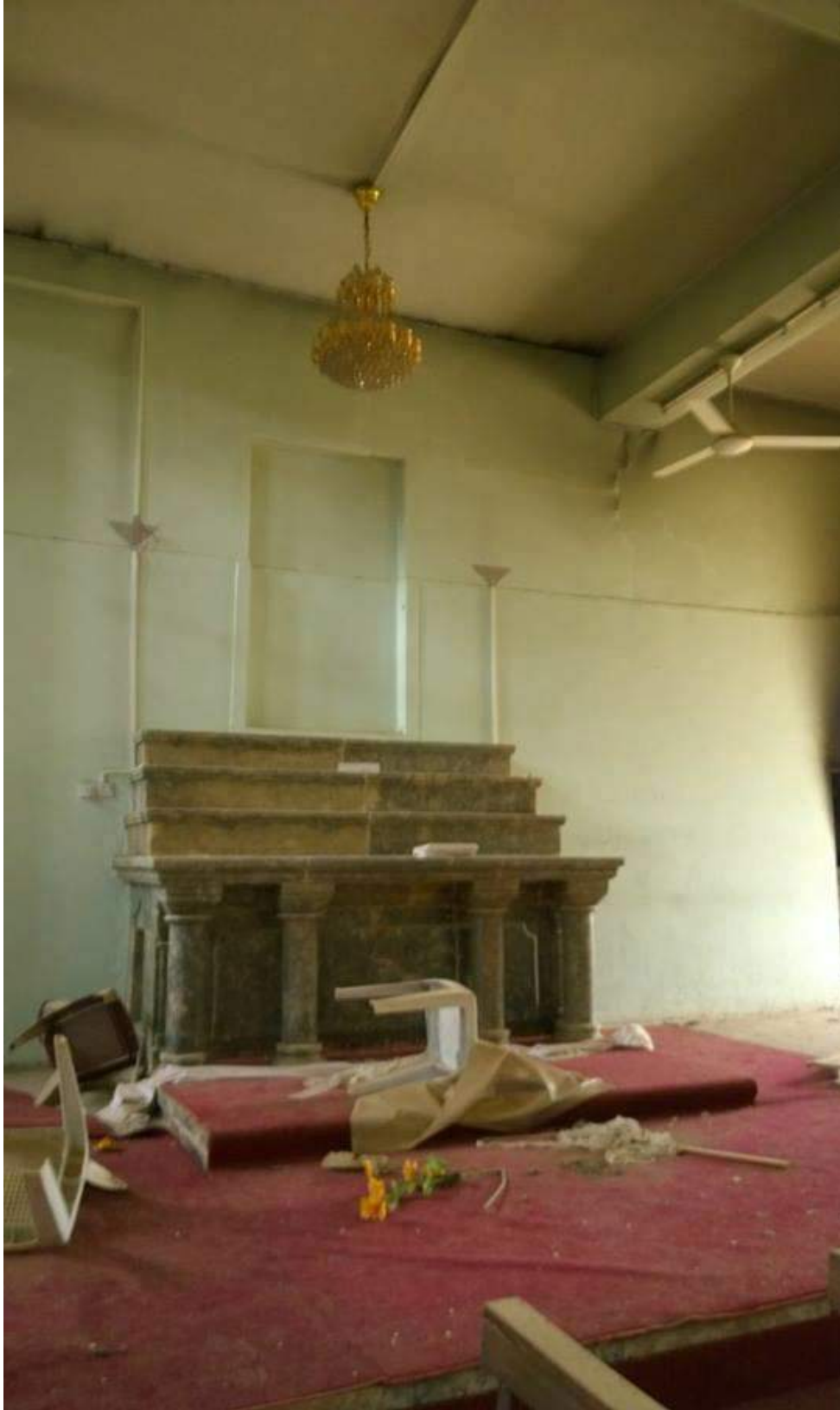
Damage to Mar Ada al-Rasool Church (Karamlesh; October 28, 2016)
