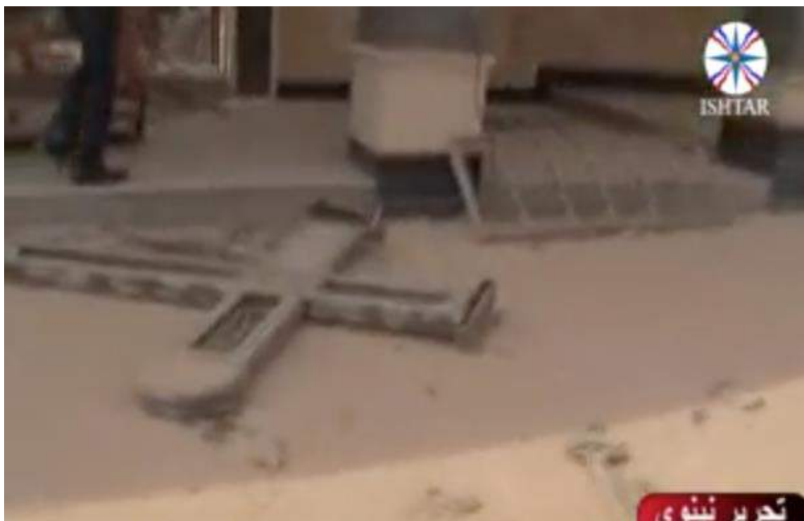
Video still of a fallen cross at the entrance to the Church of the Resurrection (Ishtar TV; November 8, 2016)
