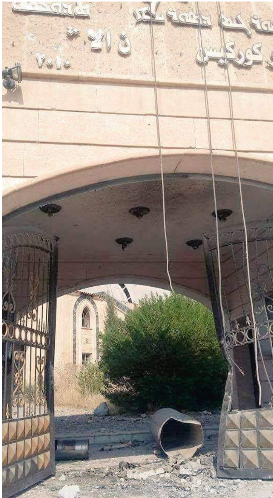
Damage to Mar Gerges Church (Christian of Iraq; October 28, 2016)
