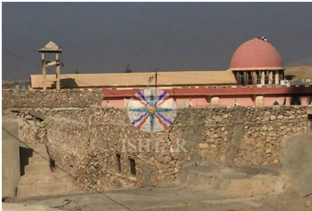
Exterior damage to Mar Ada al-Rasool Church (Ishtar TV; October 31, 2016)
