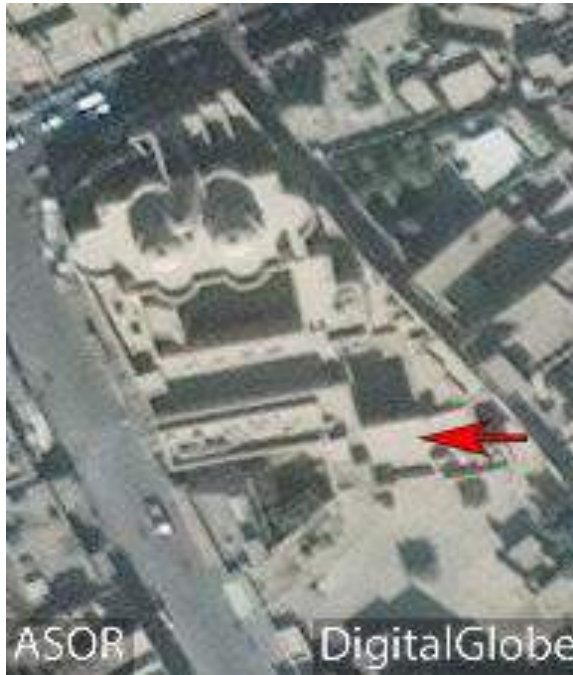
Church prior to damage (DigitalGlobe; October 21, 2016)
