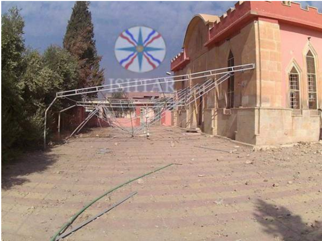
Damage to exterior of Mar Ada al-Rasool Church (Ishtar TV; October 31, 2016)
