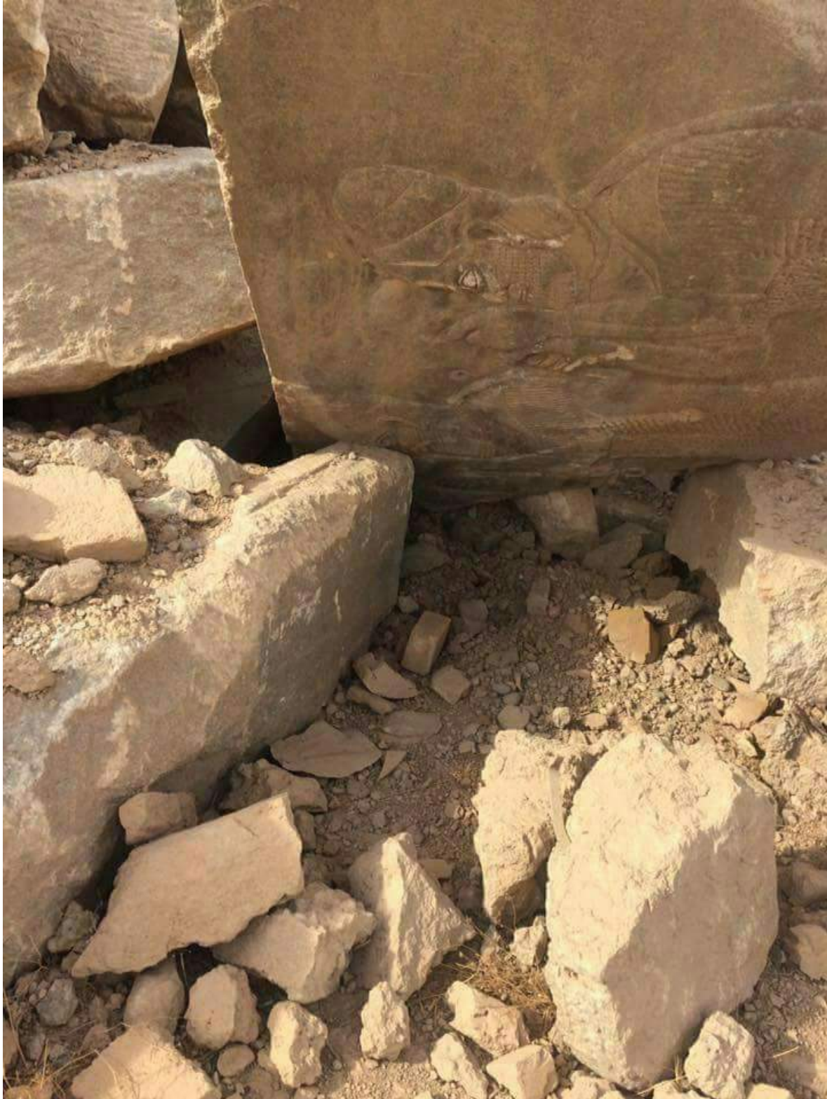
Damage to stone reliefs at Nimrud from the Northwest Palace (Al Harith Al Shwely; November 15, 2016)
