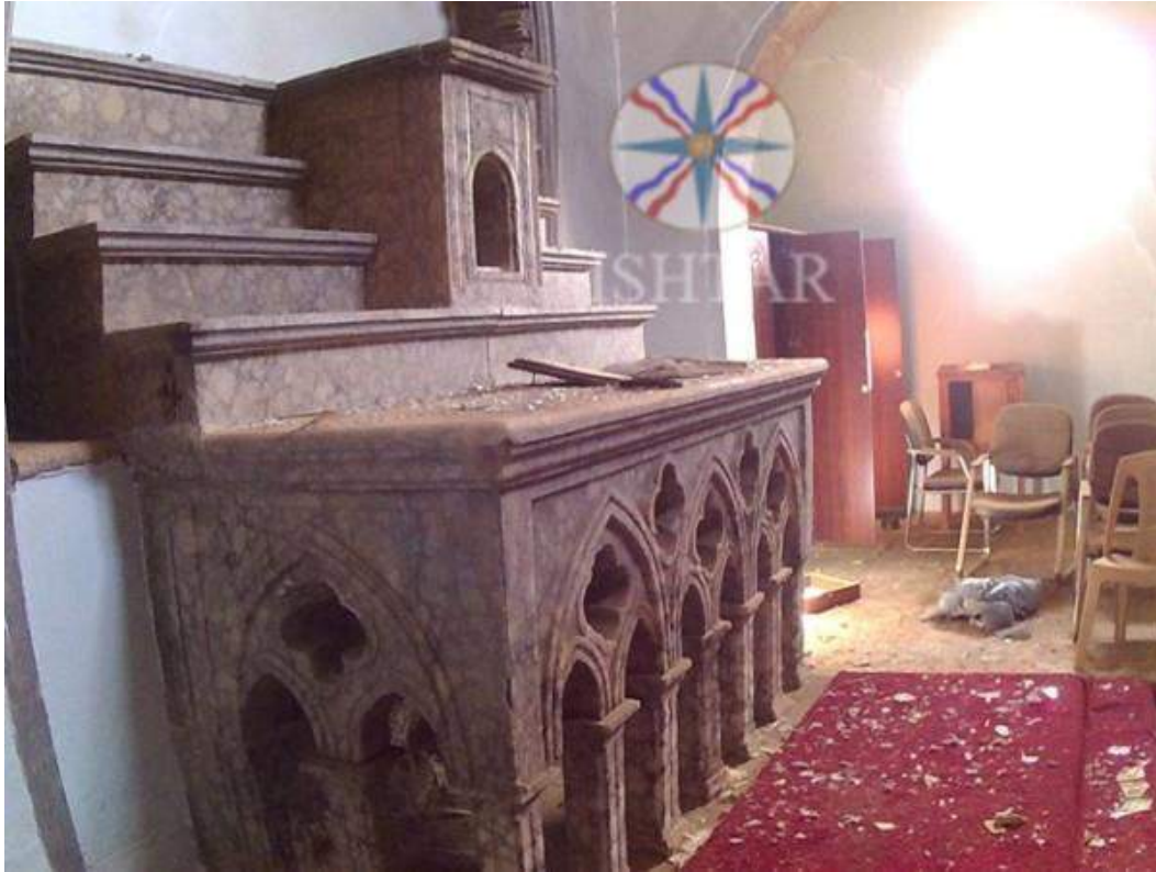
Damage to the interior of the Virgin Mary Church (Ishtar TV; October 31, 2016)
