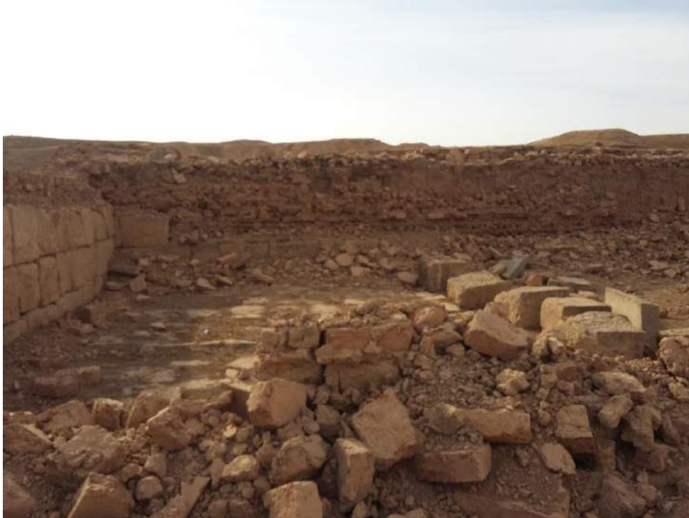
Nabu Temple at Nimrud showing debris in the courtyard (Courtesy of Max Delaney, AFP; November 15, 2016)
