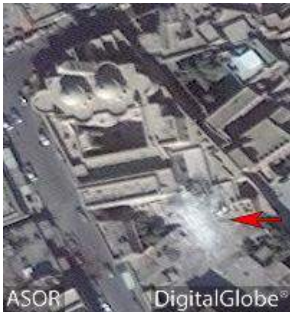
Southern part of the church damaged (DigitalGlobe; November 4, 2016)
