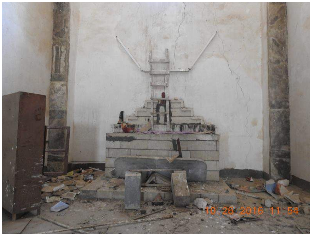
Damage to Mar Oraha Monastery (Twitter; October 26, 2016)
