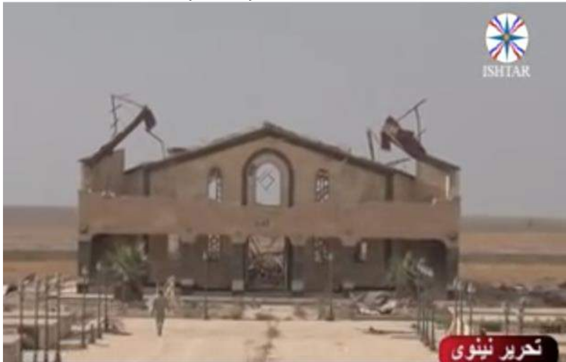
Video still of damage to the Church of the Resurrection (Ishtar TV; November 8, 2016)
