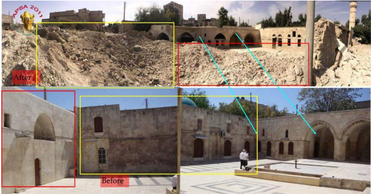
Severe damage to courtyard of al-Tawba Mosque, facing northwest (APSA; October 6, 2016)
