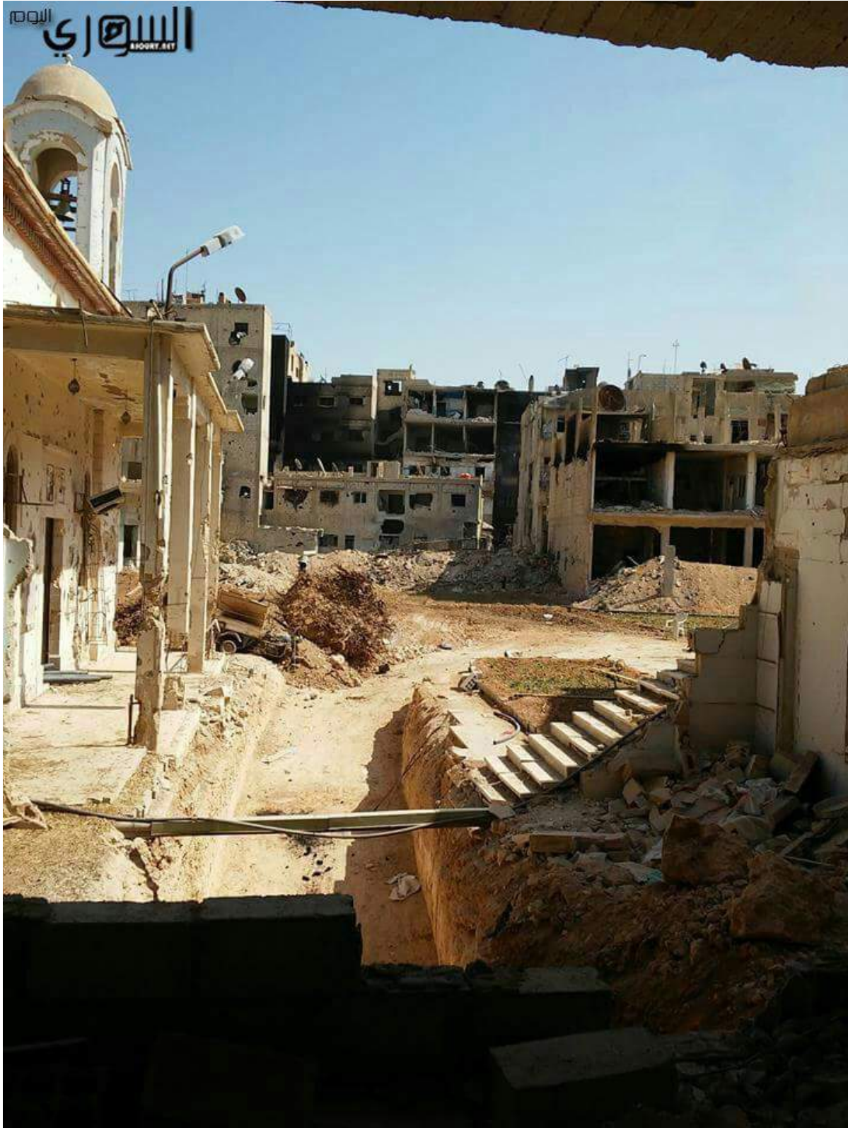
Damage to the exterior and surrounding area of Saint Paul the Apostle Church (ASoury; September 5, 2016)
