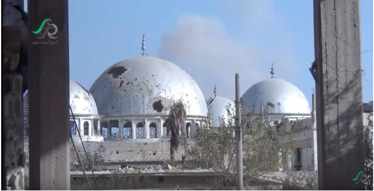
Damage to al-Nur Mosque domes (Syria Rebels Gathering; September 21, 2016)
