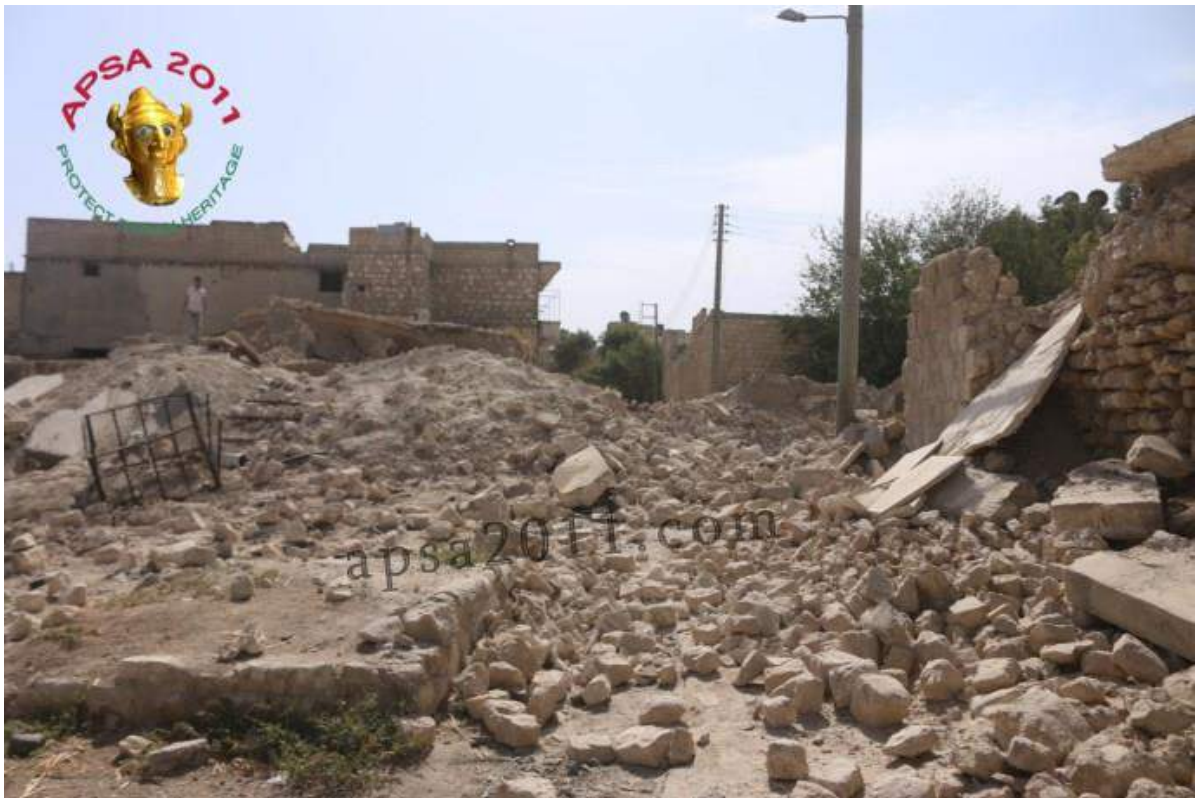
Severe damage to eastern wall of al-Tawba Mosque (APSA; October 6, 2016)
