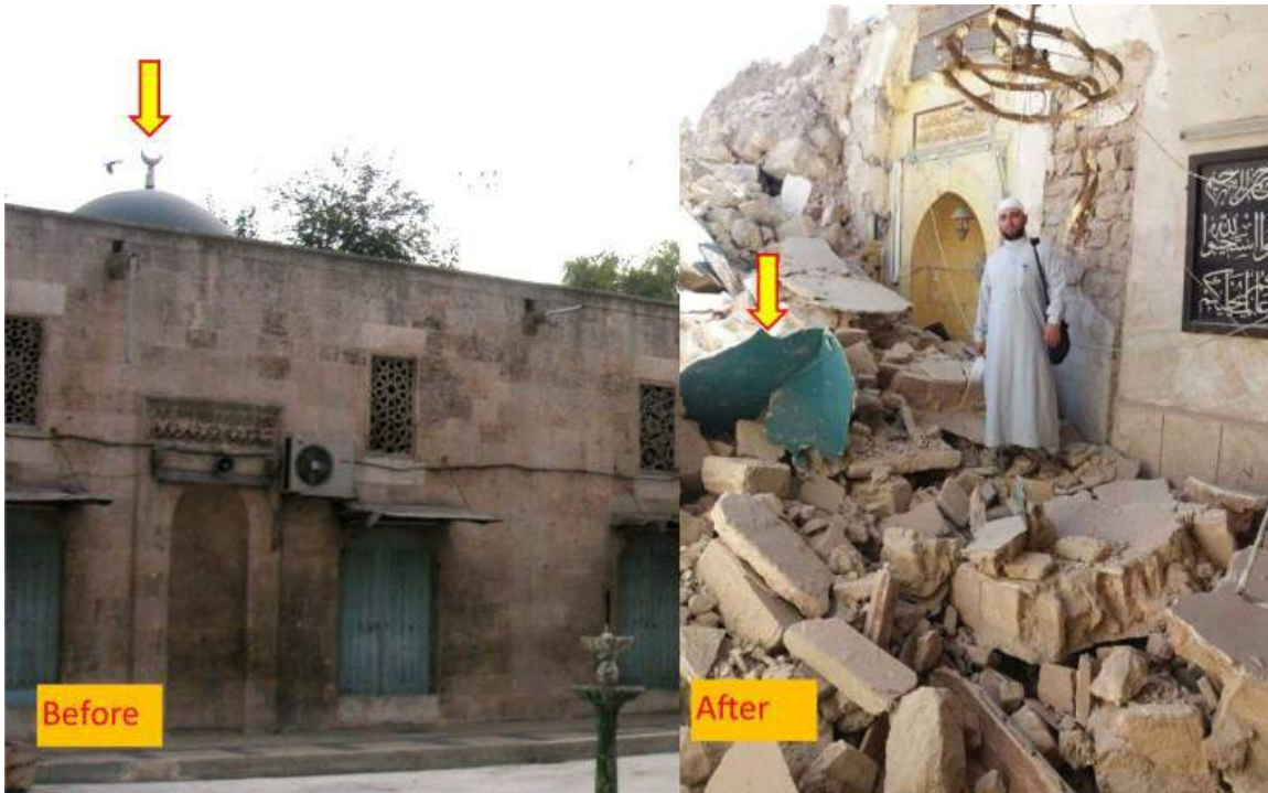
Damage to southern section of al-Tawba Mosque, including destroyed dome (APSA; October 6, 2016)
