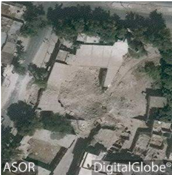
al-Tawba Mosque with severe damage to the courtyard and southern portion of the mosque (DigitalGlobe; September 25, 2016)
