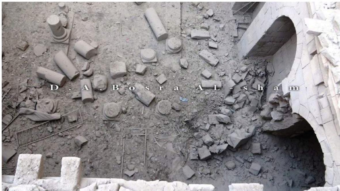
Damage to Ayyubid Citadel (Bosra al-Sham Department of Antiquities; December 22, 2015)
