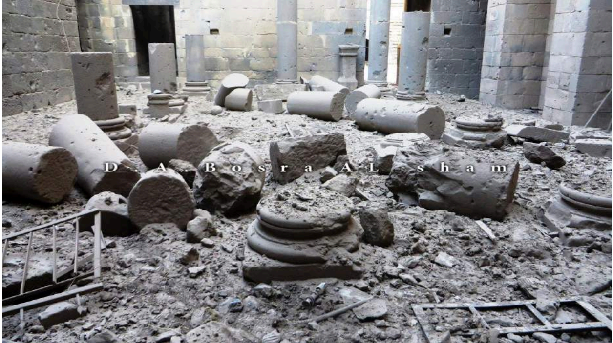
Collapse of columns in western section of Ayyubid Citadel (Bosra al-Sham Department of Antiquities; December 22, 2015)
