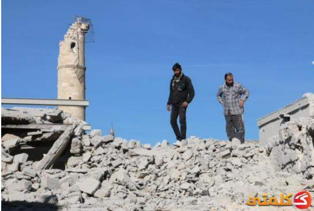
Possible photograph of damage to Al Batul Mosque (Anatolia Arabic; December 25, 2015)
