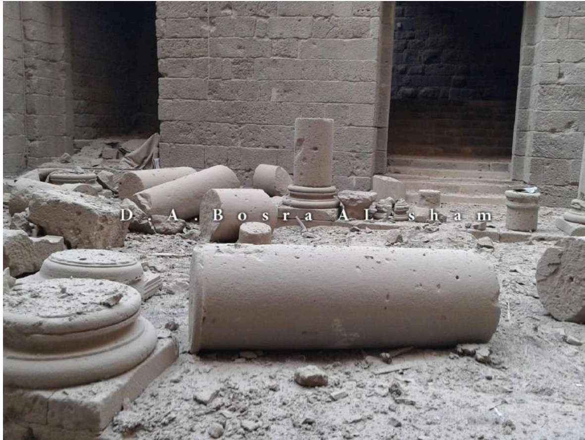
Damage to Ayyubid Citadel (Bosra al-Sham Department of Antiquities; December 22, 2015)
