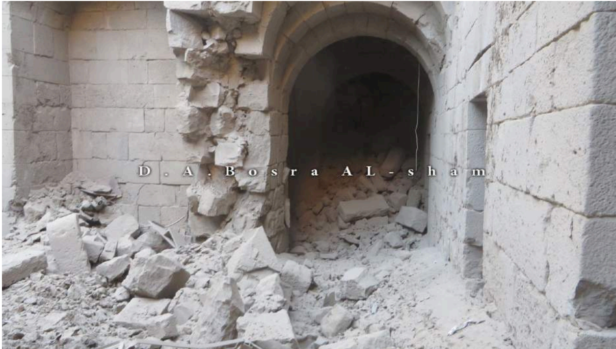
Damage to Ayyubid Citadel (Bosra al-Sham Department of Antiquities; December 22, 2015)
