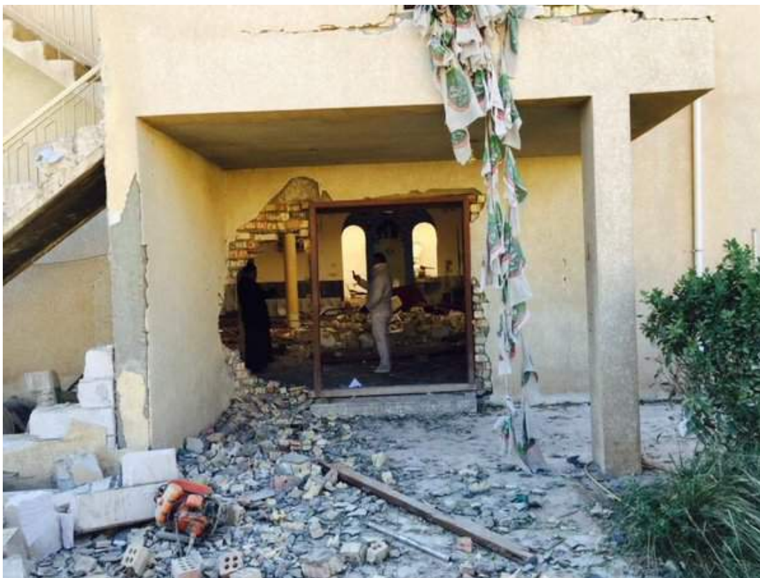
Damage to the exterior of Ammar Bin Yasser Mosque (Twitter; January 4, 2016) 79
