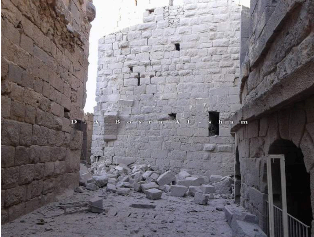
Damage to Ayyubid Citadel, Arch in front of Folklore Museum (Bosra al-Sham Department of Antiquities; December 23, 2015)
