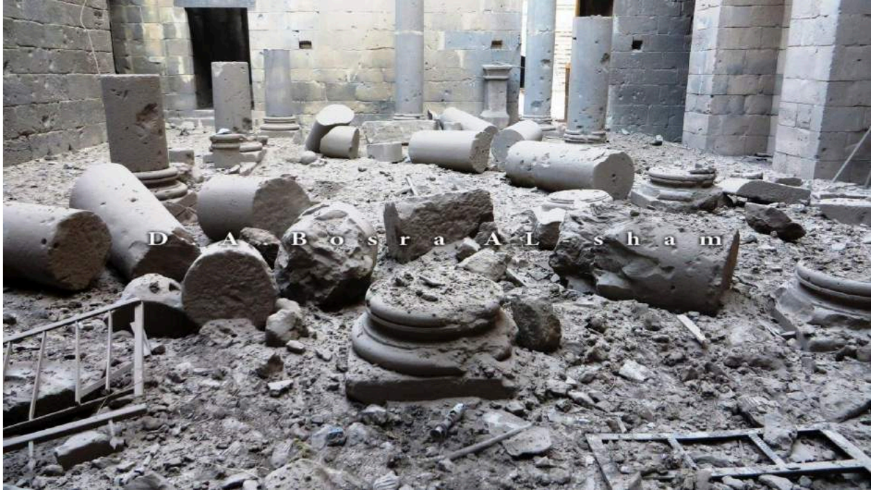
Collapse of columns in western section of Ayyubid Citadel (Bosra al-Sham Department of Antiquities; December 22, 2015)
