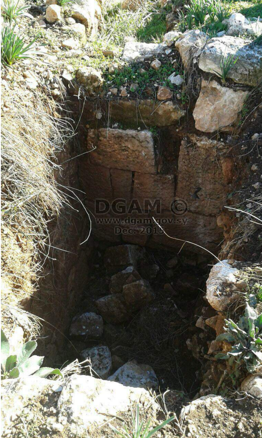
Kefr Aqab showing illegal excavation (DGAM; December, 15, 2015)
