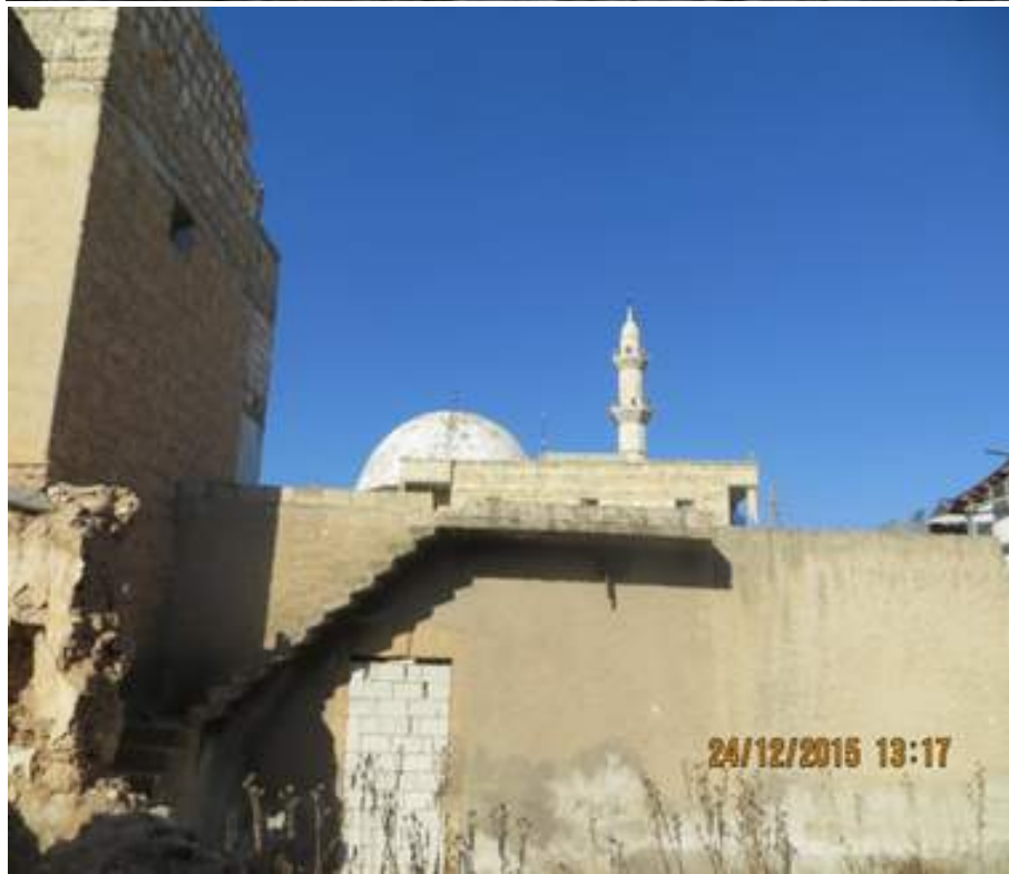
Damage to the south side of the mosque and archaeological remains of the original 1850 building
