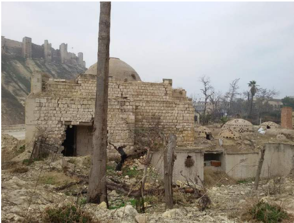
Damage to Hammam Yalbugha al-Nasiri (Private Facebook Account; December 26, 2016)
