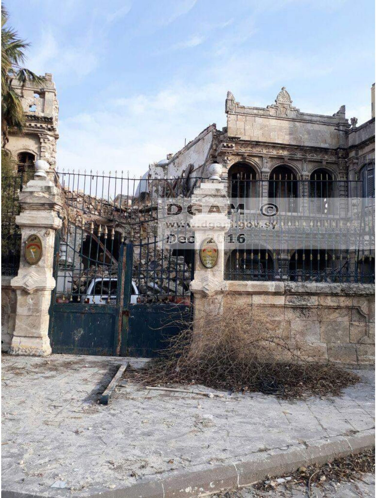
Collapsed section of Dar al-Iftaa (DGAM; December 24, 2016)
