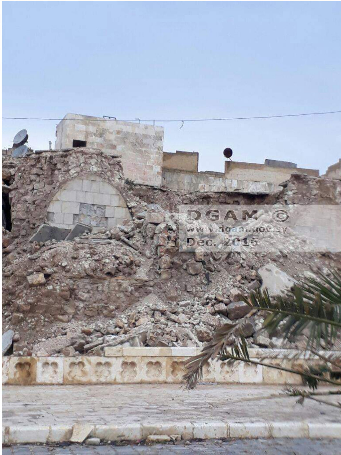
Damage to the ancient city wall and tower (DGAM; December 24, 2016)
