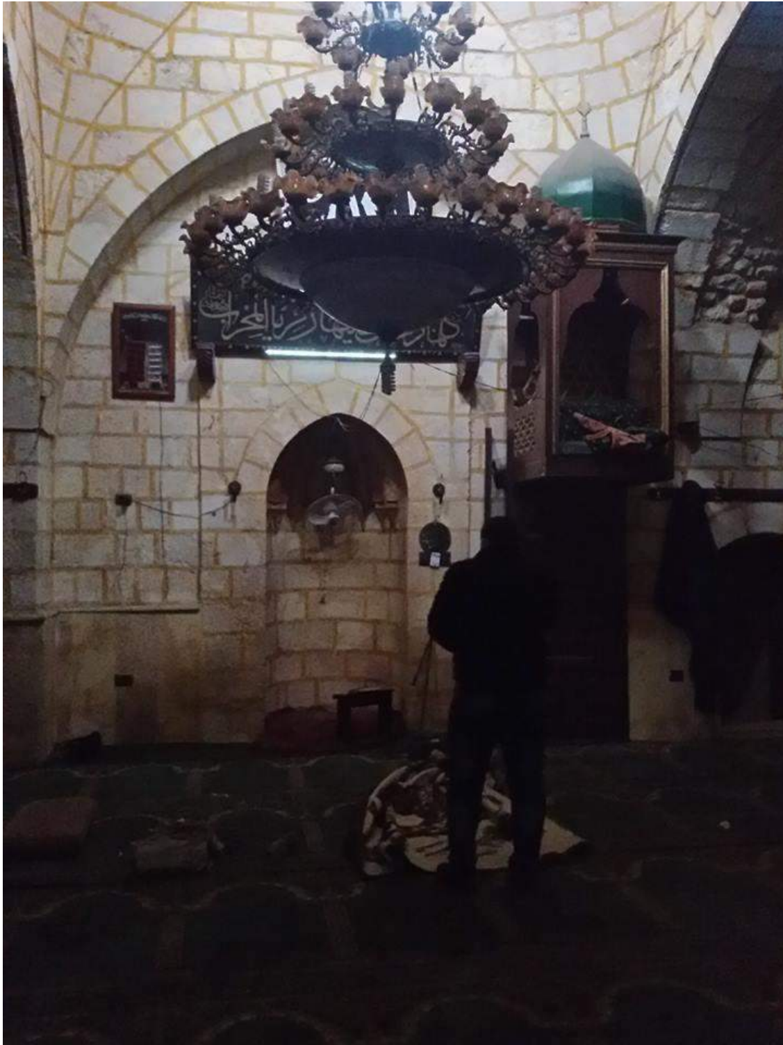
Minimal damage to al-Karamiya Mosque (Private Facebook Account; December 24, 2016)
