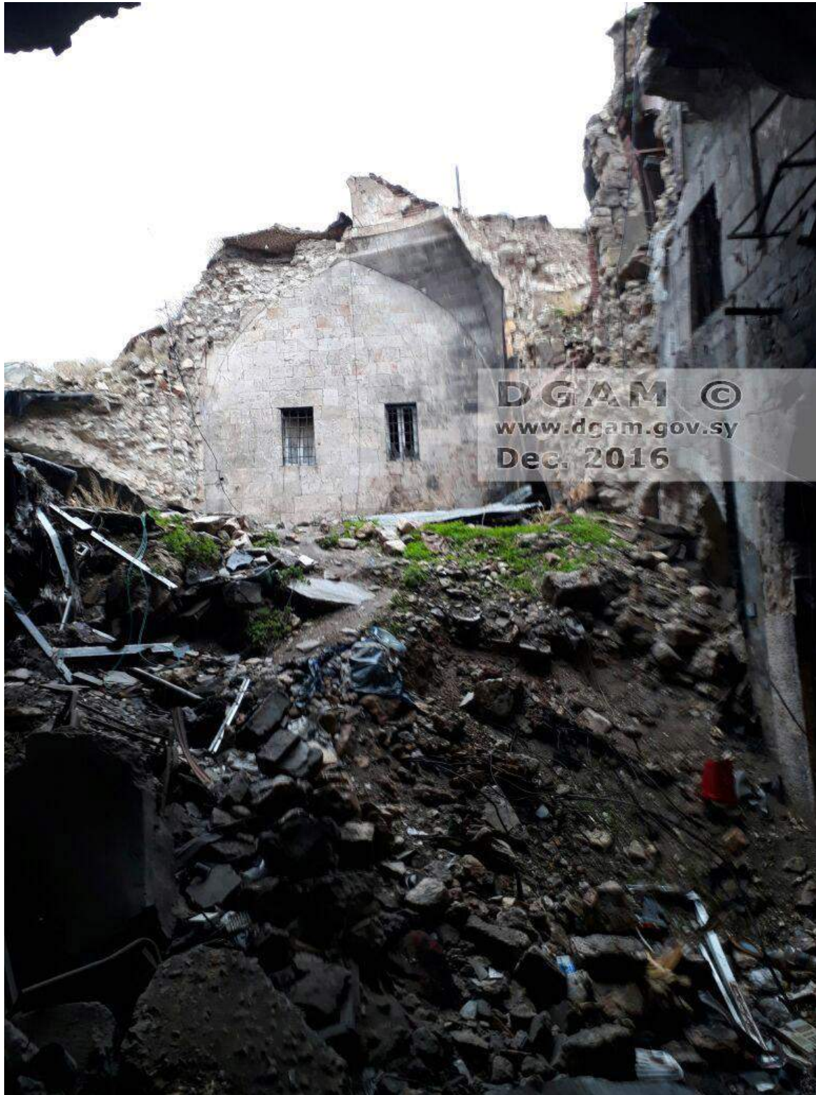
Severe damage to Khan al-Oulabiya (DGAM; December 16, 2016)
