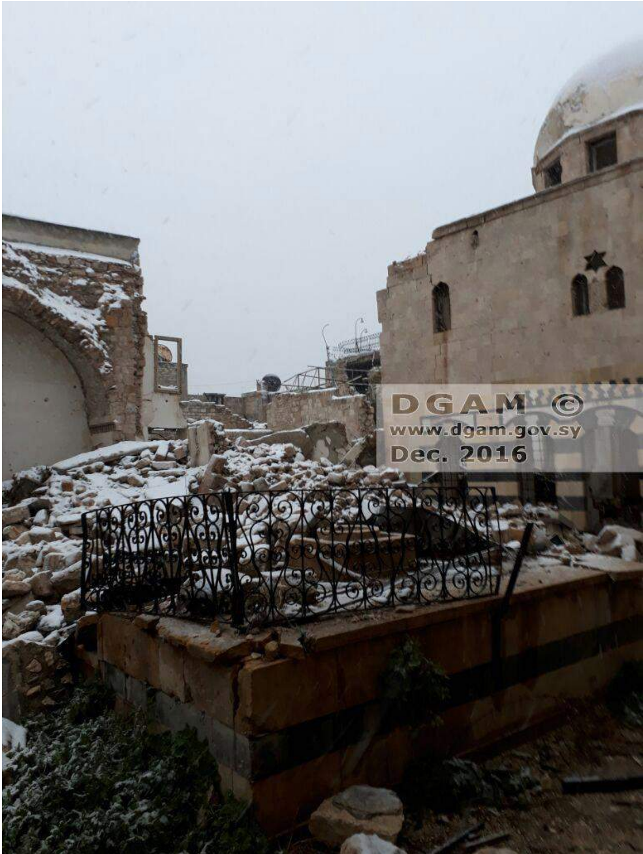
Severe damage to Beit Ghazaleh (DGAM; December 22, 2016)
