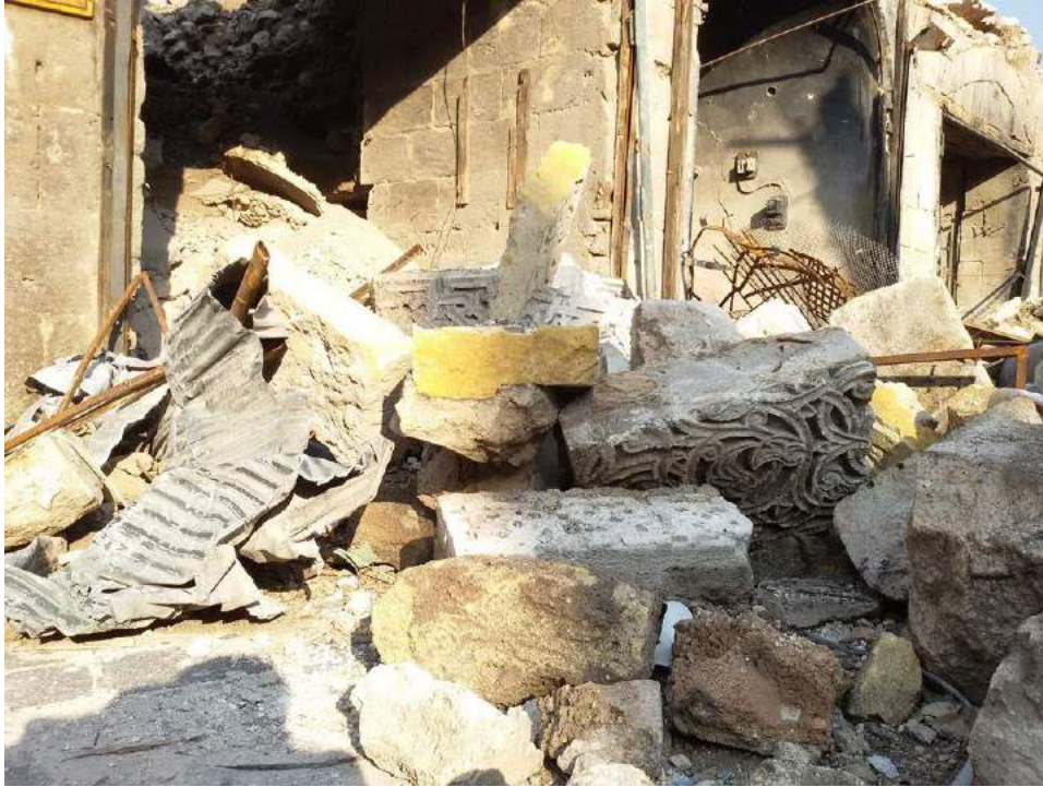
Damage to the shops of the Khan Uch Khan (Private Facebook Account; December 19, 2016)
