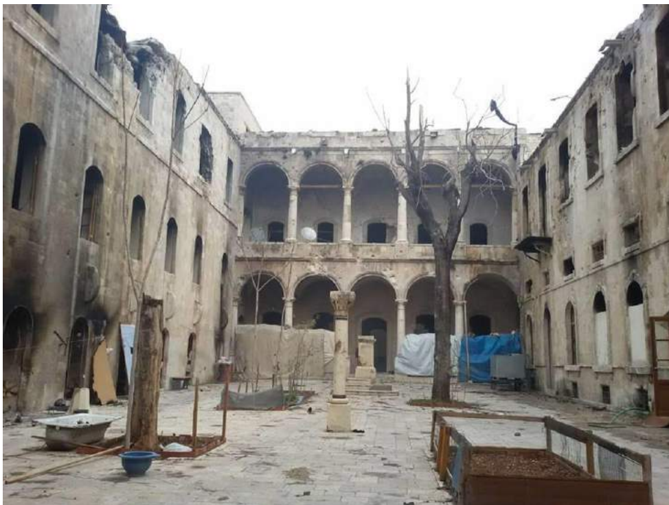
Explosives and fire damage to al-Shibani Church and School (Private Facebook Account; December 24, 2016)
