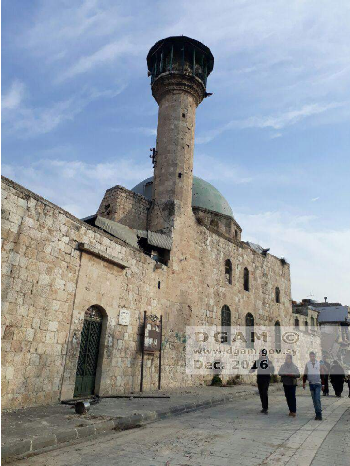
Al Hamwi Mosque showing minimal damage (DGAM; December 24, 2016)
