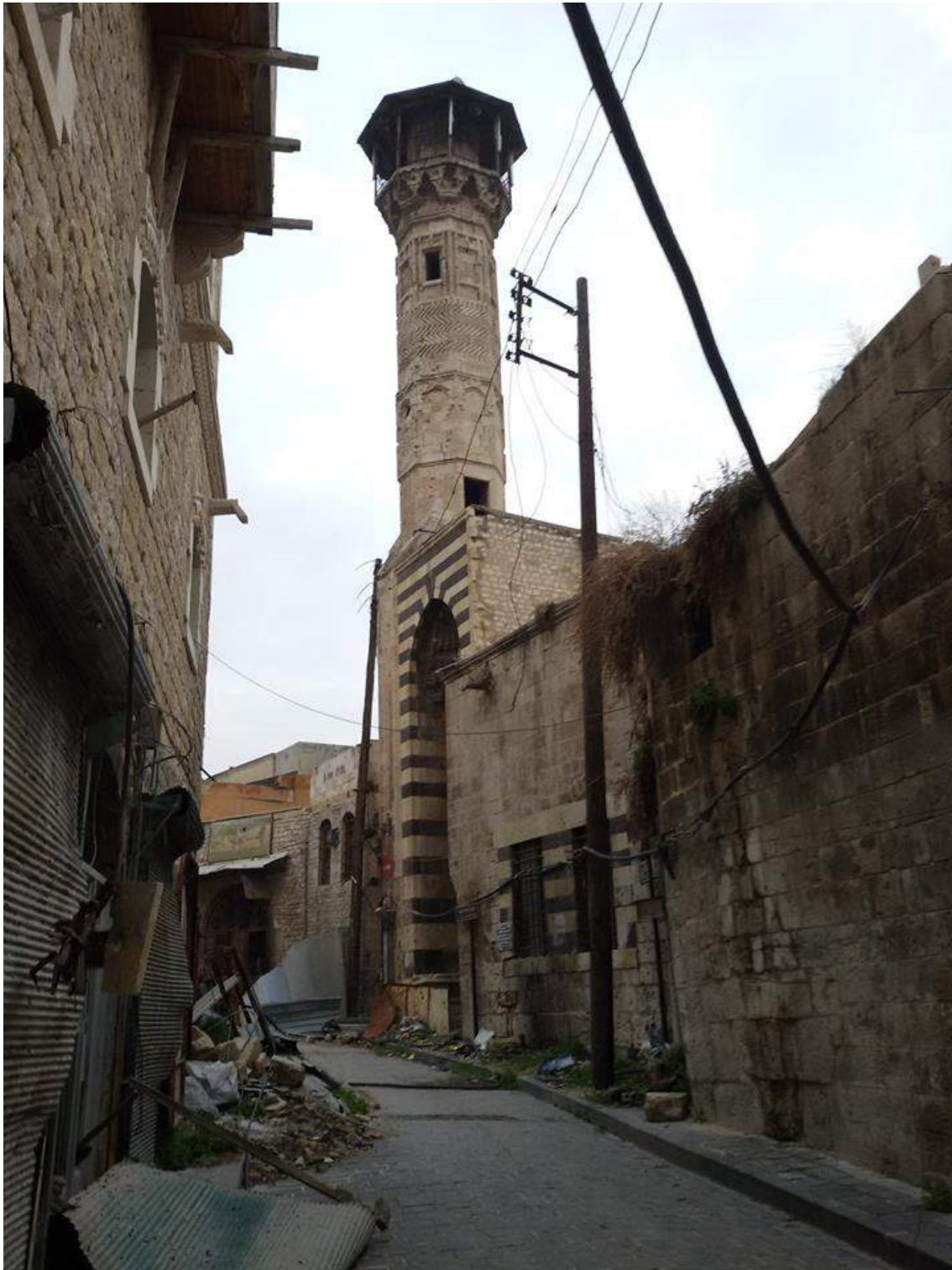
Damage and overgrowth at Saffahiya Mosque (Private Facebook Account; December 20, 2016)
