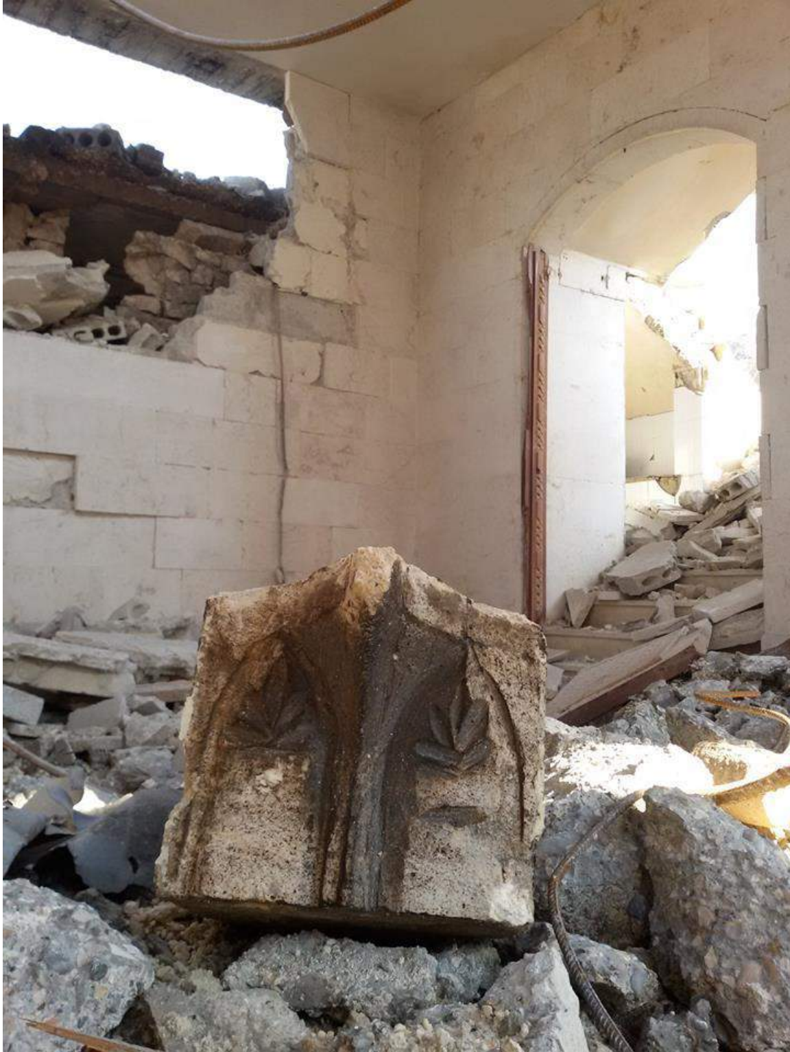
Extensive damage and rubble at al-Maidani Mosque (Private Facebook Account; December 19, 2017)
