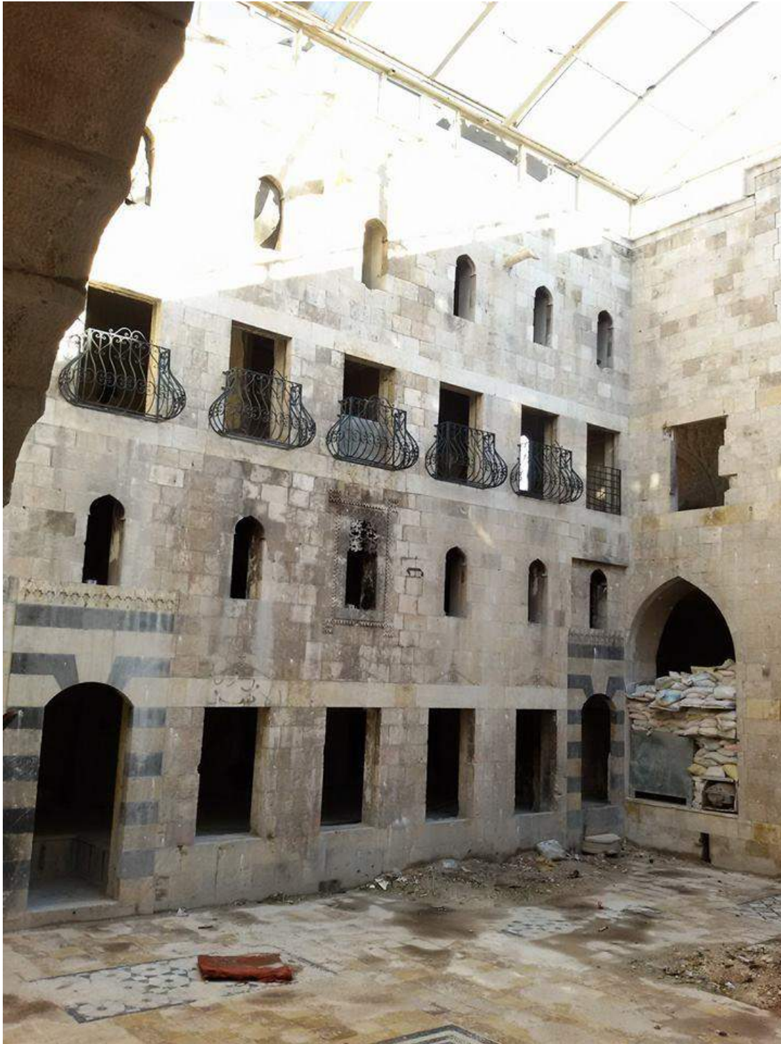
Minimal damage seen in this view of Hotel Zamaria, presence of sandbags in the far right window suggest militarization of the site (Private Facebook Account; December 17, 2016)
