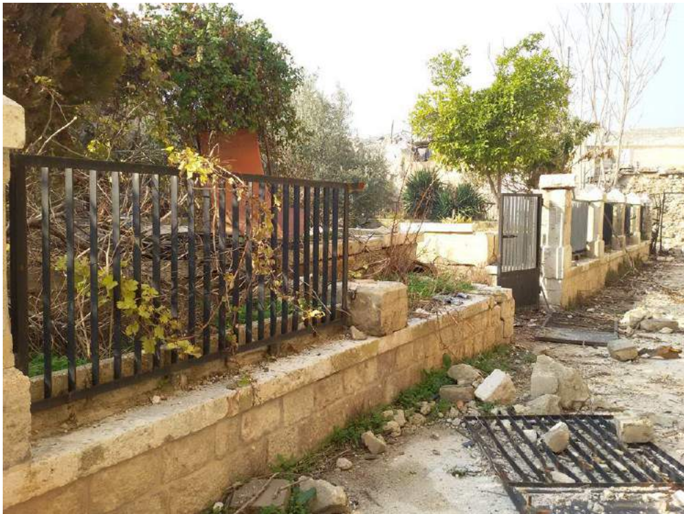
Damage to the grounds of the Yassou'iya (Private Facebook Account; December 19, 2016)
