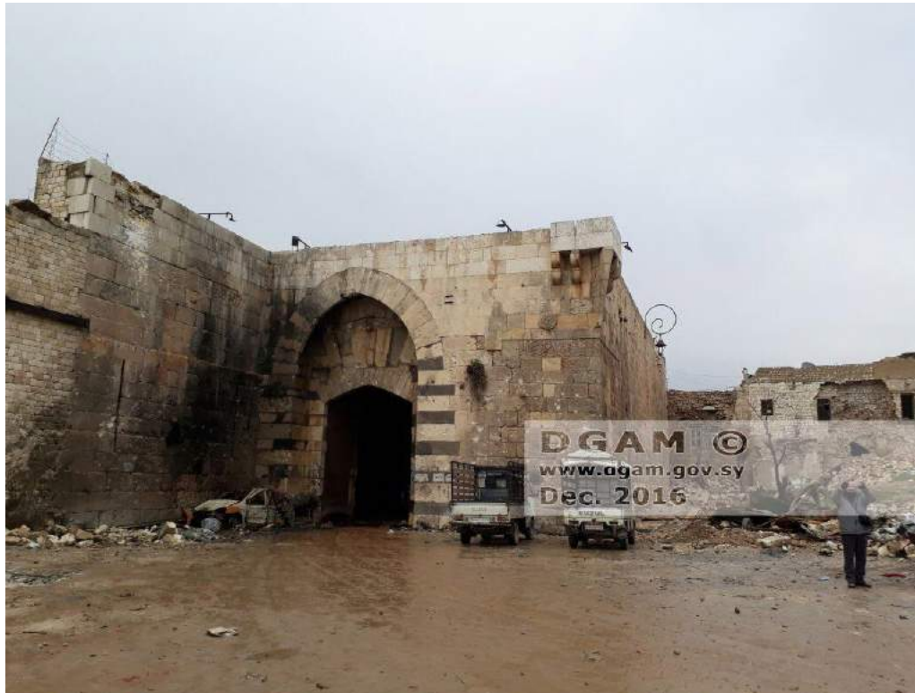
Smoke damage to the exterior of Bab Qinnasrin (DGAM; December 24, 2016)
