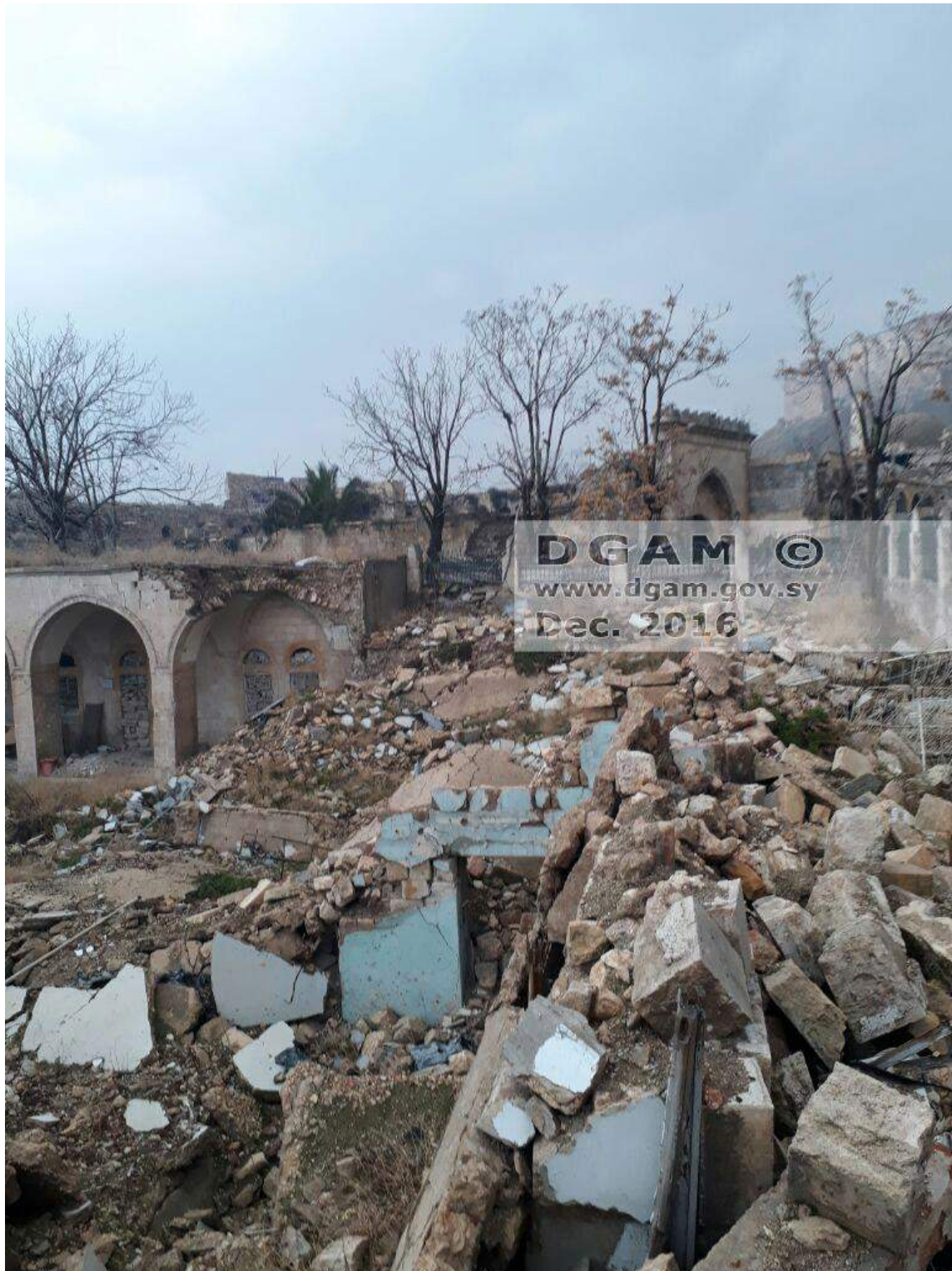
Extensive damage to Madrasa Khusruwiye (DGAM; December 28, 2016)
