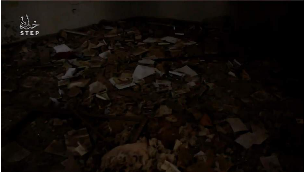
Video still of damage to the Church of Mary (Step News Agency; December 26, 2016)
