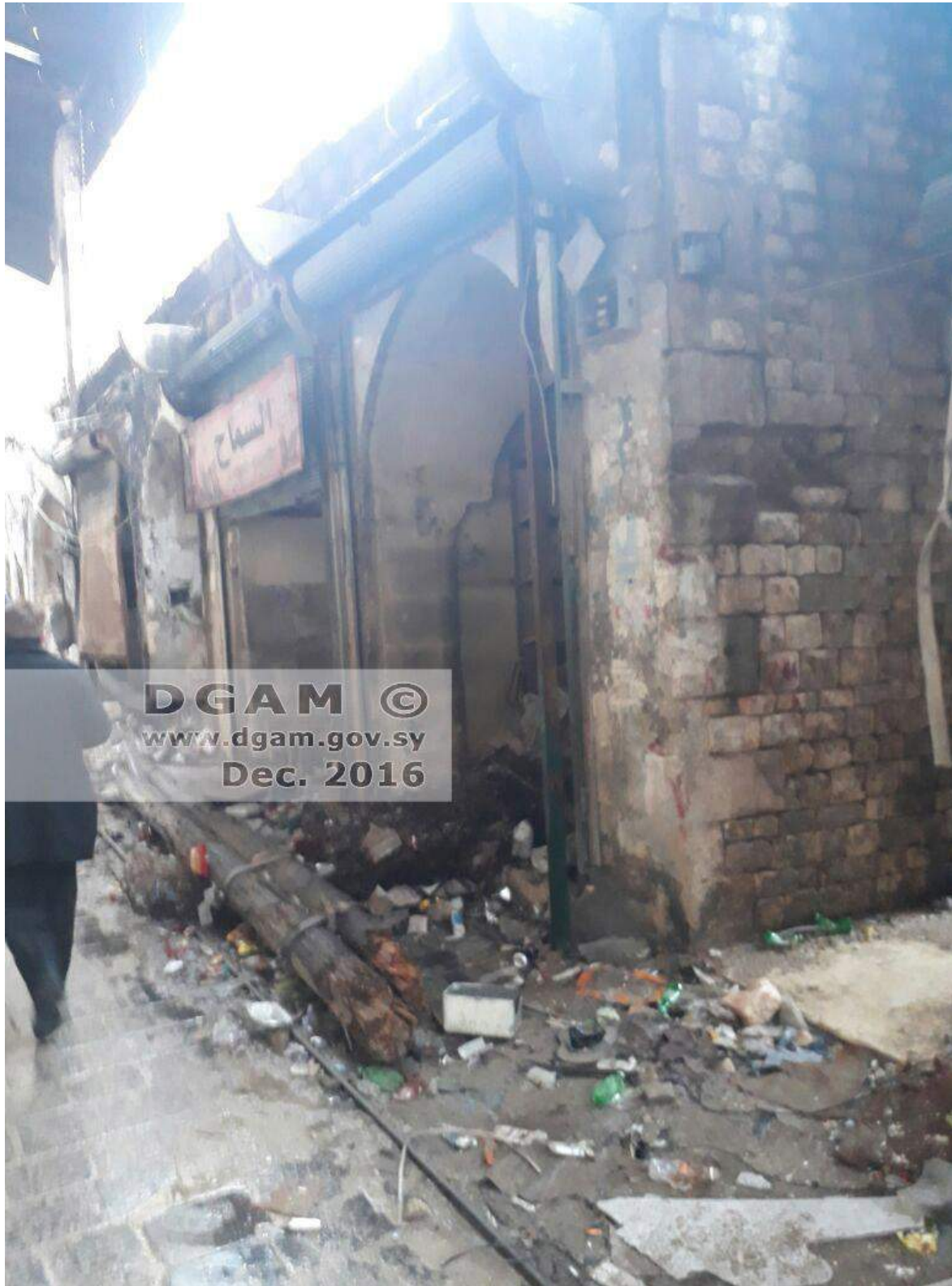
Damage to the shops within Suq al-Suweiqqa (DGAM; December 16, 2016)
