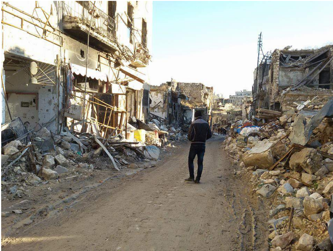
Extensive damage to Suq al-Samak (Private Facebook Account; December 15, 2016)
