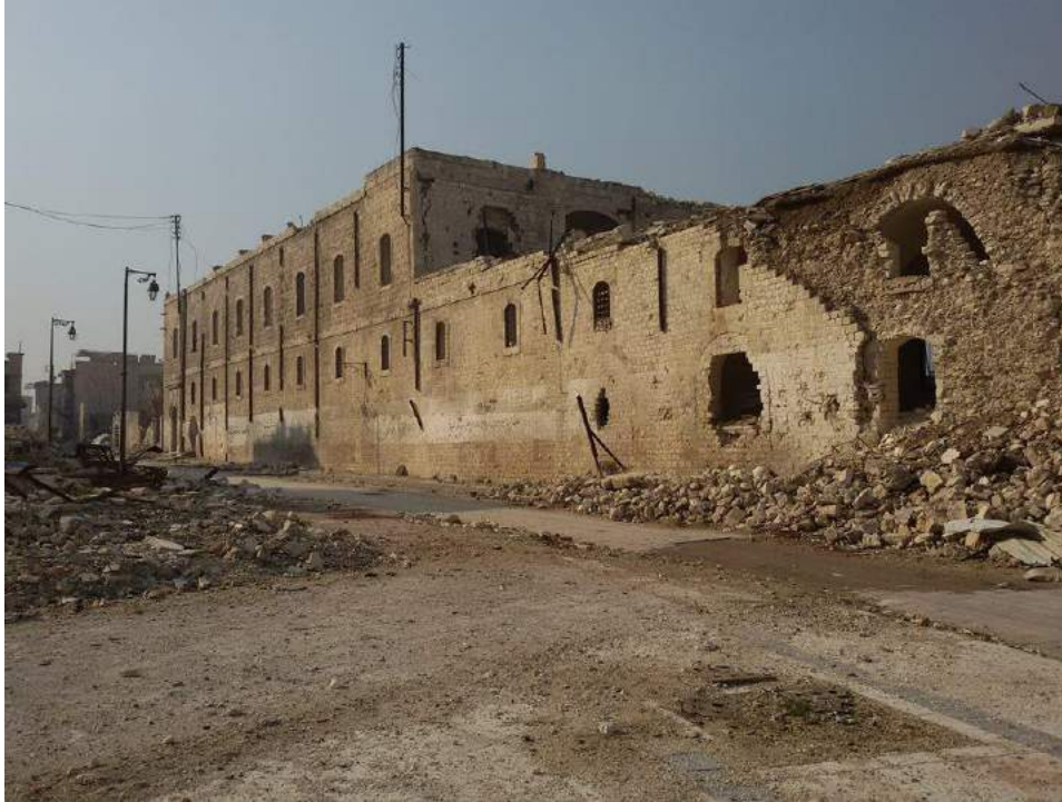
Exterior damage seen to Assma Bent Abo Bakr School (Private Facebook Account; December 19, 2016)
