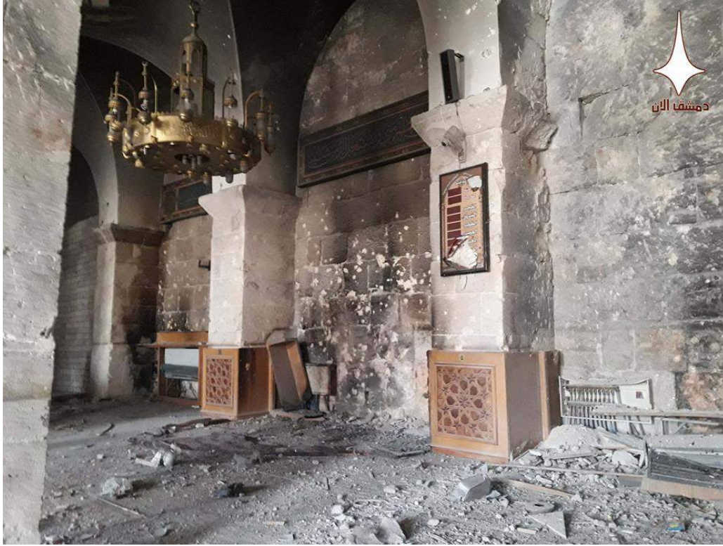
Damage to the interior of the Umayyad Mosque (Dimashq al-Aan; December 19, 2016)
