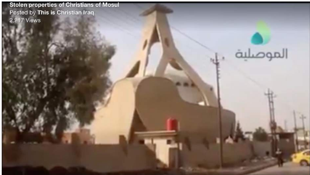
Video still of the Chaldean Catholic Church of the Holy Spirit showing little to no damage (This is Christian Iraq; December 20, 2016)
