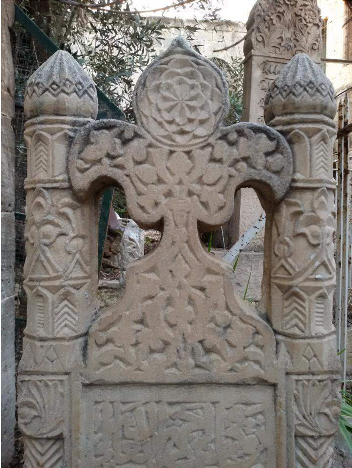
Material damage seen at Takkiya Nasimi (Private Facebook Account; December 19, 2016)
