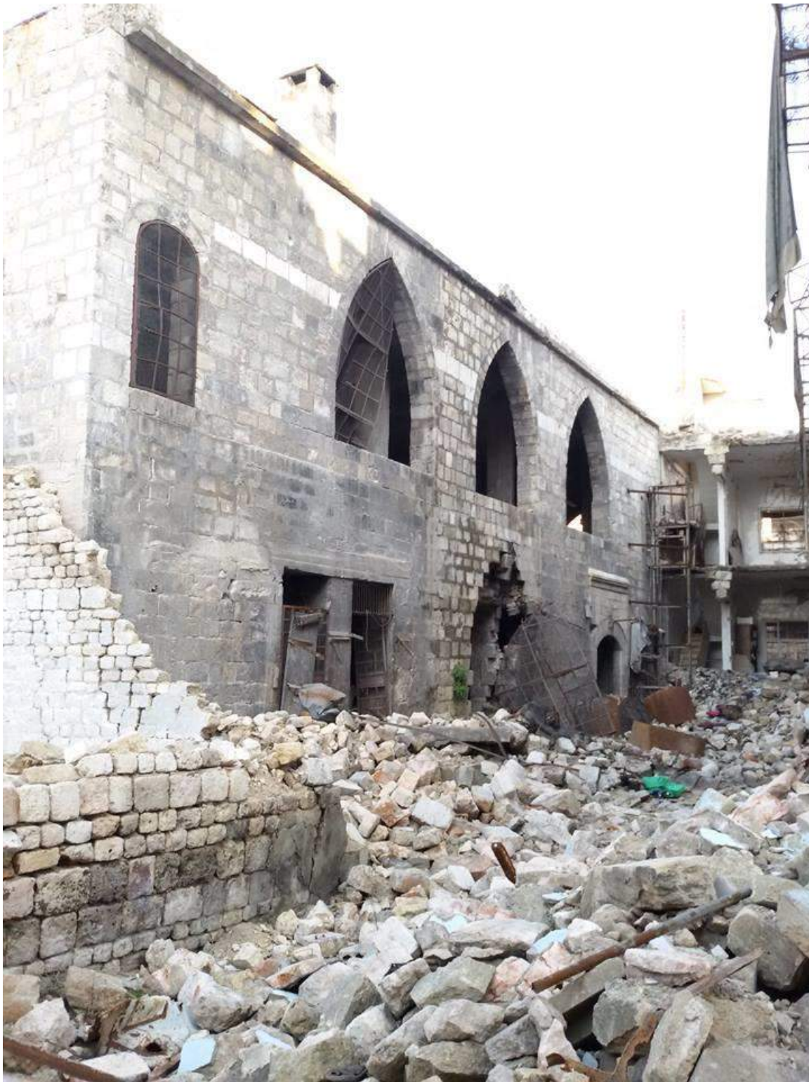
Damage to the exterior of Musabnat al-Jabili (Private Facebook Account; December 19, 2016)
