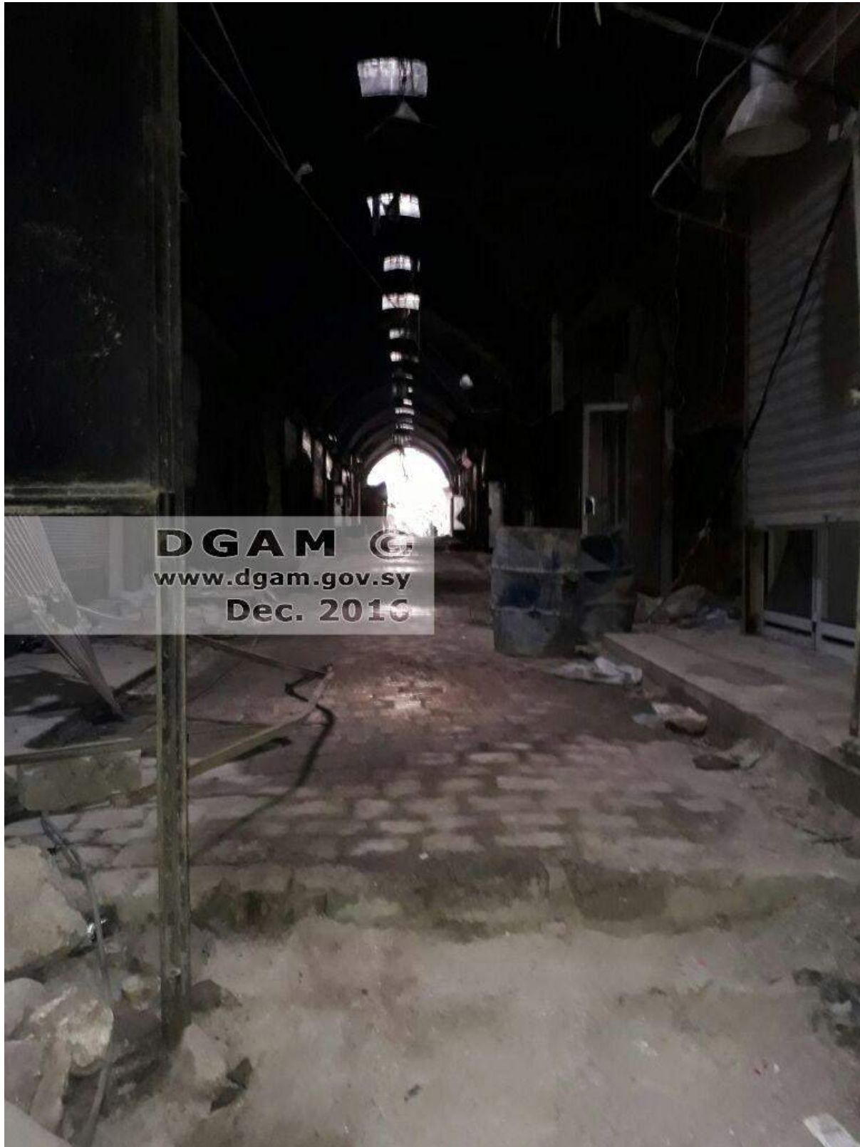
Fire damage to the interior of Suq al-Joukh (DGAM; December 16, 2016)
