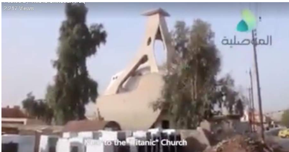
Video still of the front of the Chaldean Catholic Church of the Holy Spirit, showing little to no damage (This is Christian Iraq; December 20, 2016)
