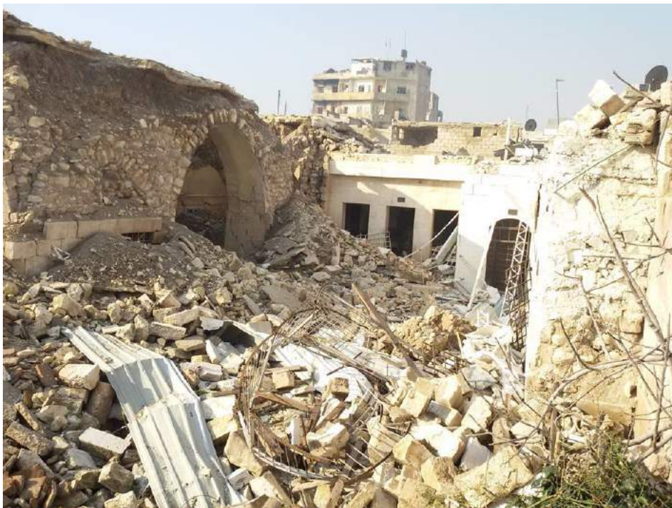
Extensive destruction of al-Maidani Mosque (Private Facebook Account; December 19, 2017)
