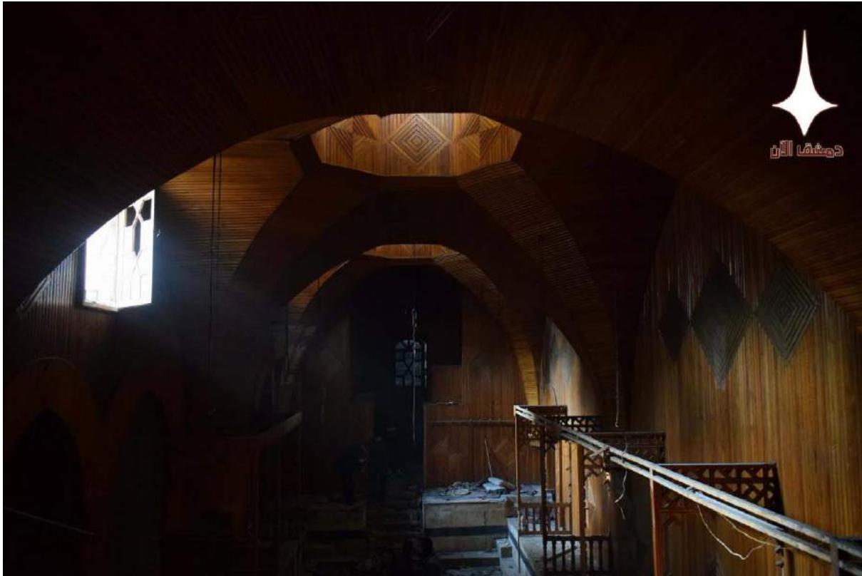
Damage to the interior of Hammam al-Nahasin (Dimashq al-Aan; December 19, 2016)
