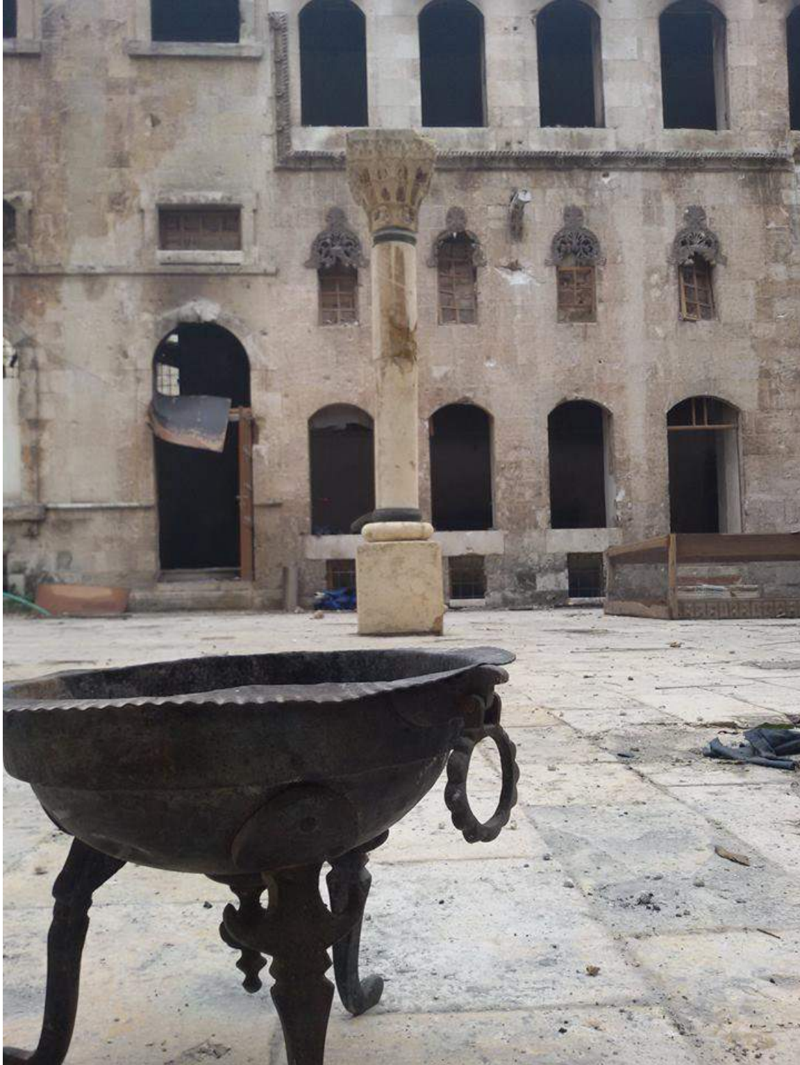
Explosives damage at al-Shibani Church and School (Private Facebook Account; December 24, 2016)
