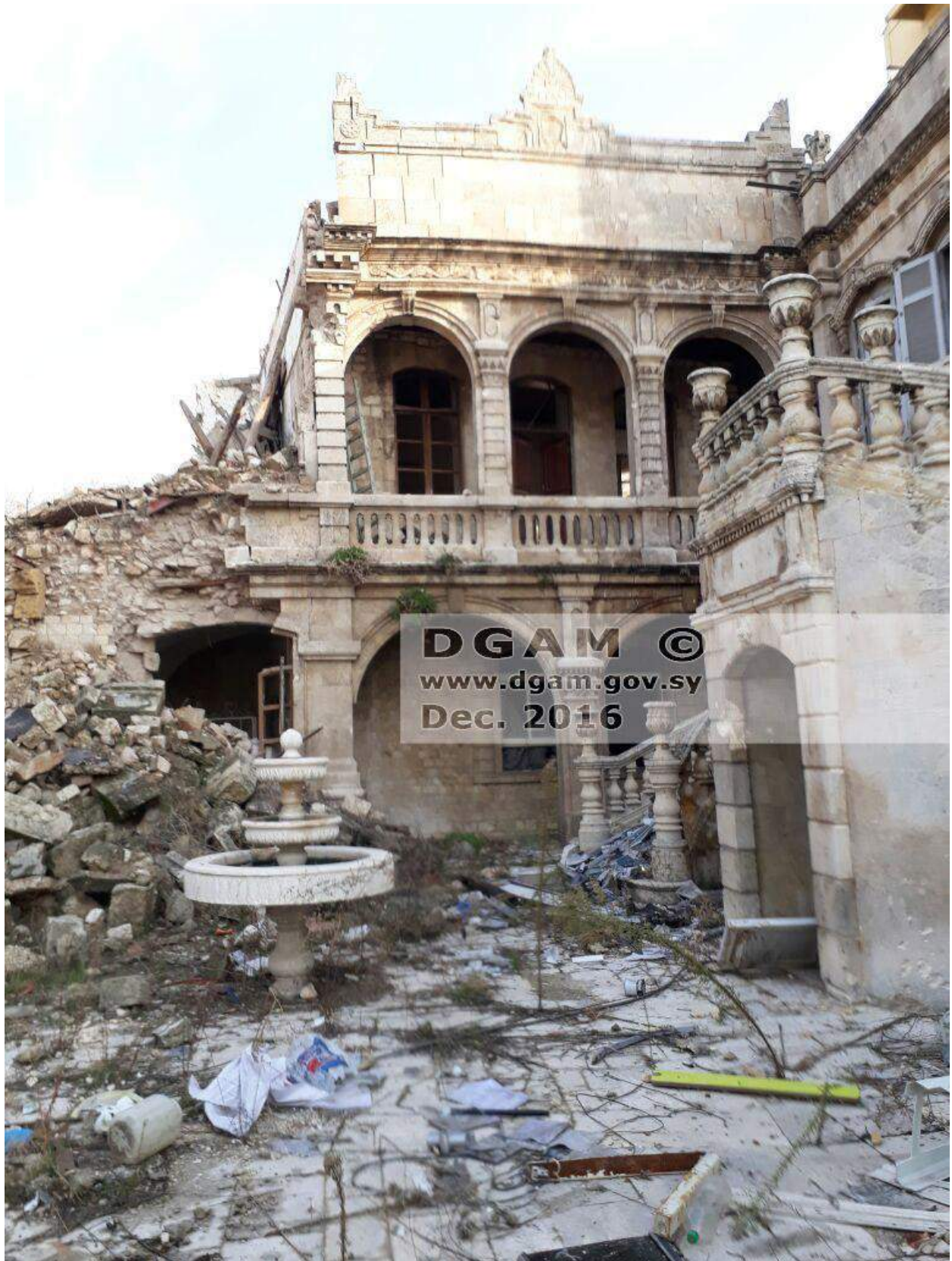
Collapsed section of Dar al-Iftaa and debris scattered in the courtyard (DGAM; December 24, 2016)
