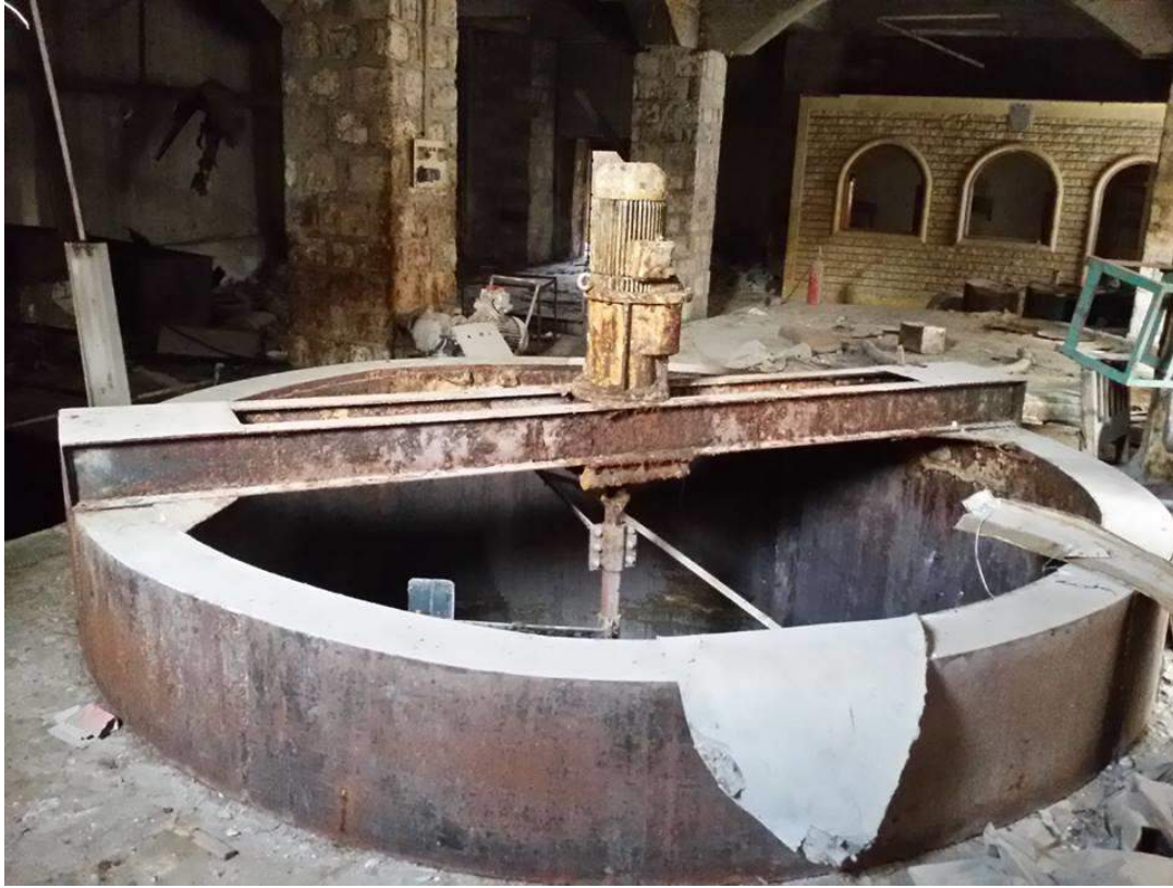
Damage to the interior of Musabinat al-Jabili (Private Facebook Account; December 19, 2016)
