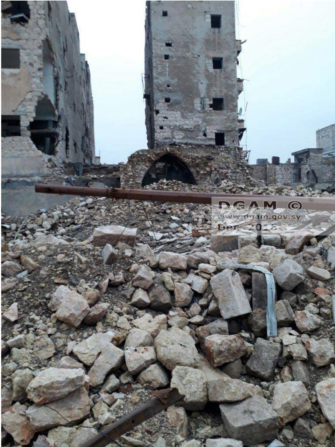
The destruction of Noor al-Dein Mosque (DGAM; December 25, 2016)
