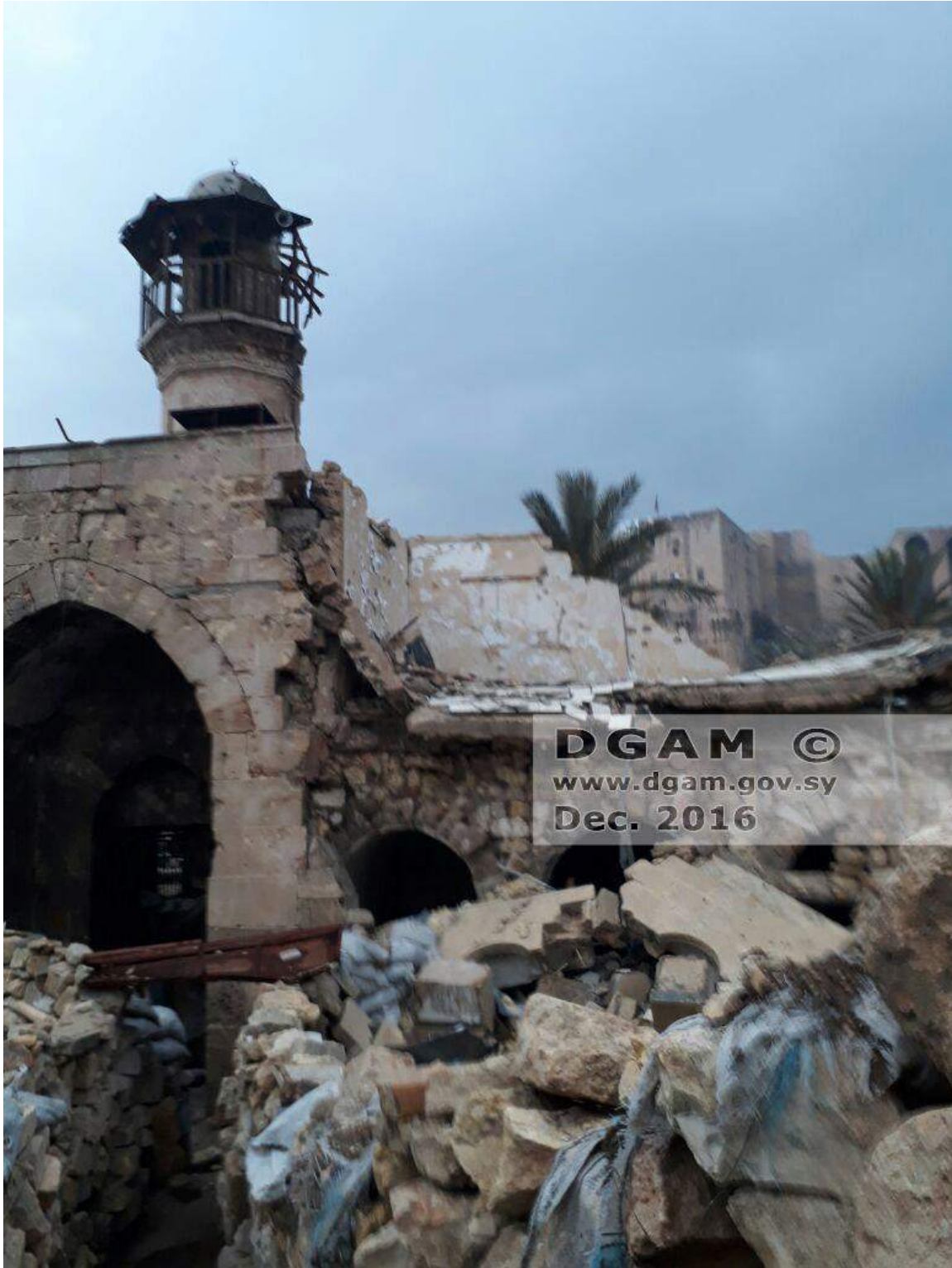
Extensive damage to al-Sultaniyah Mosque and Madrasa (DGAM; December 28, 2016)
