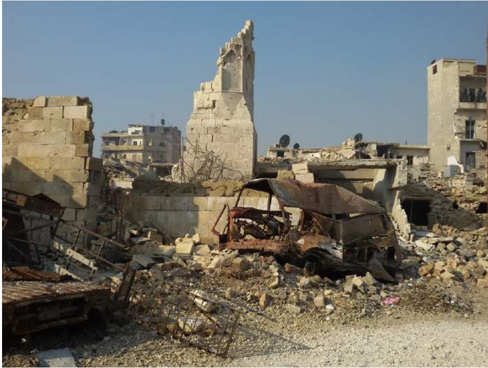
Extensive destruction of al-Maidani Mosque Minaret (Private Facebook Account; December 19, 2017)
