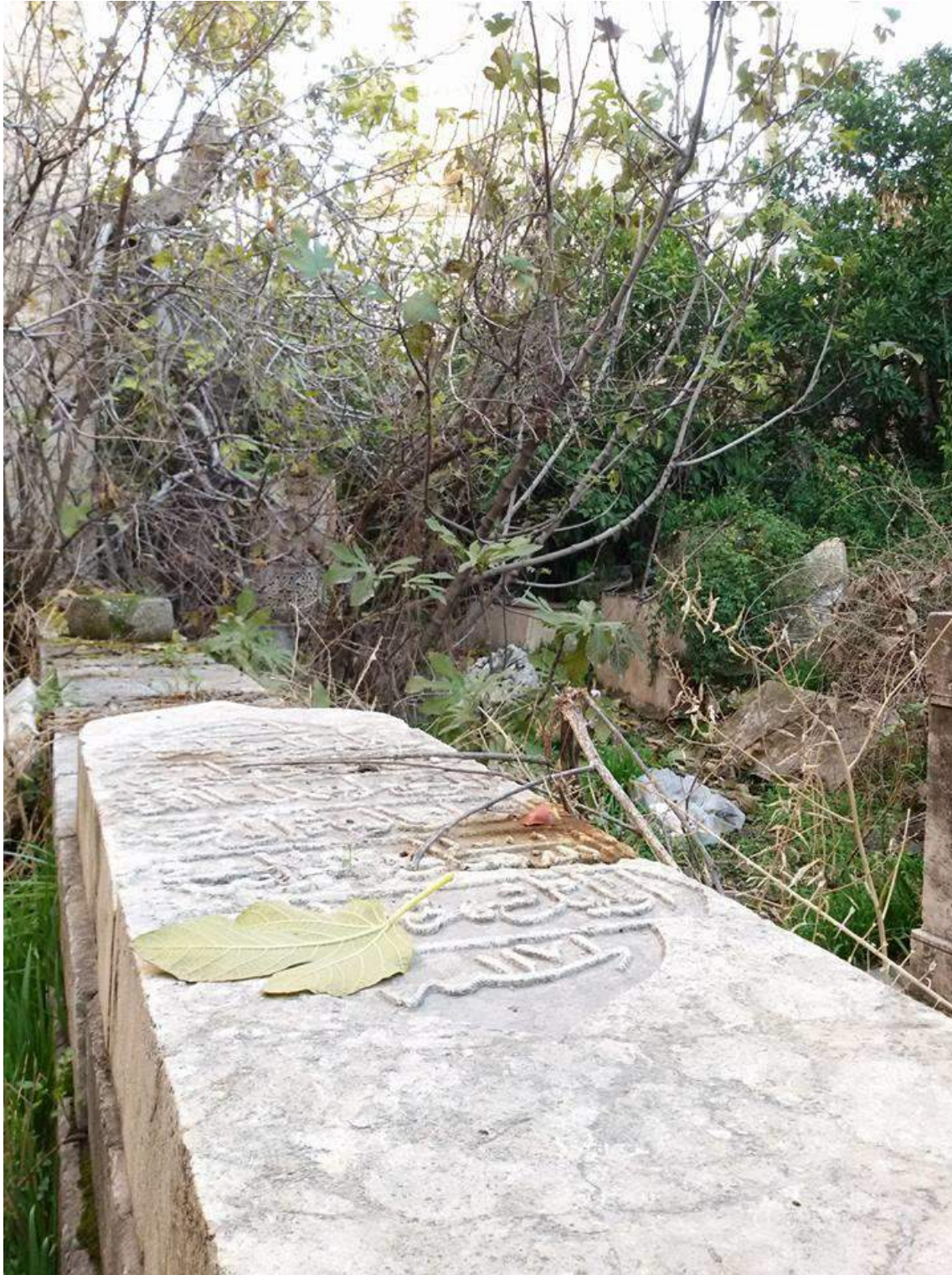
Damage to graves and overgrowth inside the Uthmaniya Mosque cemetery (Private Facebook Account; December 15, 2016)
