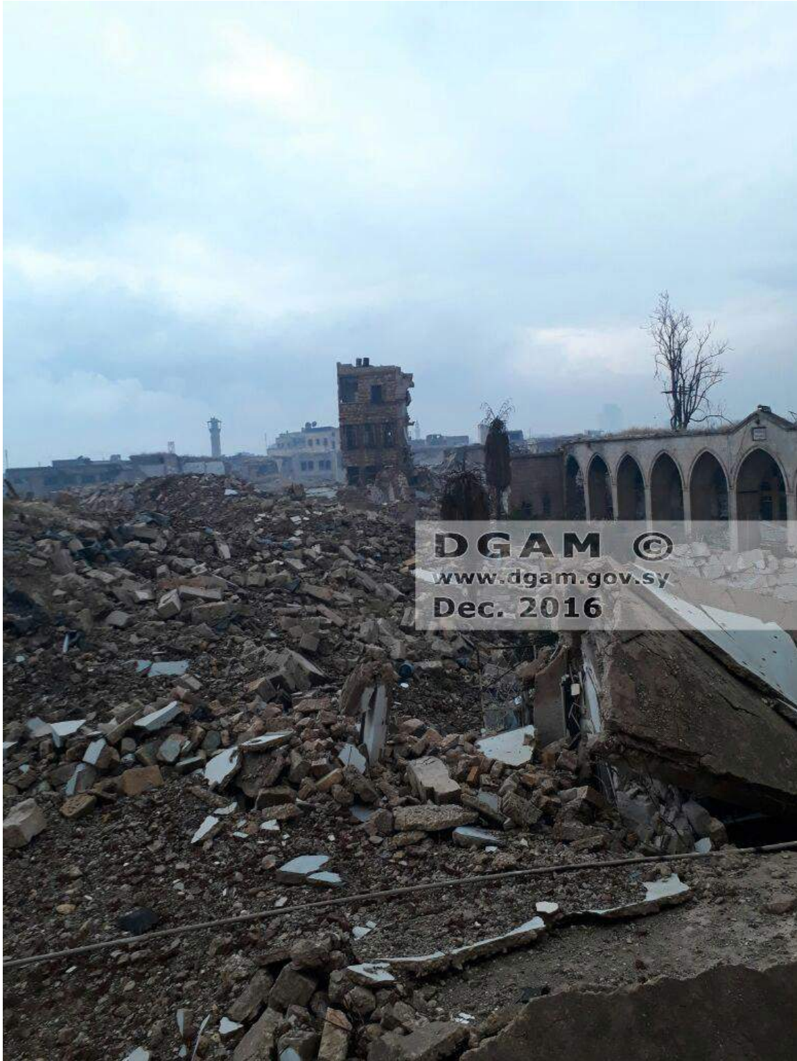
Extensive damage to Madrasa Khusruwiye (DGAM; December 28, 2016)
