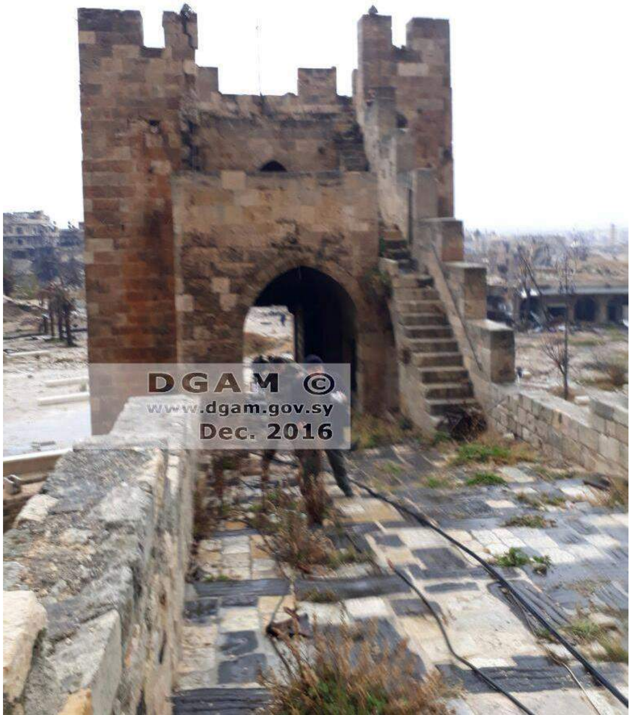
Damage to the entrance of the Citadel (DGAM; December 16, 2016)
