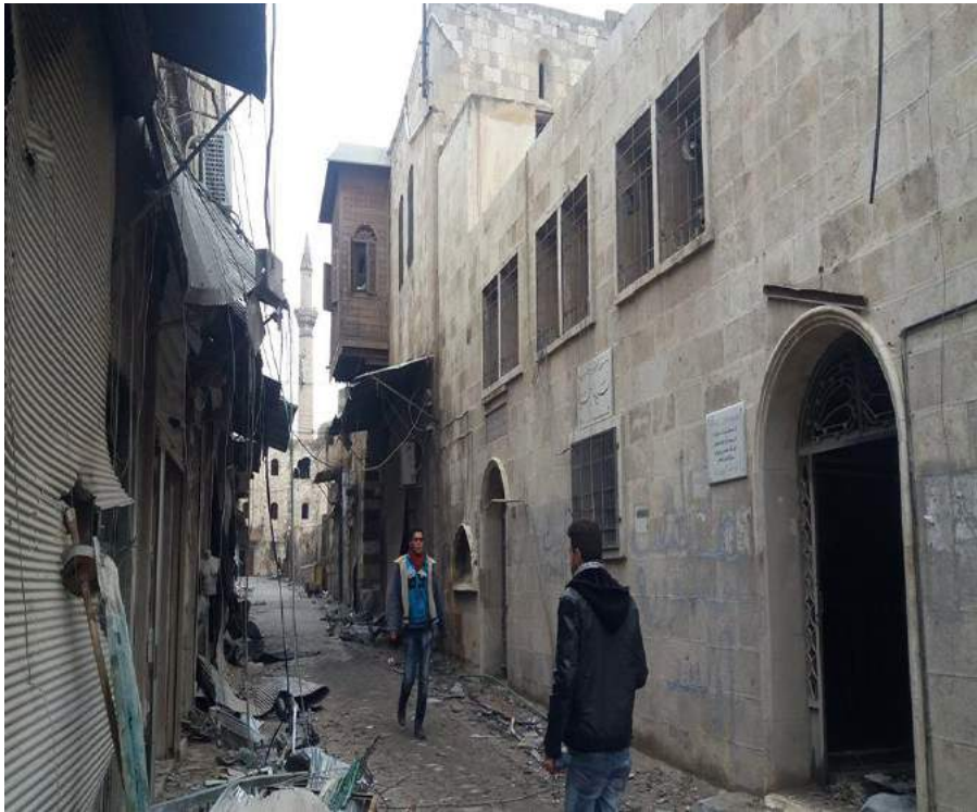
Light damage and graffiti present at Sayedna Hamza Mosque (Private Facebook Account; December 24, 2016)
