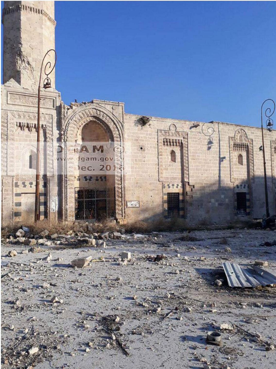
Damage seen to Mosque Ouroush (DGAM; December 20, 2016)
