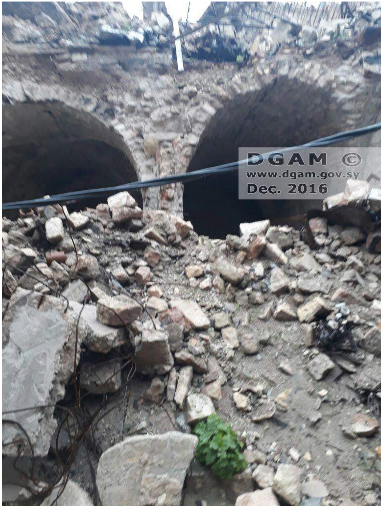
Collapsed part of the Suq al-Suweiqā (DGAM; December 16, 2016)
