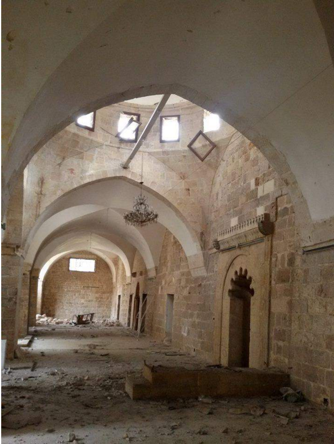
Damage to the interior of al-Omari Mosque (Private Facebook Account; December 17, 2016)
