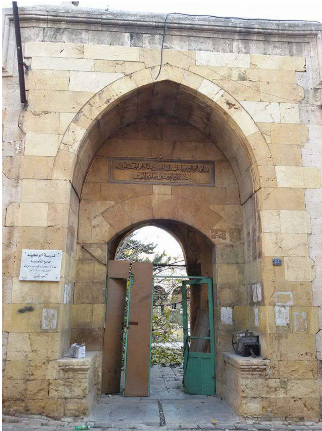
Broken doors seen at al-Uthmaniya Mosque (Private Facebook Account; December 15, 2016)
