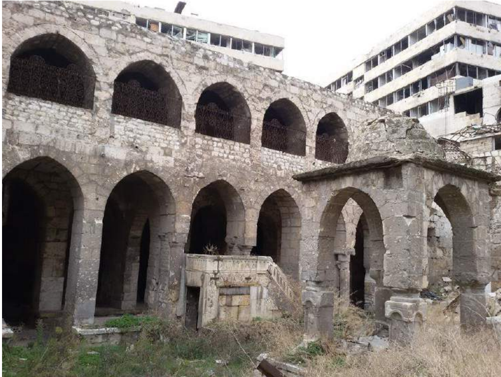
Damage to and overgrowth of vegetation at Bandara Synagogue (Private Facebook Account; December 17, 2016)
