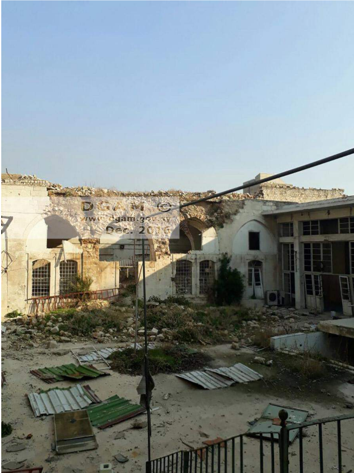
Damage and rubble present at Banqusa Mosque (DGAM; December 20, 2016)
