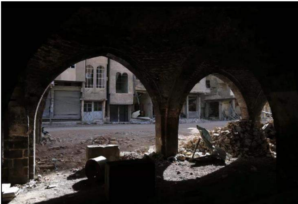
Extensive damage seen at Harasta Olive Oil Mill (Bisan Ilan Kurumu; November 22; 2016)
