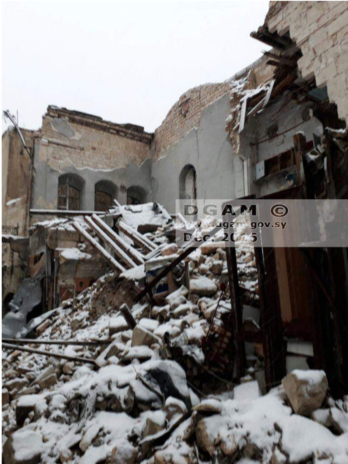
Severe damage to Beit Ghazaleh (DGAM; December 22, 2016)
