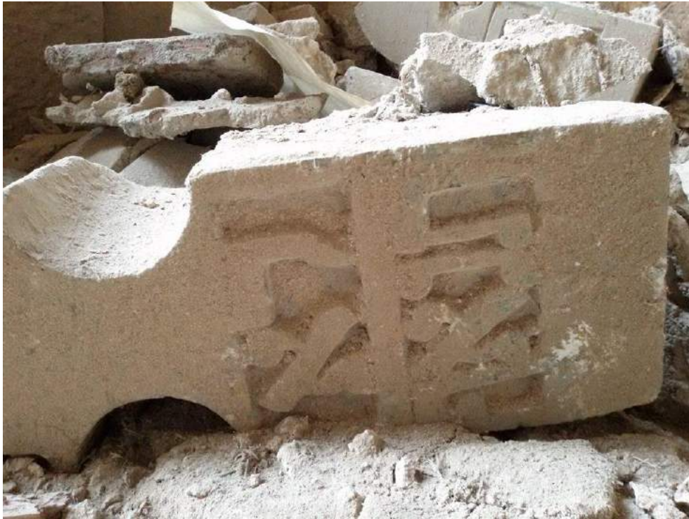
Detail of damage to Bandara Synagogue (Private Facebook Account; December 17, 2016)
