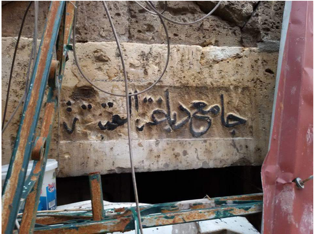
Detail of damage to Mosque Dabbagha al-'Atiqa (Private Facebook Account; December 17, 2016)
