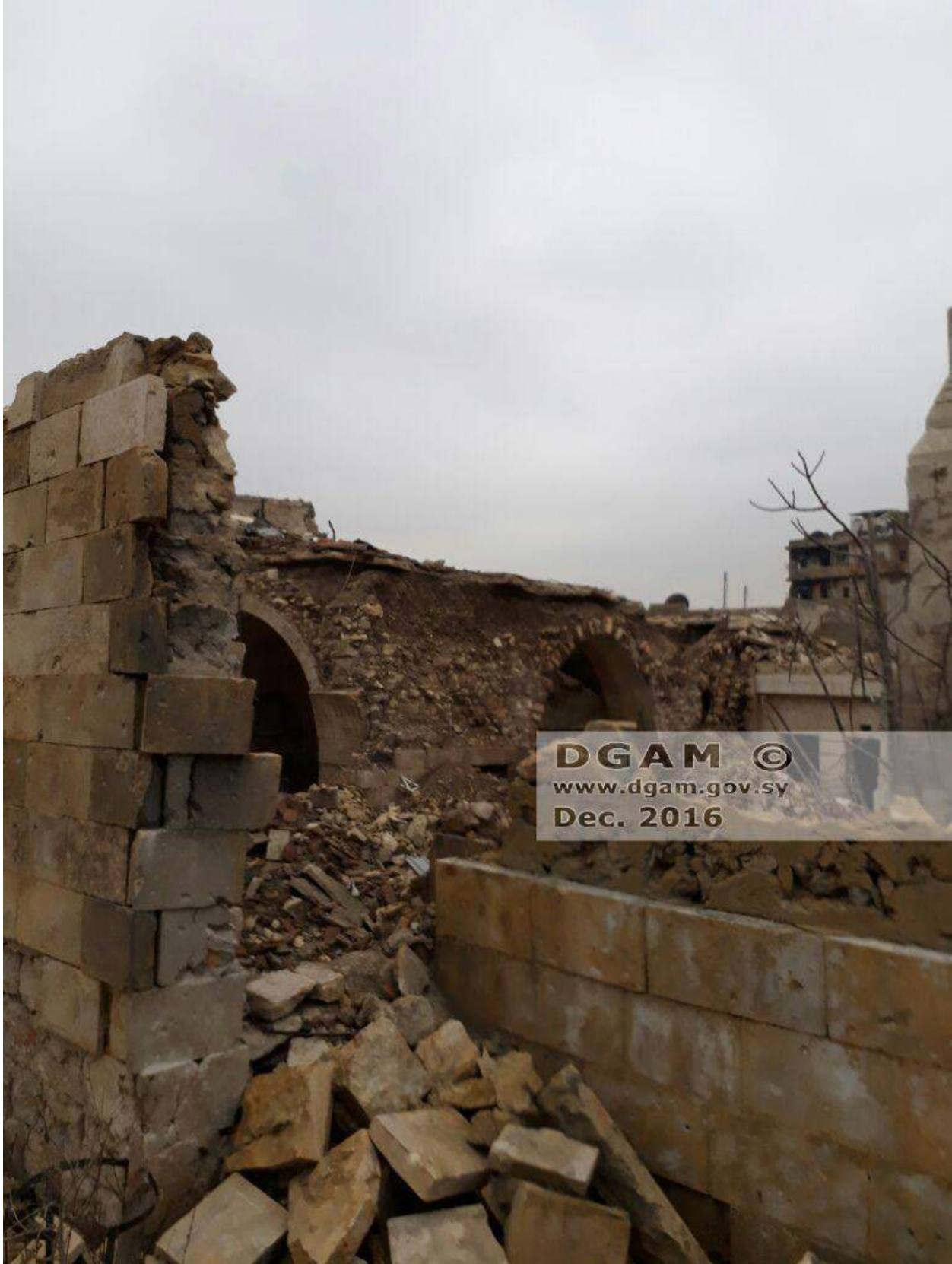
Extensive destruction of al-Maidani Mosque (DGAM; December 24, 2016)
