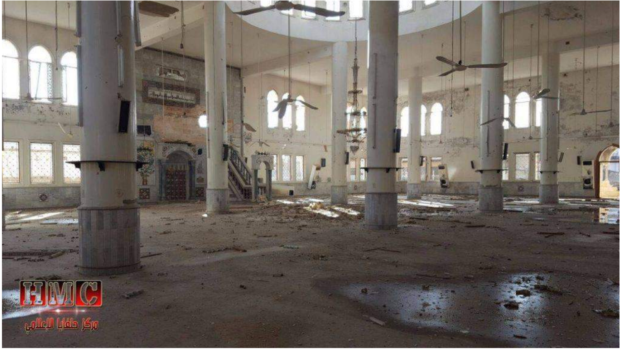
Damage to Halfaya al-Kabir Mosque (SNHR: December 30, 2016)
