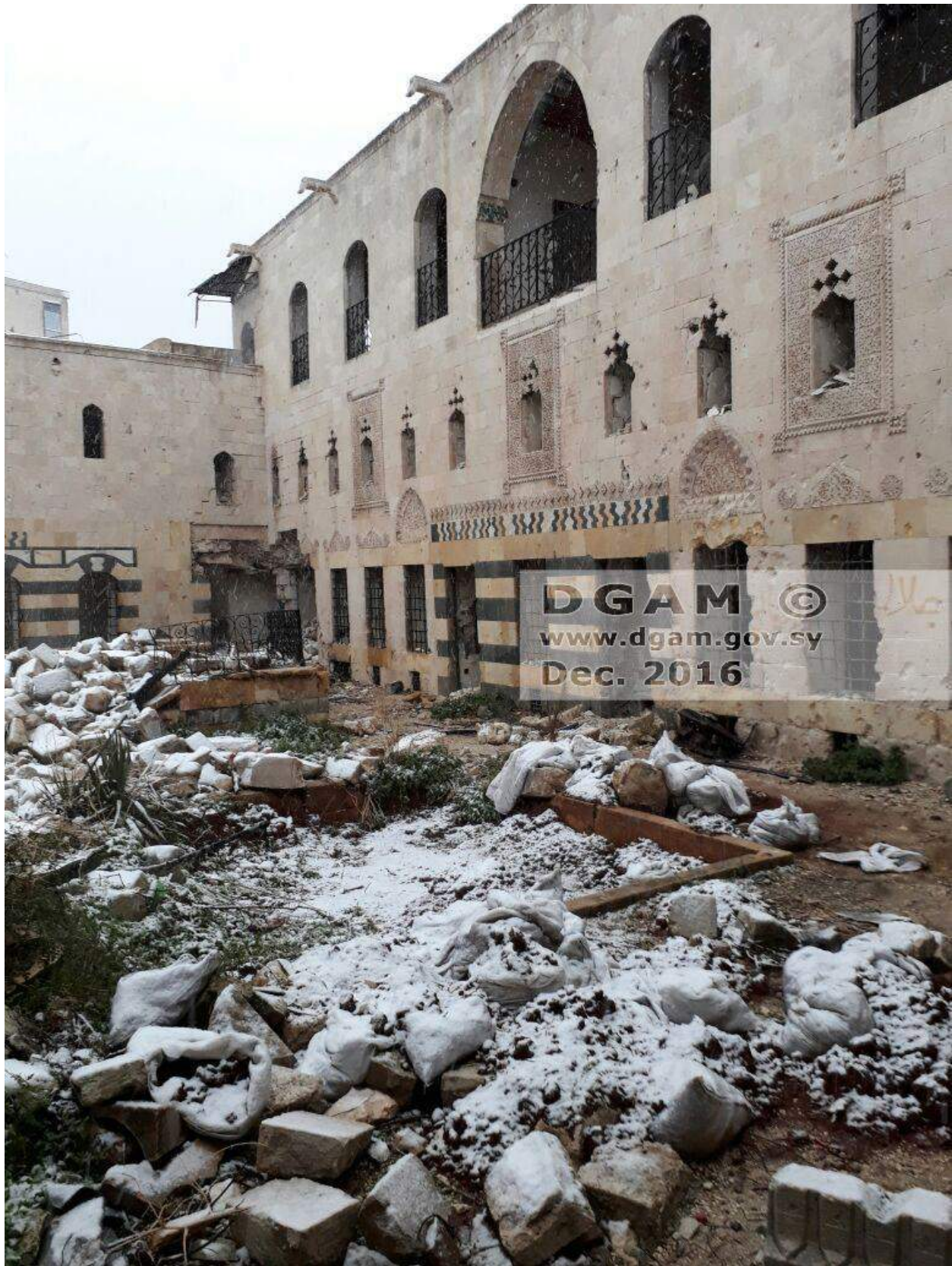
Severe damage to Beit Ghazaleh (DGAM; December 22, 2016)
