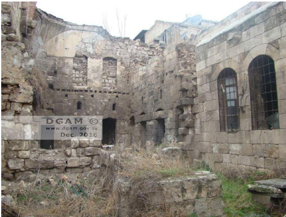
Damage and overgrowth of vegetation at Bimaristan Arghun al-Kamili (DGAM; December 31, 2016)
