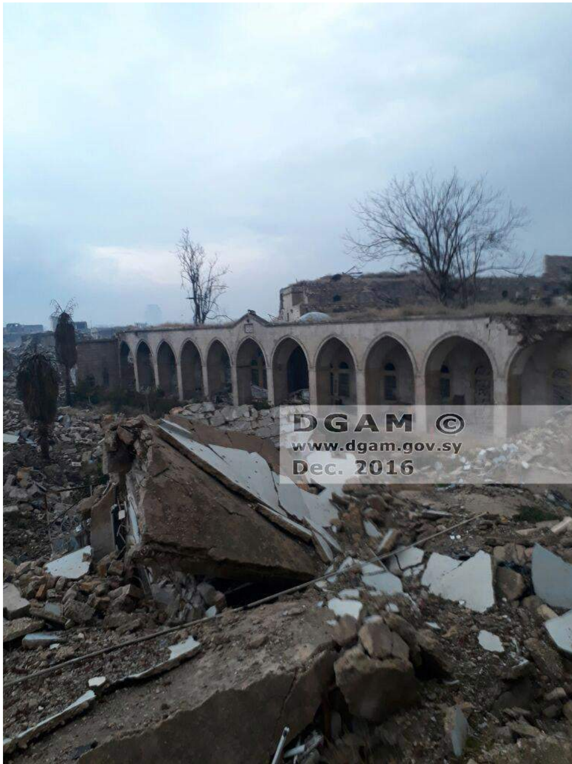
Extensive damage to Madrasa Khusruwiye (DGAM; December 28, 2016)
