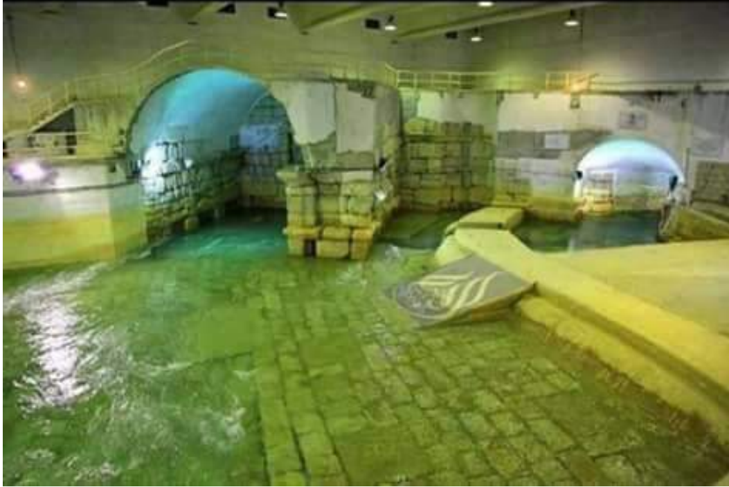
Damage to Ain al-Fijah Spring (Discover Syria; December 27, 2016)
