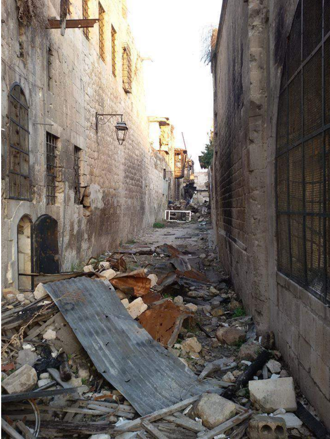
Damage seen outside Takkiya Nasimi (Private Facebook Account; December 19, 2016)
