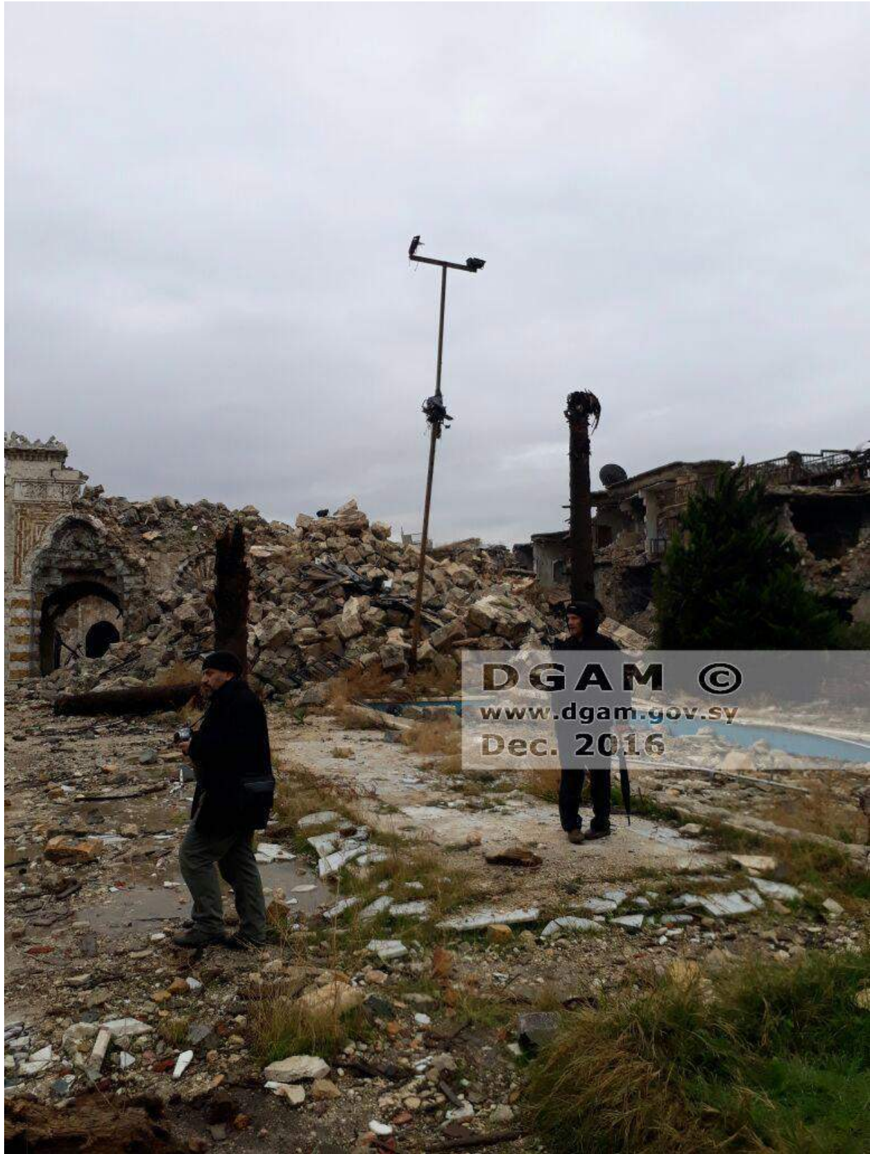
Rubble from the collapsed minaret of the Umayyad Mosque (DGAM; December 16, 2016)
