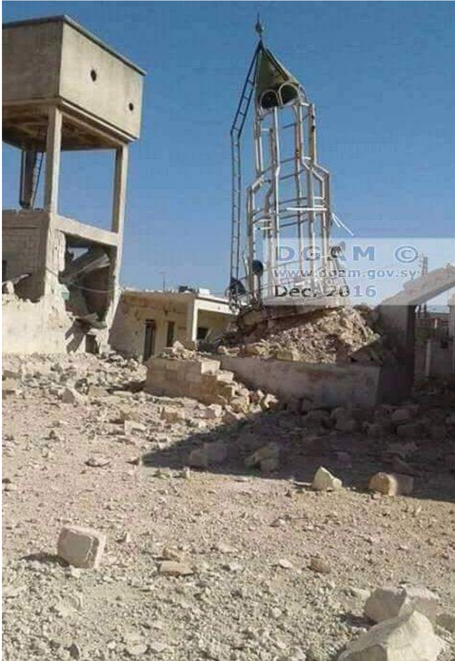
Damage to al-Hazazeh Minaret (DGAM; December 20, 2016)
