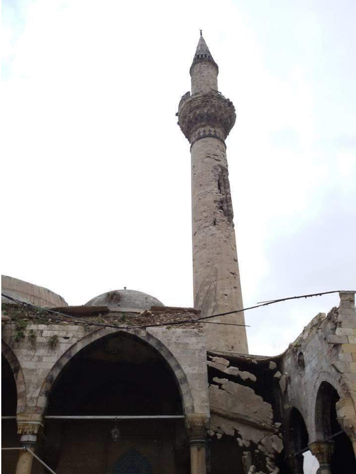
Structural damage seen to Adliyah Mosque (Private Facebook Account; December 17, 2016)
