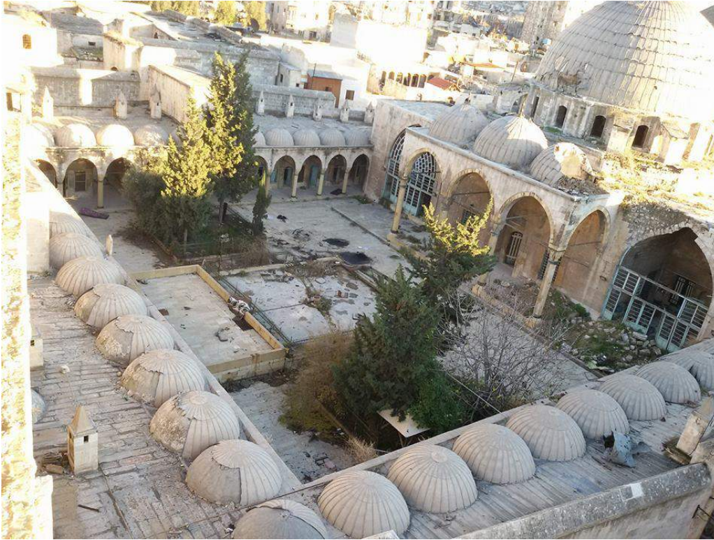
An overview of the damage to al-Uthmaniya Mosque (Private Facebook Account; December 15, 2016)
