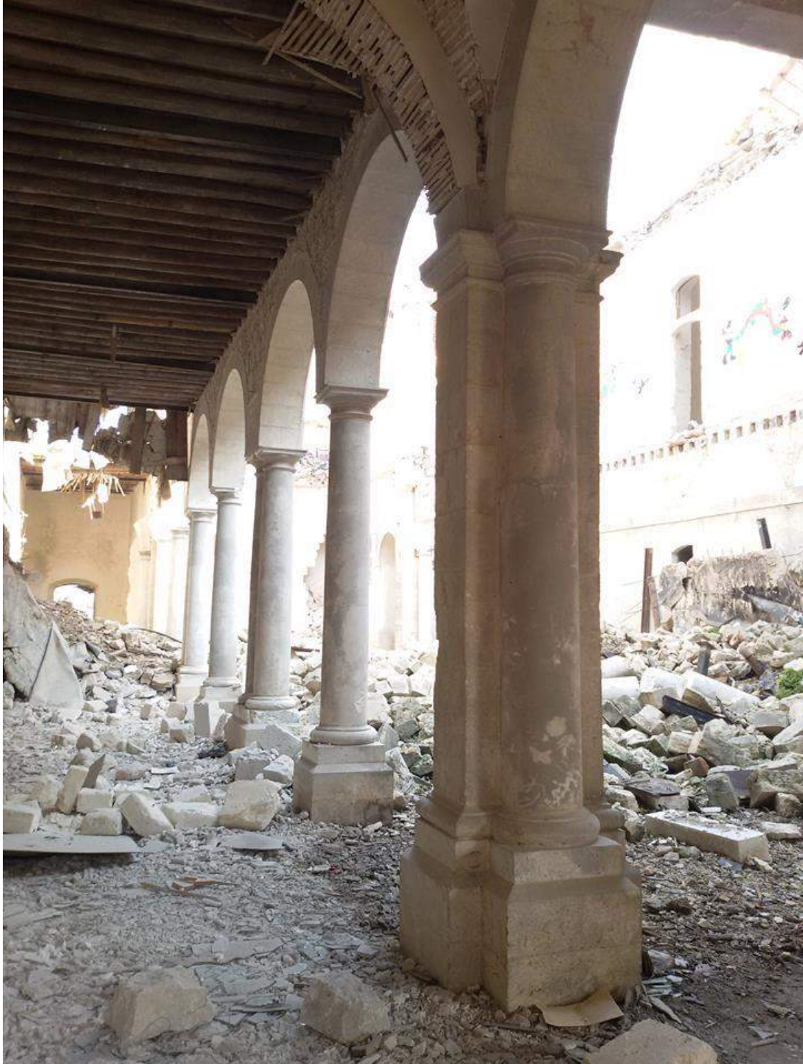
Severe damage to the interior and courtyard of the Yassou'iyah (Private Facebook Account; December 19, 2016)
