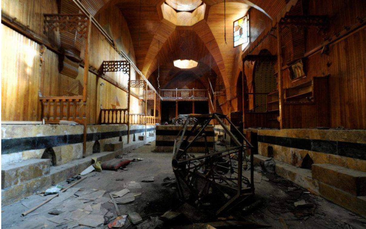
Damage to the interior of Hammam al-Nahasin (Reuters; December 21, 2016)
