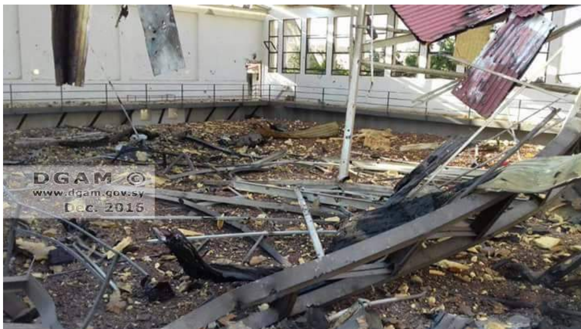
Extensive damage to Tayyibet al-Imam Museum (DGAM; December 20, 2016)
