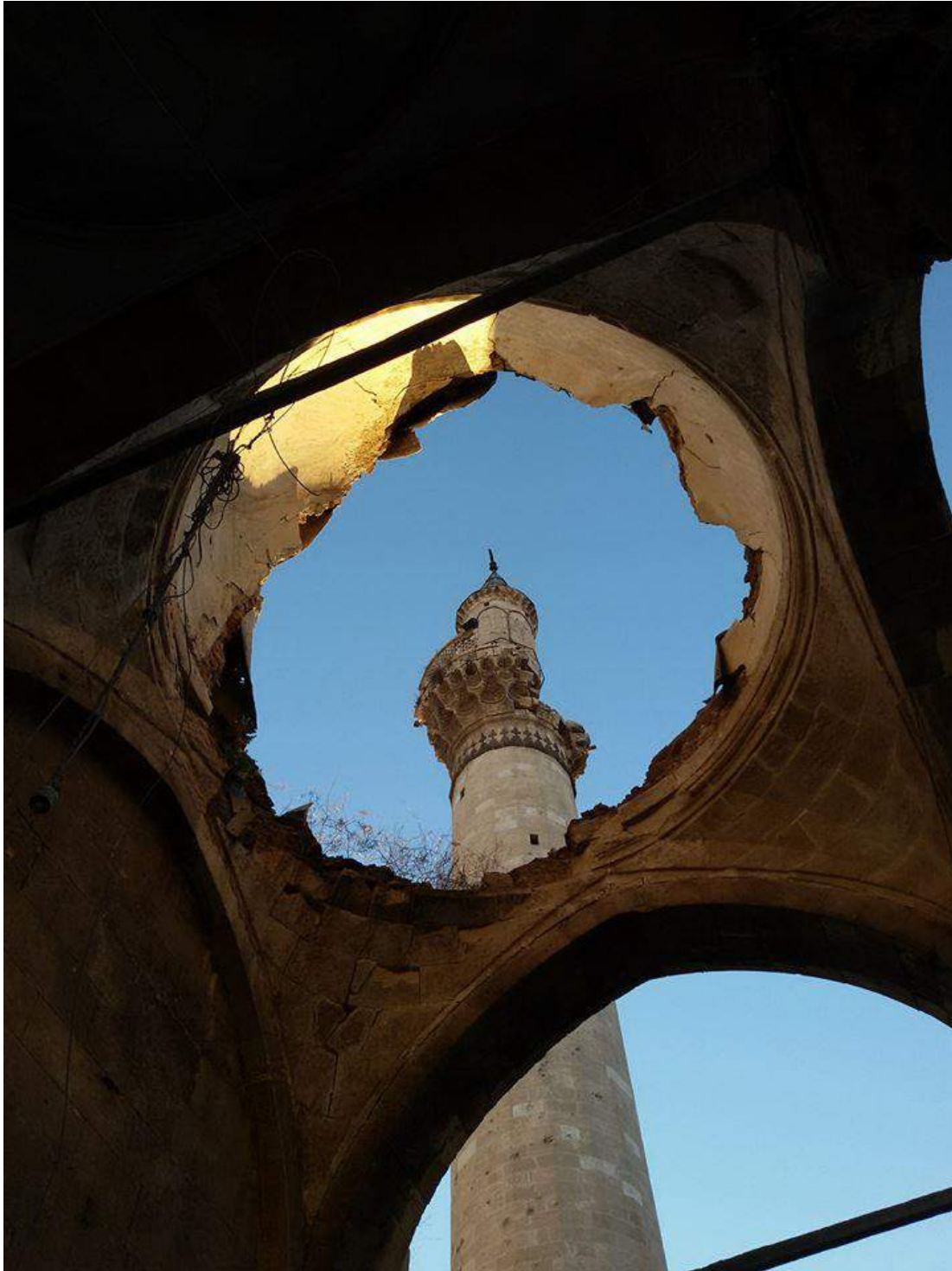
What appears to be a missing dome inside al-Uthmaniya Mosque (Private Facebook Account; December 15, 2016)
