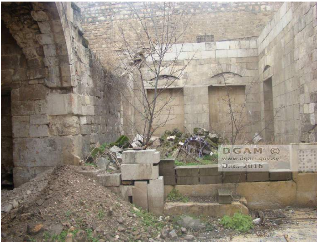
Moderate damage and debris present at Bimaristan Nur al-Din (DGAM; December 31, 2016)
