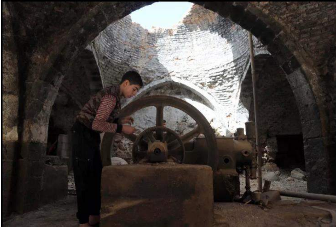
Extensive damage seen at Harasta Olive Oil Mill (Bisan Ilan Kurumu; November 22; 2016)
