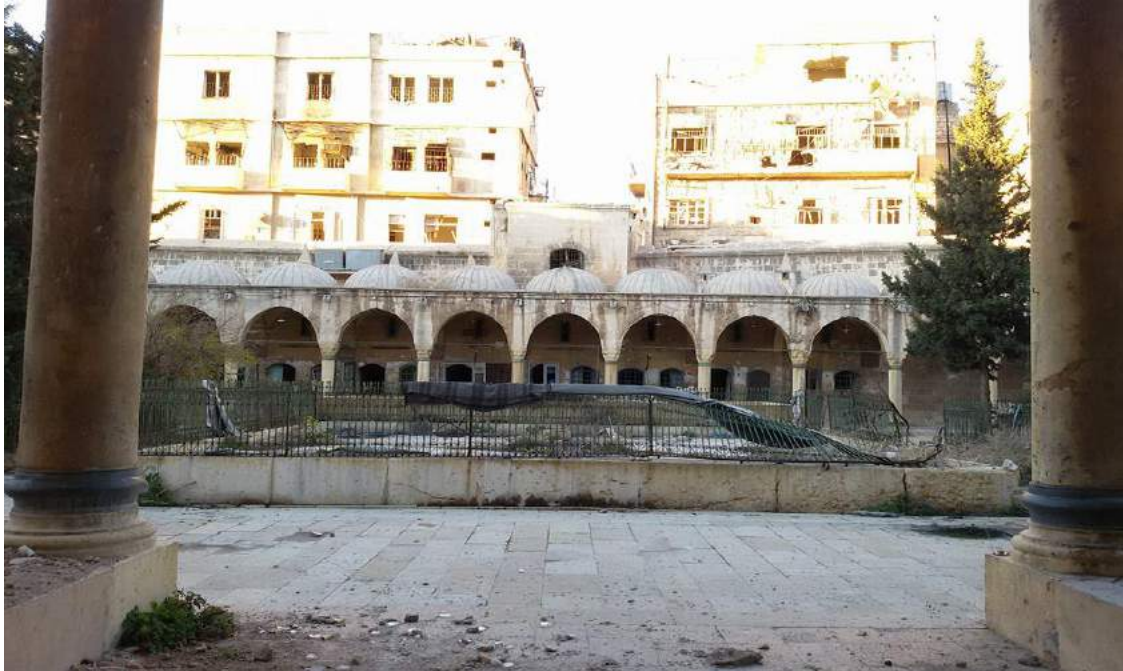
The condition of al-Uthmaniya Mosque (Private Facebook Account; December 15, 2016)
