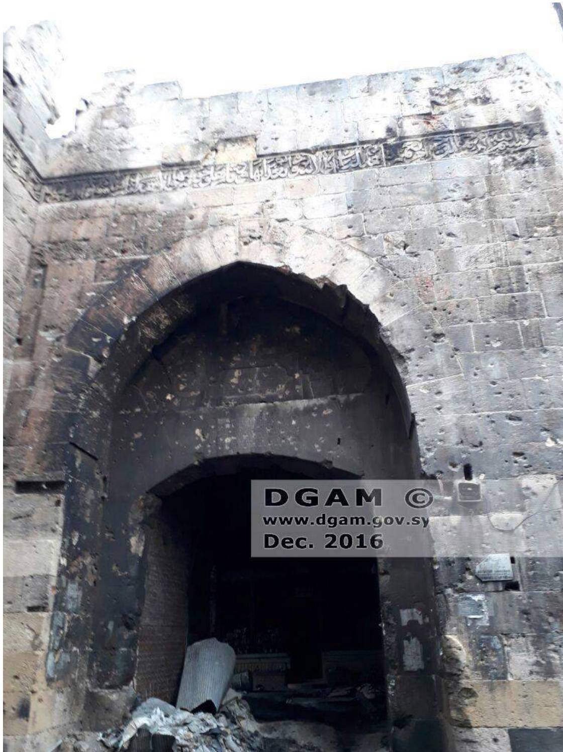
Smoke damage and shrapnel or gunfire damage to the Bab Antakya (DGAM; December 24, 2016)
